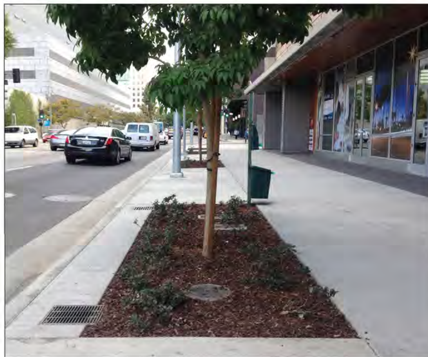
Tree well with planting and mulch along with concrete convenience strip
