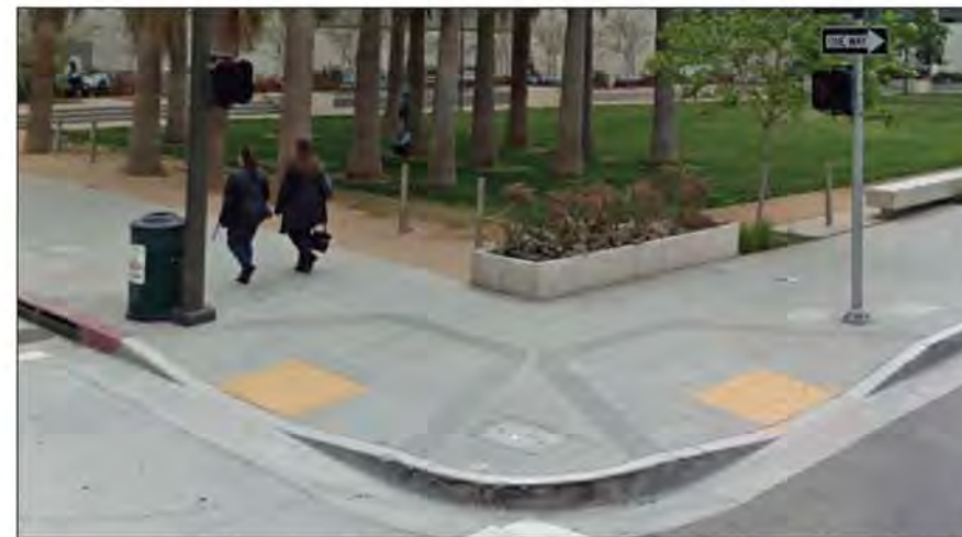
Dual curb ramps with detectable warning surfaces
