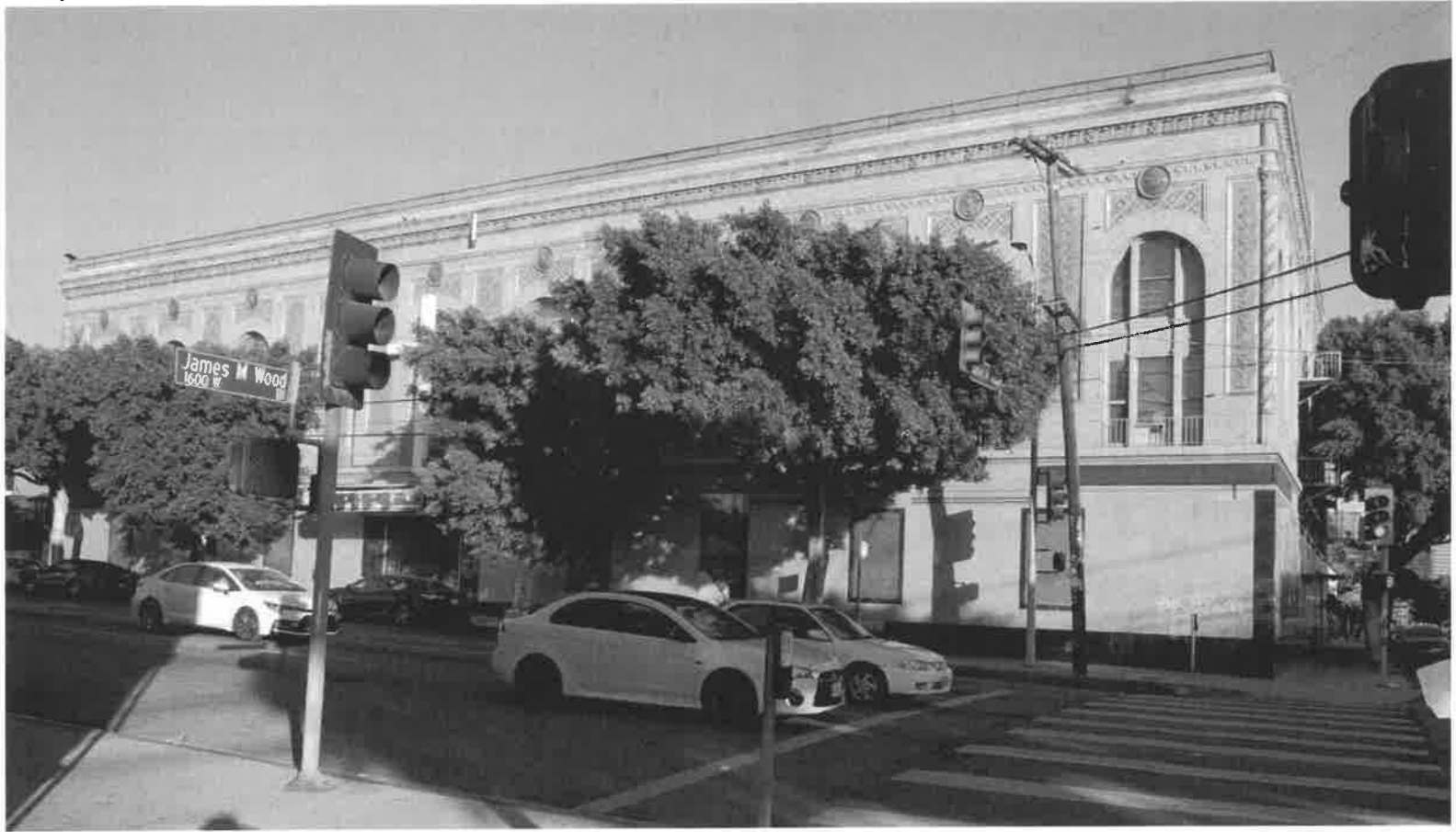
West façade, 846 S. Union Ave. View east. (2022 Luftman)
