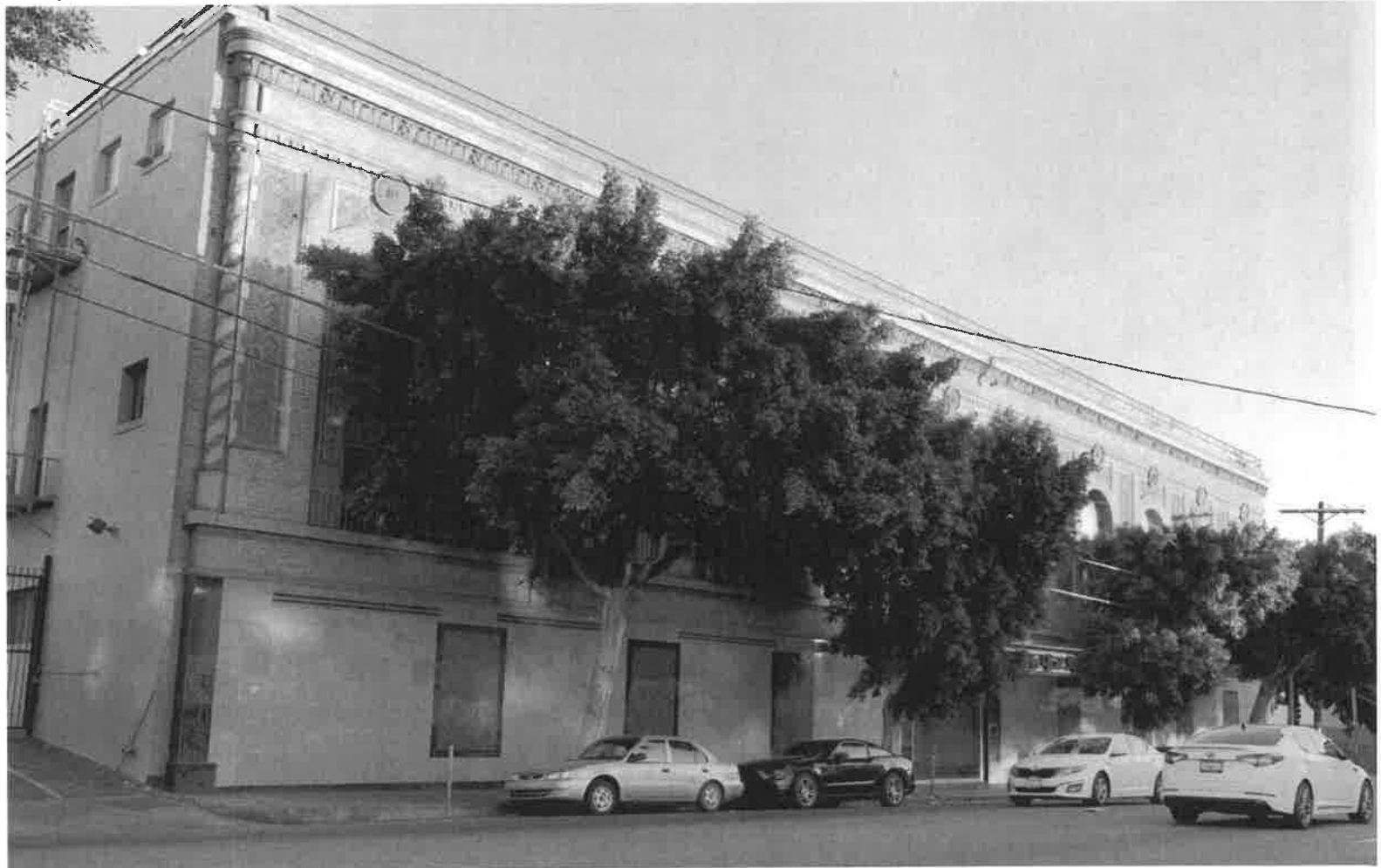
West façade, 846 S. Union Ave. View southeast. (2022 Luftman)
