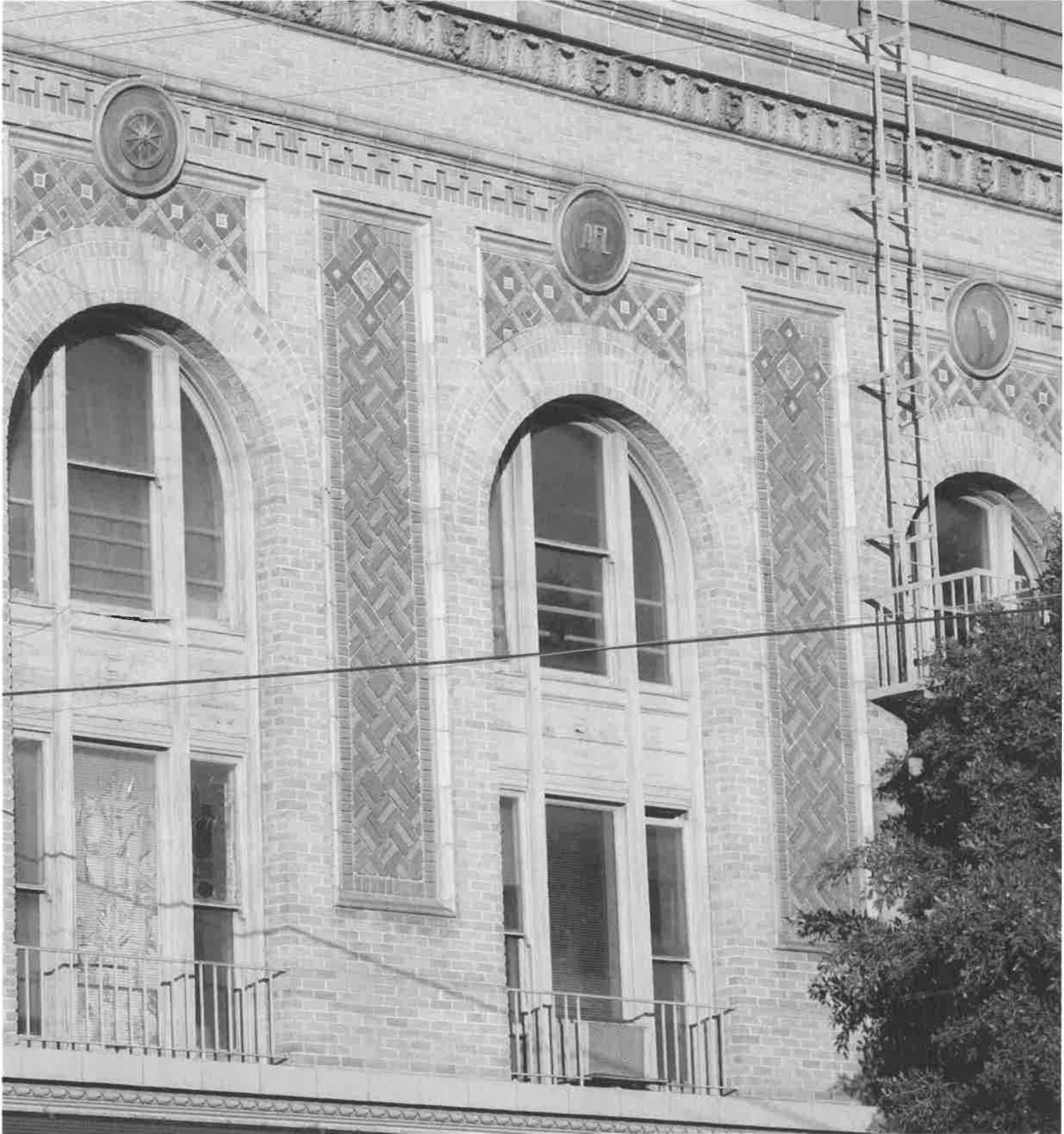
South façade, 846 S. Union Ave. View northeast. Above each arch is a cartouche of three different designs, the wagon wheel Teamsters emblem, AFL initials, and a waving American flag. (2022 Luftman)
