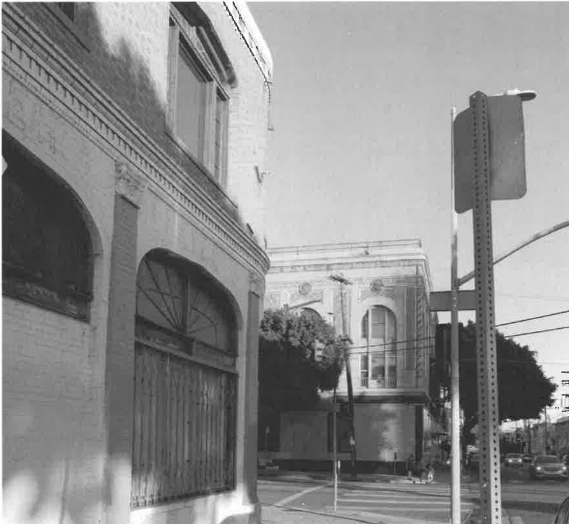
West façade, 846 S. Union Ave. View east. (2022 Luftman)
