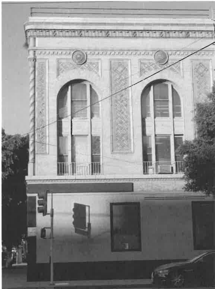
South façade, 846 S. Union Ave. View north. (2022 Luftman)
