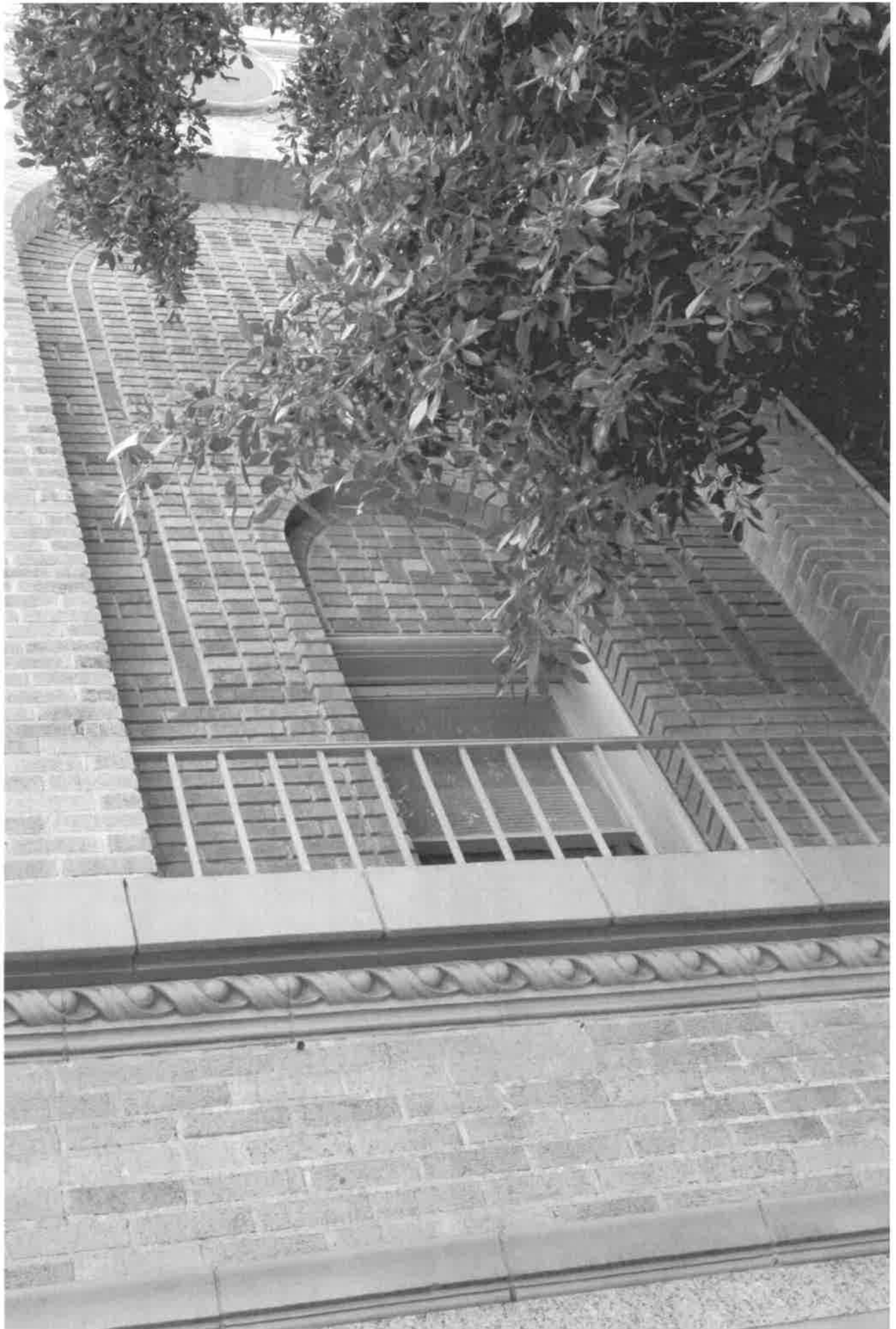
On the west façade of the subject building, the northernmost arch is bina with elaborate brick mull, and a smaller bina-arch with a simple wood-framed double-hung one-over-one window centered at the base of the second floor. View east. (2022 Luftman)
