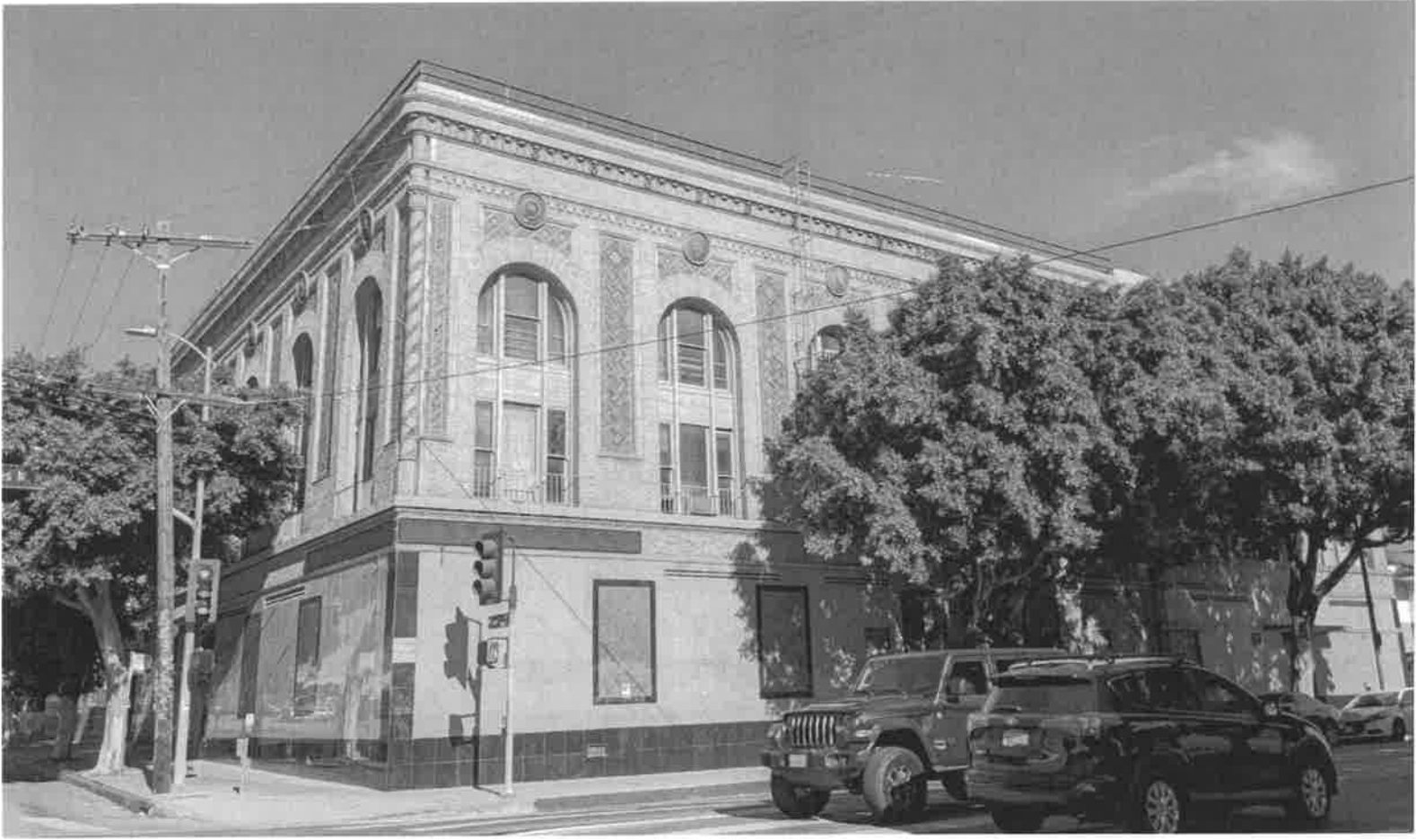
outh façade, 846 S. Union Ave. View north. (2022 Luftman)
