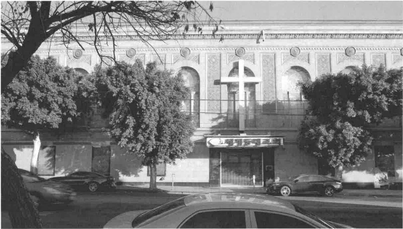
Primary entrance, west façade, 846 S. Union Ave. View east. (2022 Luftman)
