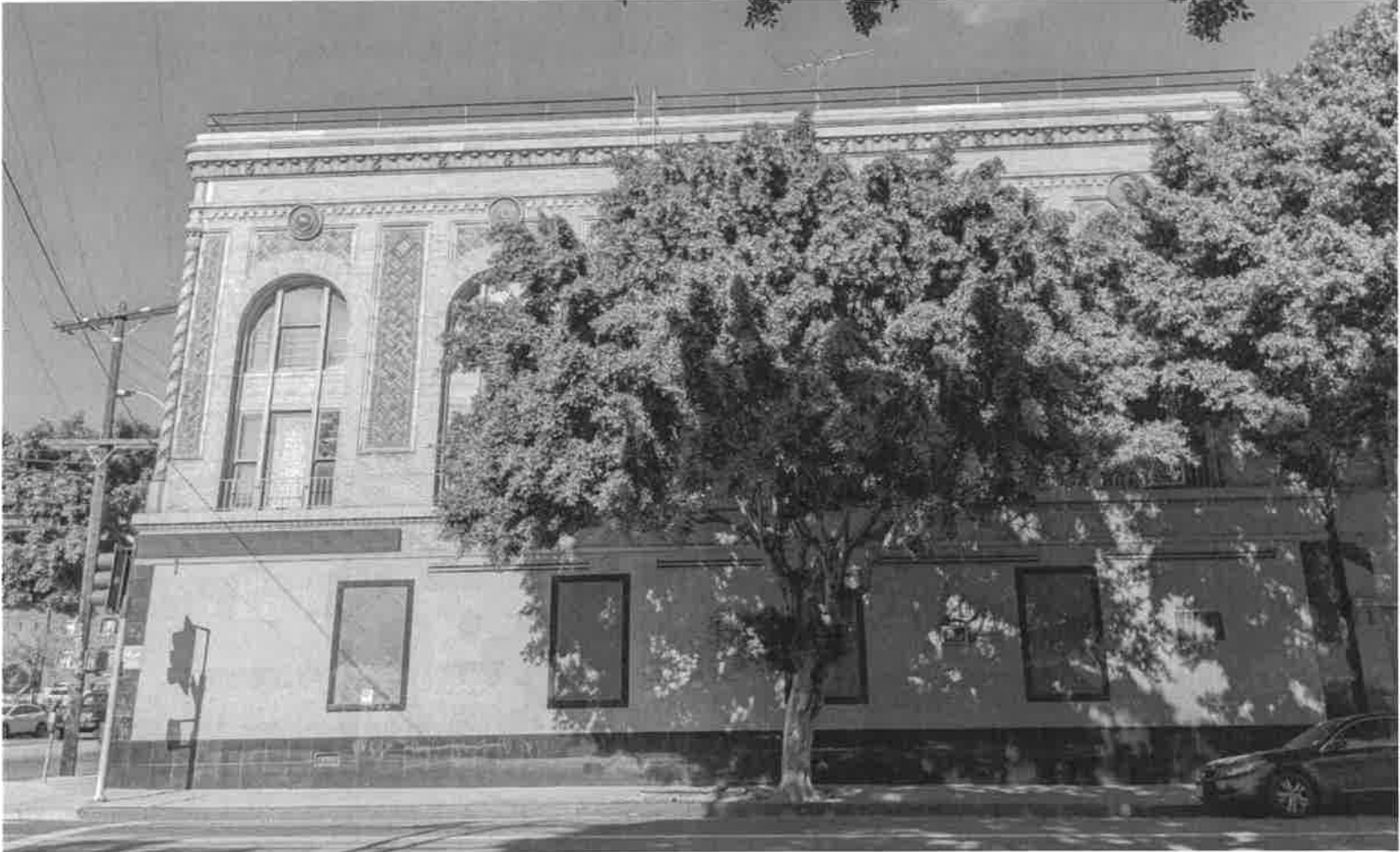
outh façade, 846 S. Union Ave. View north. (2022 Cooper)
