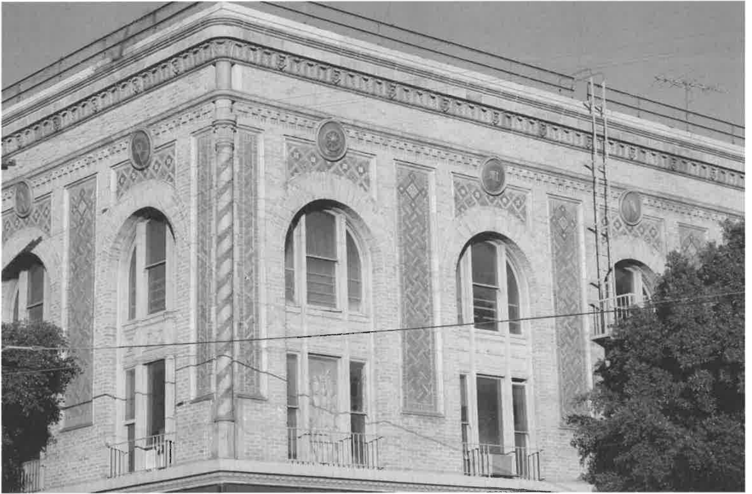
West and south façades, 846 S. Union Ave. View northeast. (2022 Luftman)
