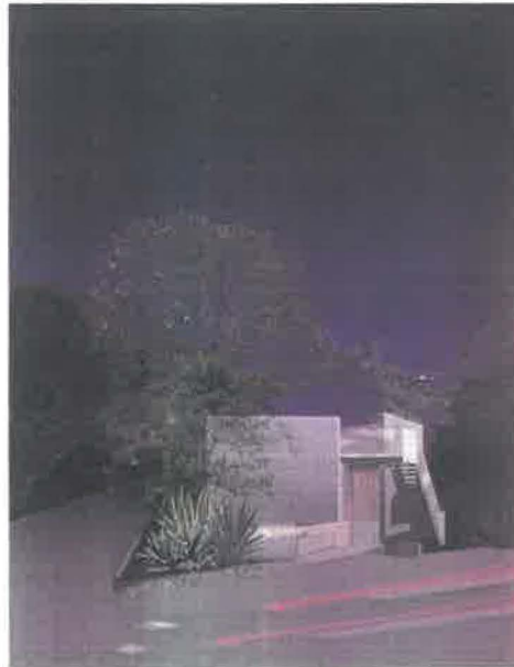
B1 - WEST ELEVATION WITH FRONT ENTRY LOOKING EAST FROM CLIFF DR
