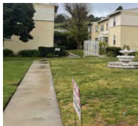
Existing concrete paving, to be rehabilitated
