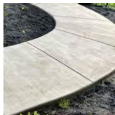
New concrete walkways
