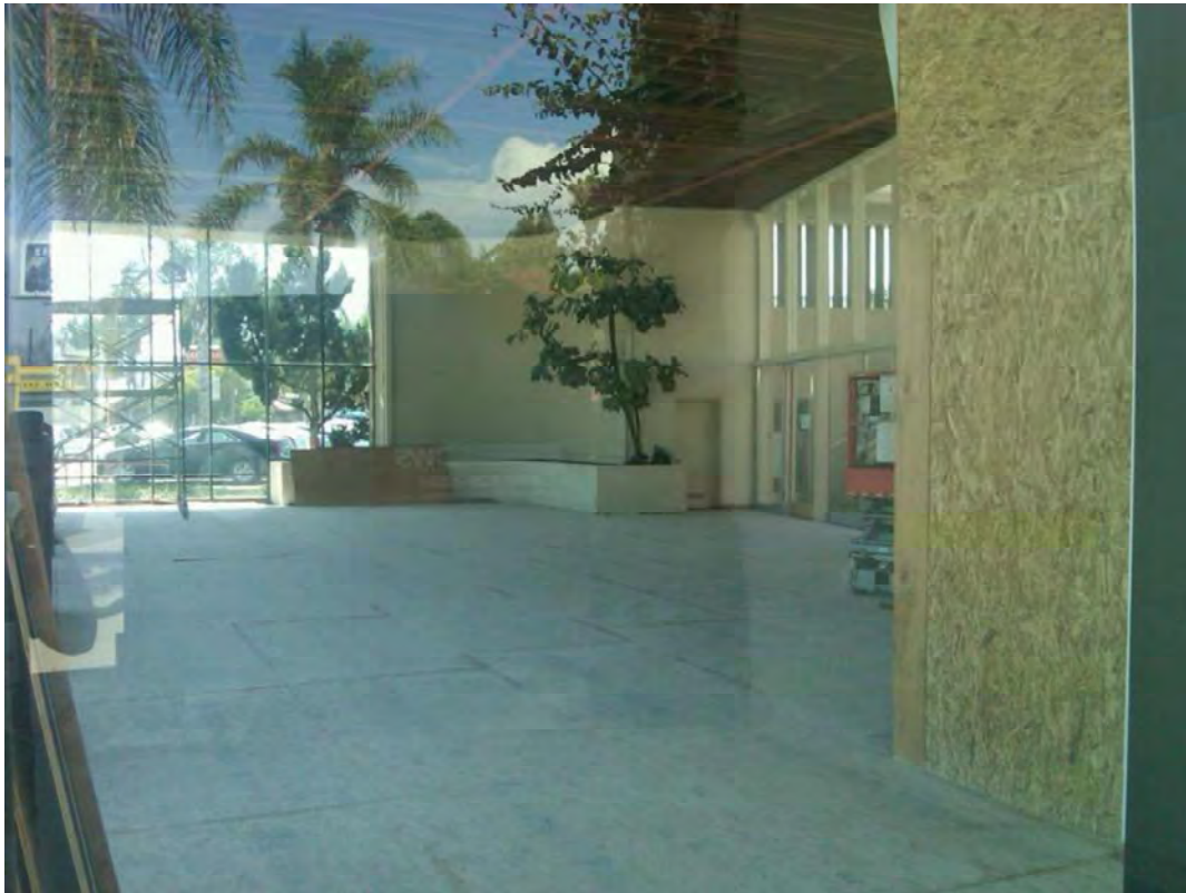
Casa de Cadillac, terrazzo floor protected during work, 14401 Ventura Blvd, September 28, 2012 (Photograph by Steve Vilerino)
