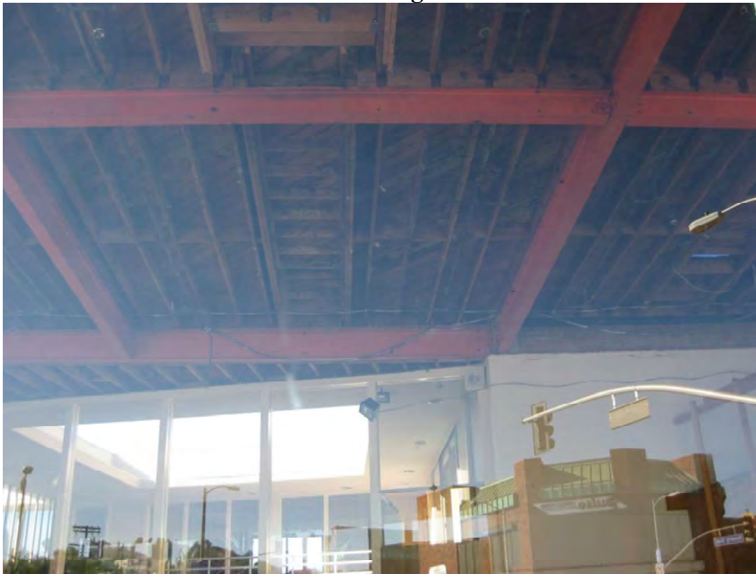
Casa de Cadillac, ceiling removed from showroom, 14401 Ventura Boulevard, September 28, 2012 (Photograph by Steve Vilerino)
