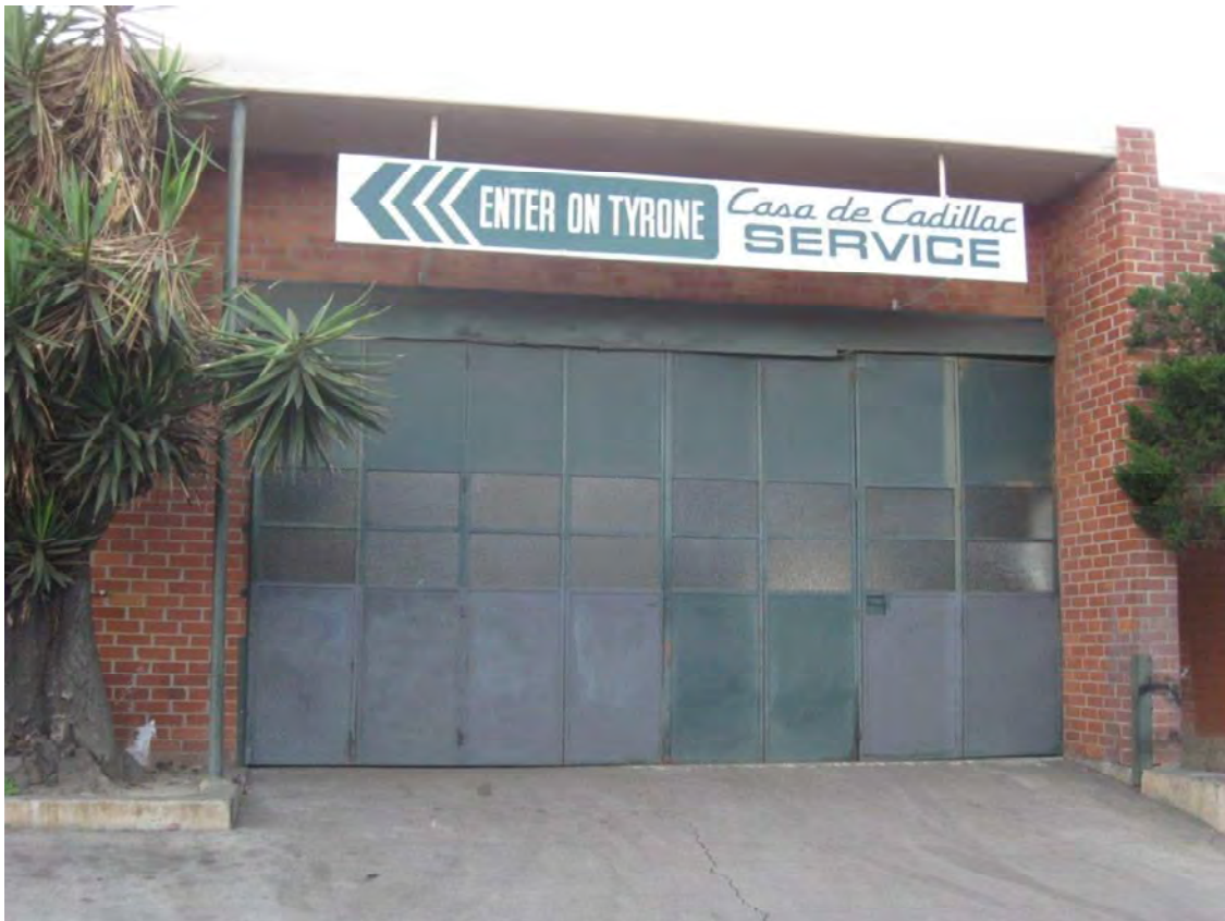
Casa de Cadillac, service entrance, 14401 Ventura Boulevard, November 26, 2009 (Photograph by Chris Green)
