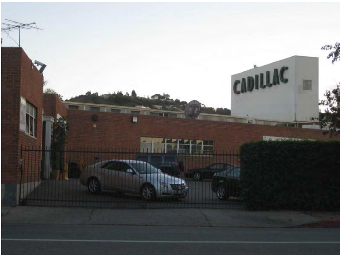
Casa de Cadillac, rear of service wing, 14401 Ventura Boulevard, November 26, 2009 (Photograph by Chris Green)
