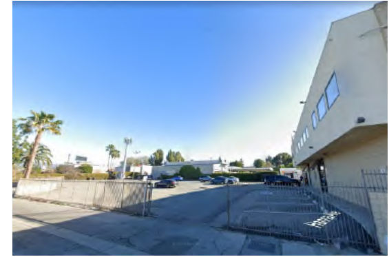
EXISTING WEST CORNER LOOKING NORTH-EAST
