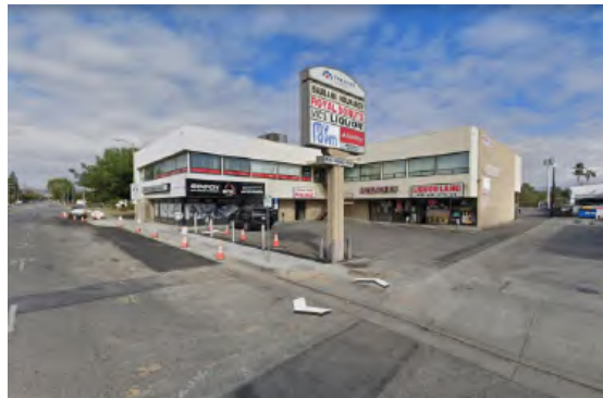
EXISTING SOUTH-EAST CORNER LOOKING NORTH
