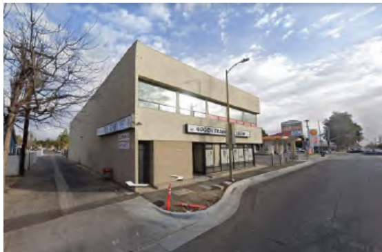
EXISTING SOUTH-WEST CORNER LOOKING NORTH
