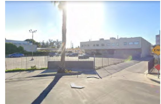
EXISTING NORTH-WEST CORNER LOOKING SOUTH
