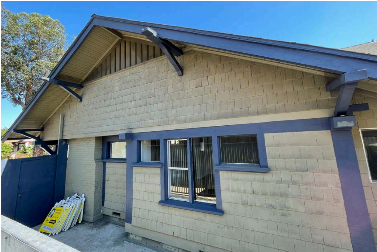
North elevation of subject residence, showing chimney serving the living room fireplace, and the dining room “false bay” window. Also note the knee braces with integral feet supporting the gable, another “Webster-ism.” Photo taken by nomination preparers.
