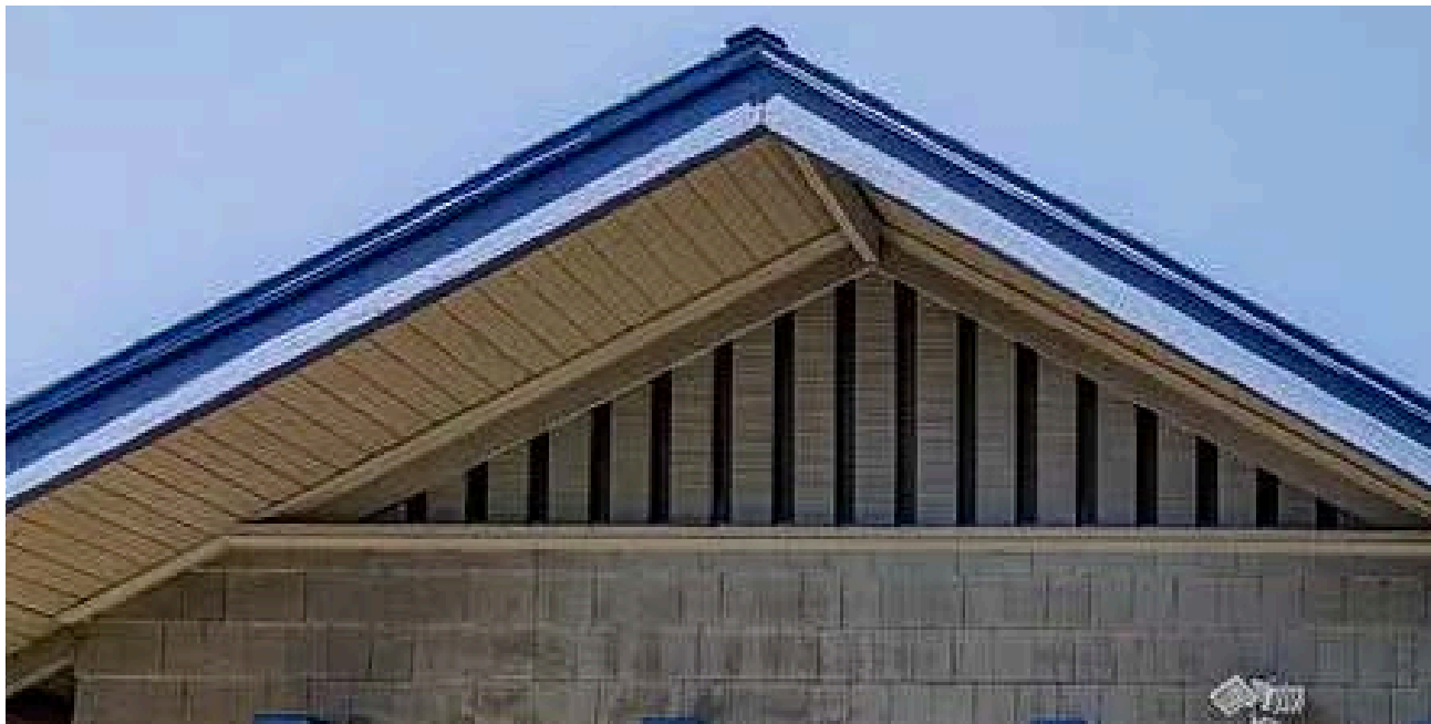
Left: East facing gable (front facade) with infill featuring board-on-board gable vents in signature Webster style (Source: MLS Photo, 2022) Right: North facing gable with vents (Source: nomination preparer) Below: Diagram by John Ripley showing Webster’s board-on-board gable vents.
