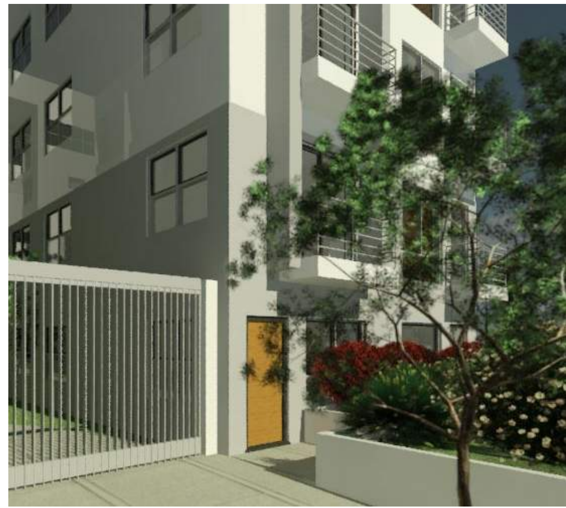
UNIT 121 WITH ENTRY DOOR FACING FRONT AVE.
