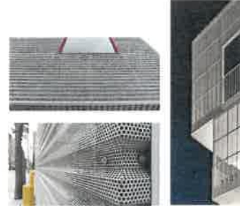
EXIT BALCONIES METAL PANEL METAL SALES MANUFACTURING CORPORATION T16-E-WALL PANEL PERFORATED VERTICAL & HORIZONTAL INSTALLATION PANEL COVERAGE: 36" RIB HEIGHT: 3/4" COVERAGE: 36"
