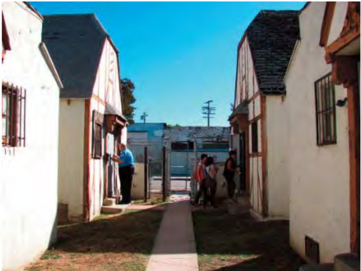
Central courtyard, facing east. Source: Holmes + Zepeda, 2012.
