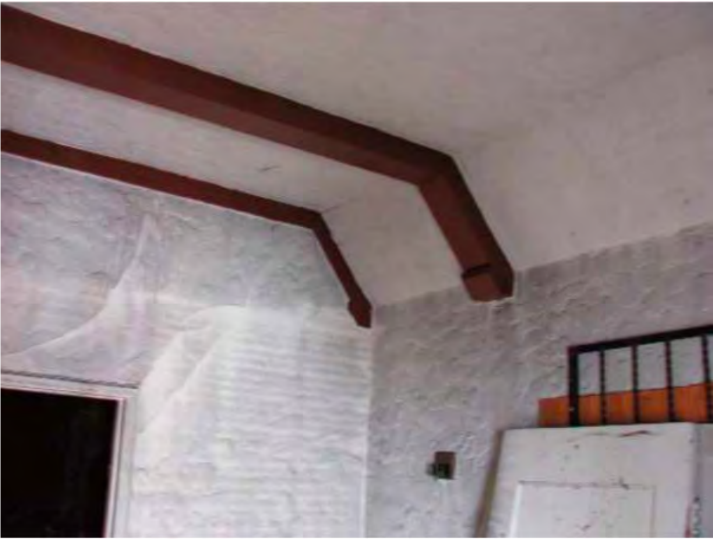
Interior ceiling. Source: Holmes + Zepeda, 2012.
