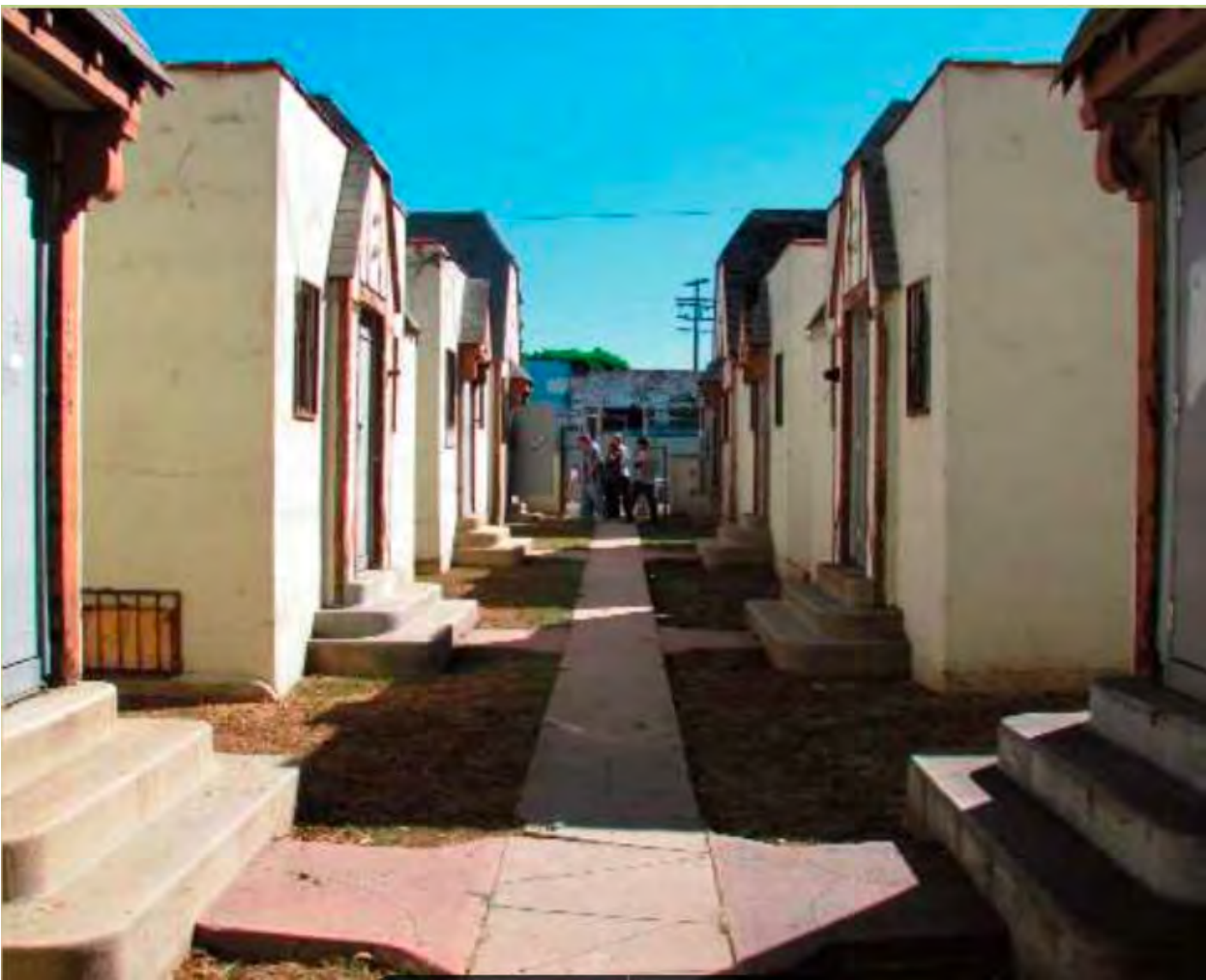
Central courtyard, facing east. Source: Holmes + Zepeda, 2012.
