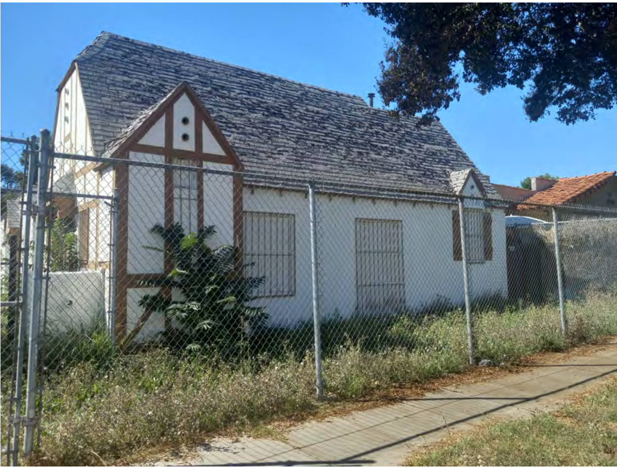
Front facade of northeastern unit, facing northwest. Source: Raymond Gutierrez, 2023.
