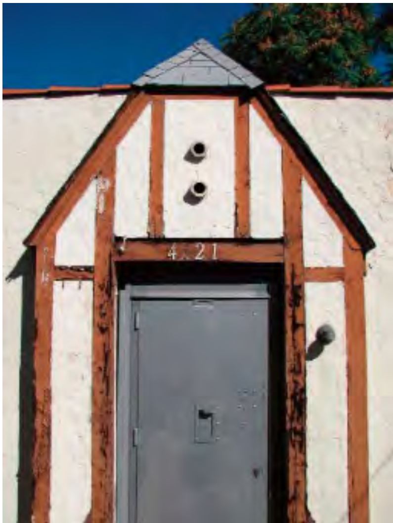
Detail, entrance of 4221 N. Maycrest Avenue. Source: Holmes + Zepeda, 2012.
