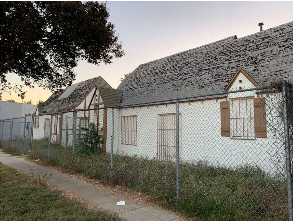
Front facade, facing southwest. Source: Lindsay Mulcahy/ L.A. Conservancy, 2023.
