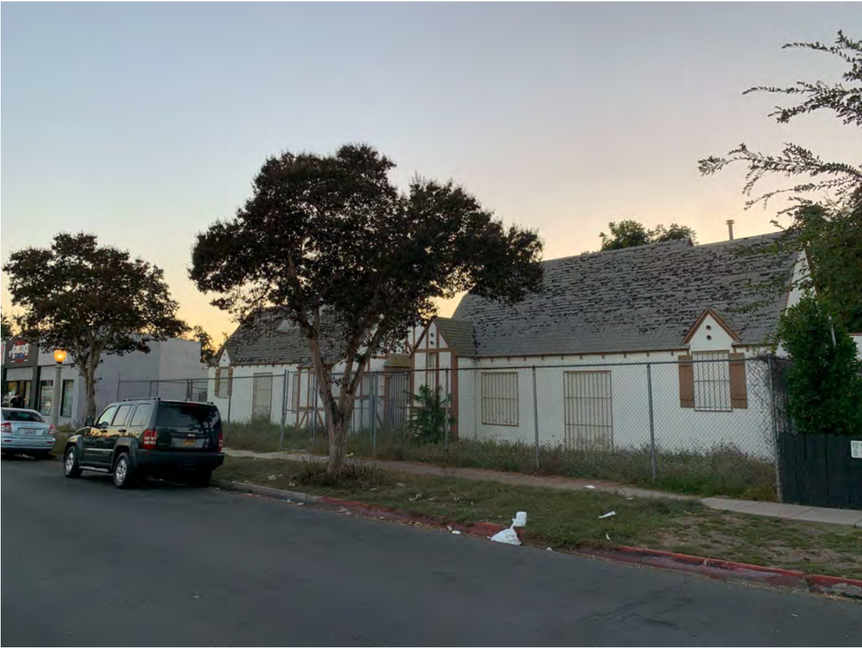
Streetview, facing southwest. Source: Lindsay Mulcahy/ L.A. Conservancy, 2023.
