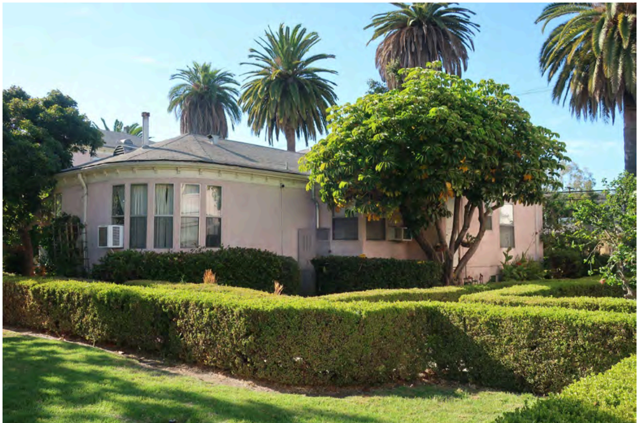
East Elevation of Building A
