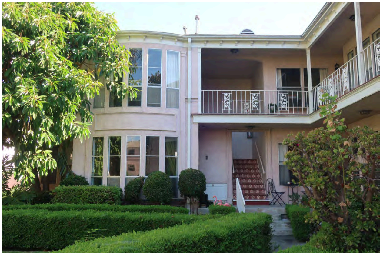
North Elevation of Building C (secondary)
