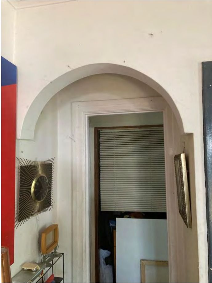
928 Marco Pl Original Interior Arch 4.29.24
