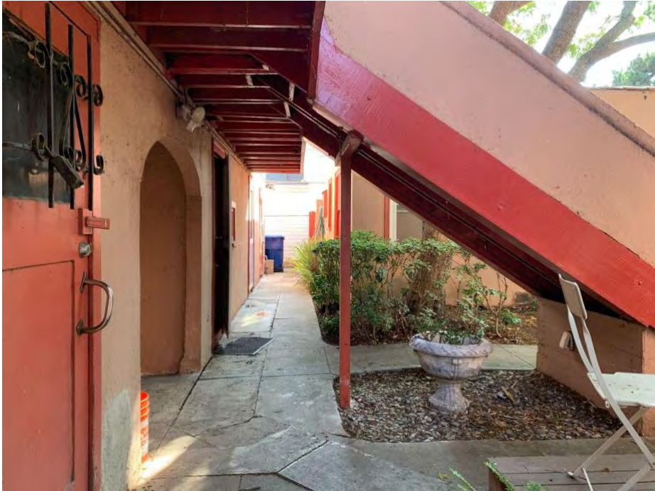
View facing southwest under stair 10.21.24
