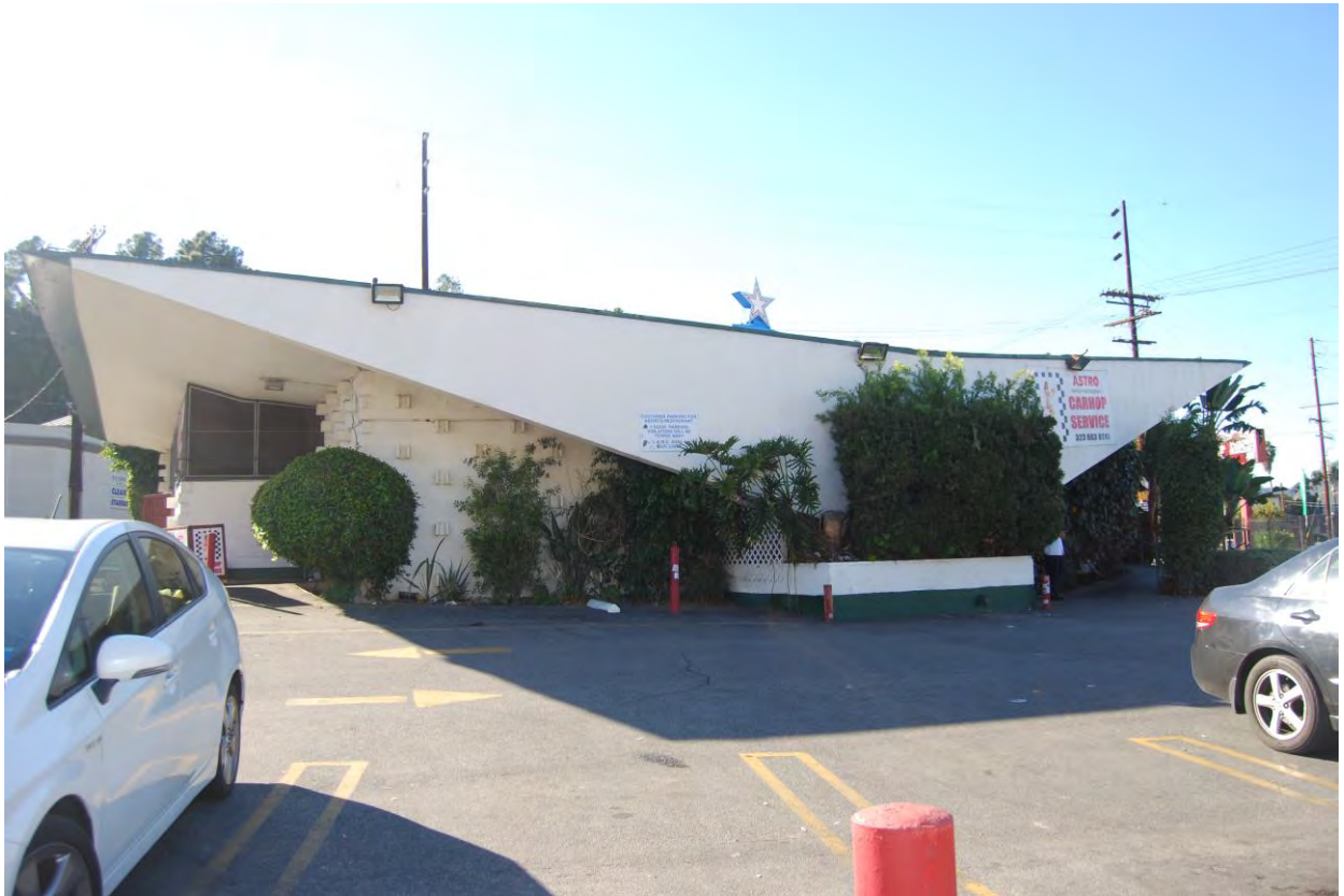
Astro Family Restaurant, Southeast facade, 2306 Fletcher Drive, November 22, 2022 (Photograph by Charles J. Fisher)
