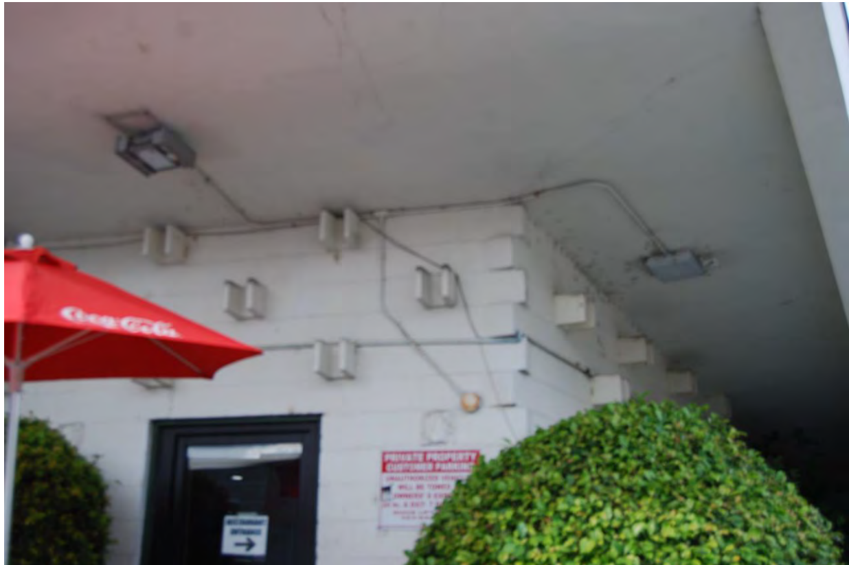
Astro Family Restaurant, decorative concrete at rear, 2306 Fletcher Drive, November 22, 2022 (Photograph by Charles J. Fisher)
