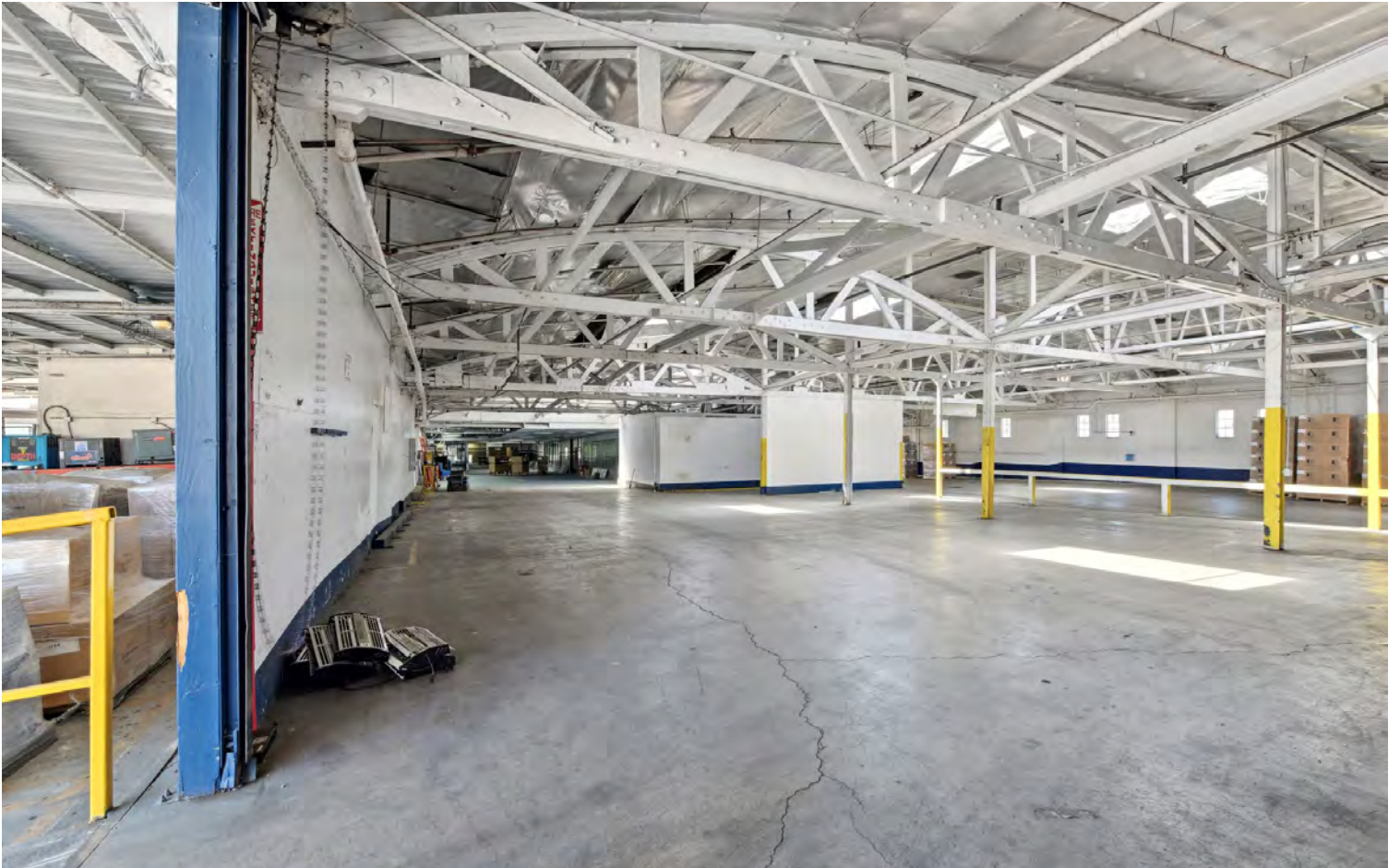
Sparkletts interior, original exposed wood beamed and trussed curved ceiling is extant. (LoopNet 2025)
