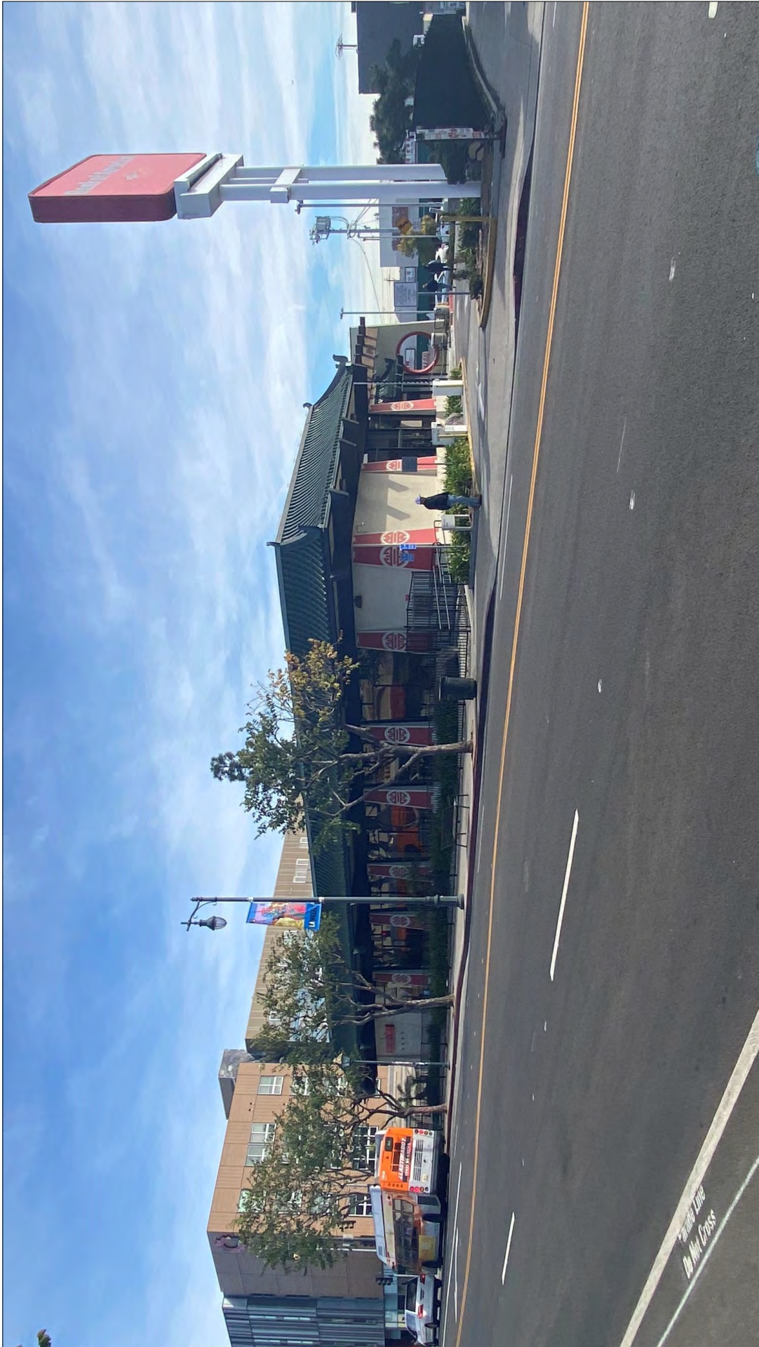
Figure 1: Bank of America, 850 North Broadway, west (left) and south (right) elevations, view northeast (Snow, 2020)
