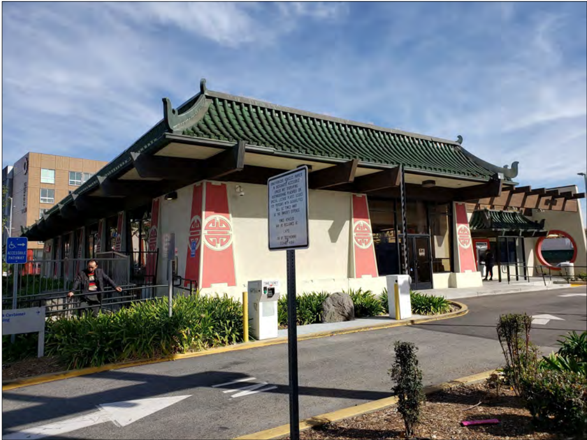
Figure 4: Bank of America, 850 North Broadway, west (left) and south (right) elevations, view northeast (Los Angeles Conservancy, 2020)
