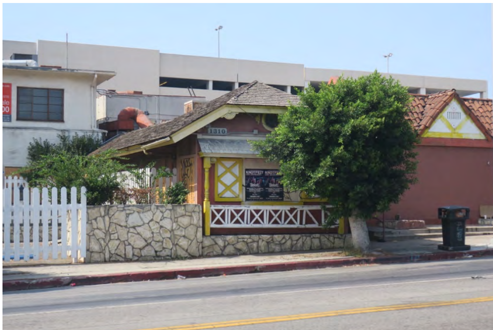
North façade of dining car, view southwest (ARG, 2021).
