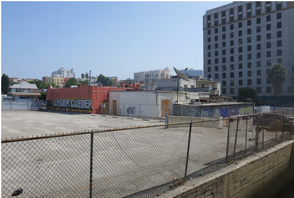
South and west façades from adjacent lot, view northeast (ARG, 2021).
