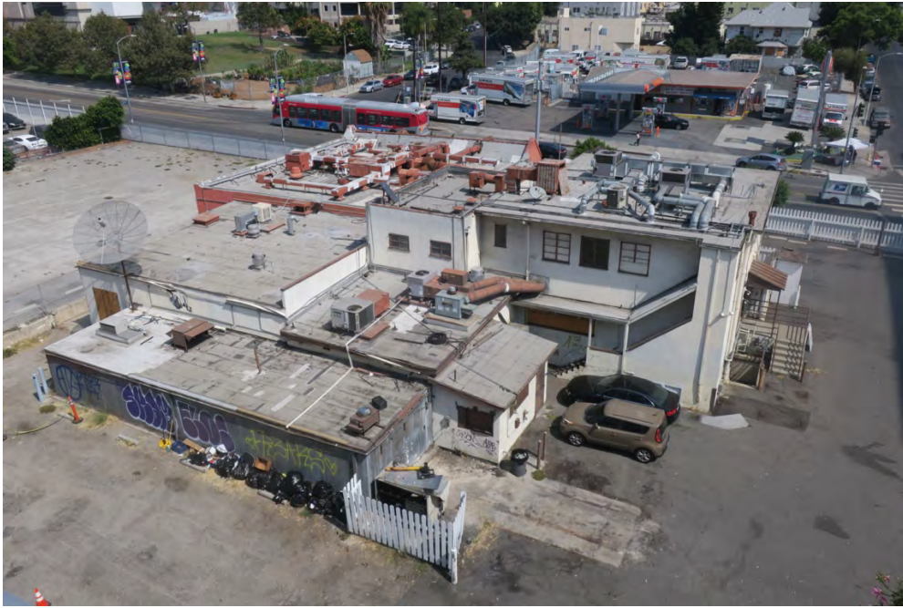
Property overview showing rear (south) and east façades, view northwest (ARG, 2021).
