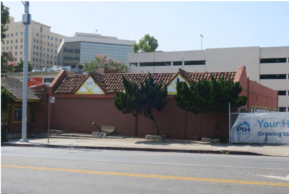
North façade of west dining room, view southeast (ARG, 2021).
