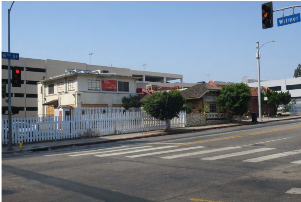
Property overview showing primary (north) façade, view southwest (ARG, 2021).
