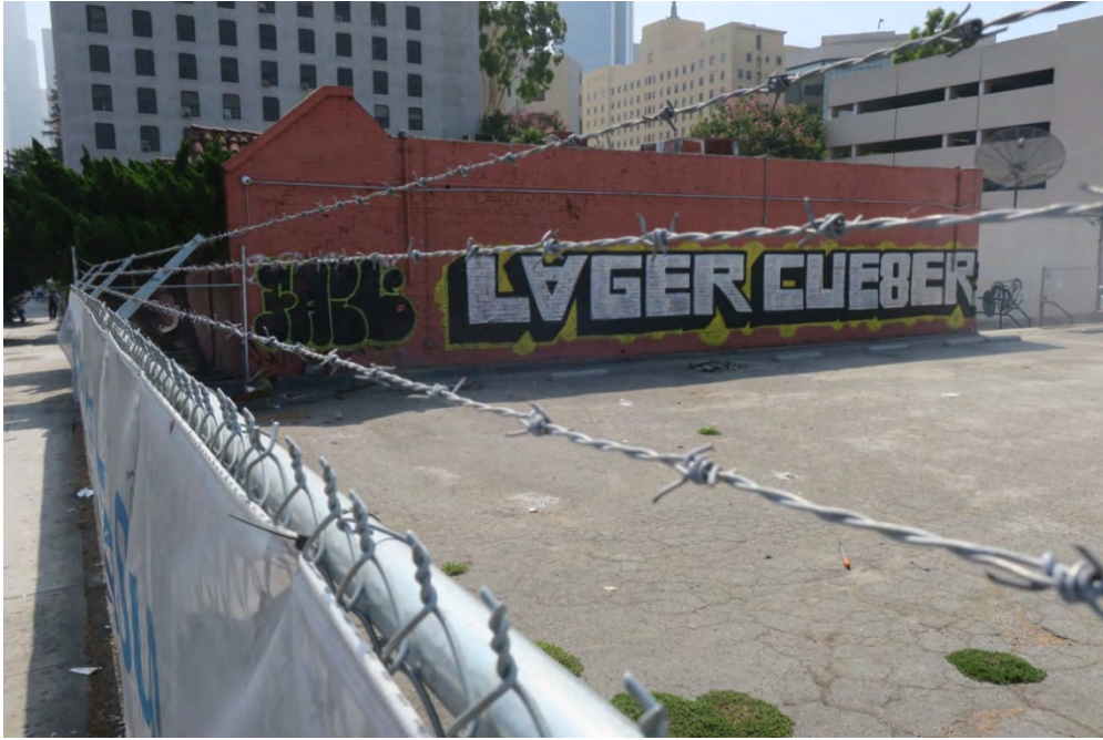
West façade of west dining room, view east (ARG, 2021).
