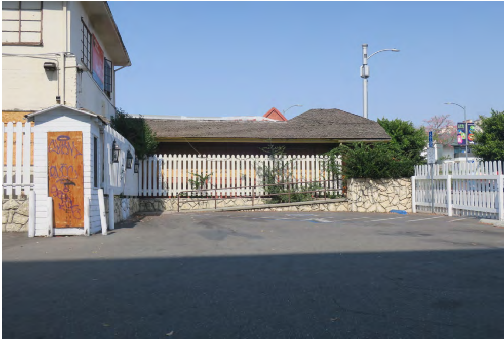
East façade of dining car, view west (ARG, 2021).
