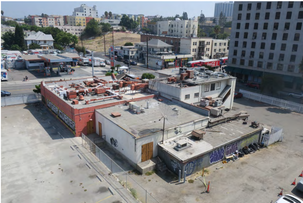
Property overview showing rear (south) and west façades, view northeast (ARG, 2021).
