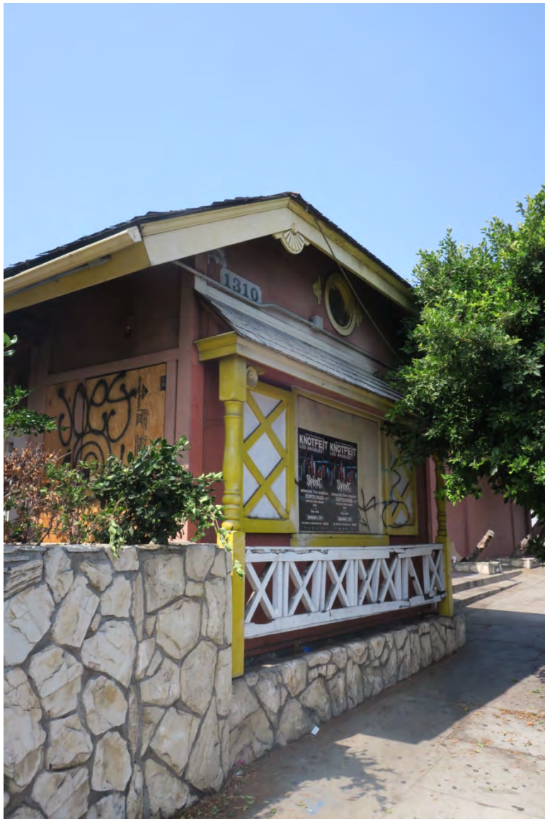
Detail: north façade of dining car, view southwest (ARG, 2021).
