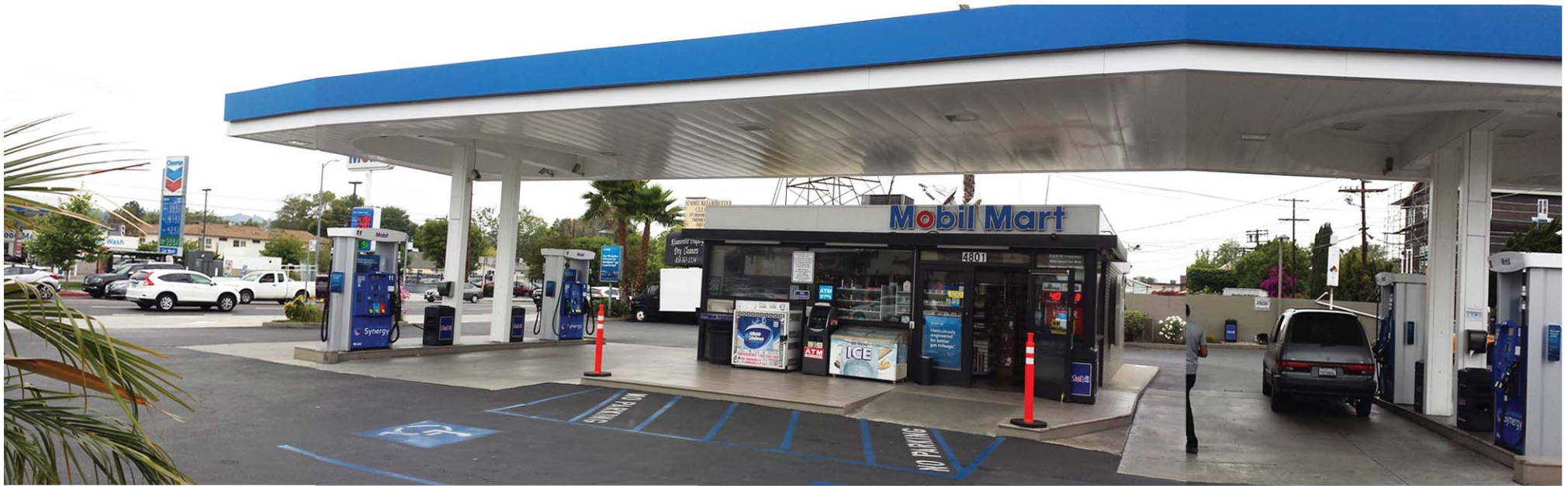
① Facing West - South at the east side of project property. East of property, East facade of existing fuel canopy with dispensers/ conc. curb and convenience store with curb (tile and conc. finish on top). And depicting existing handicap parking with conc. ramp.
