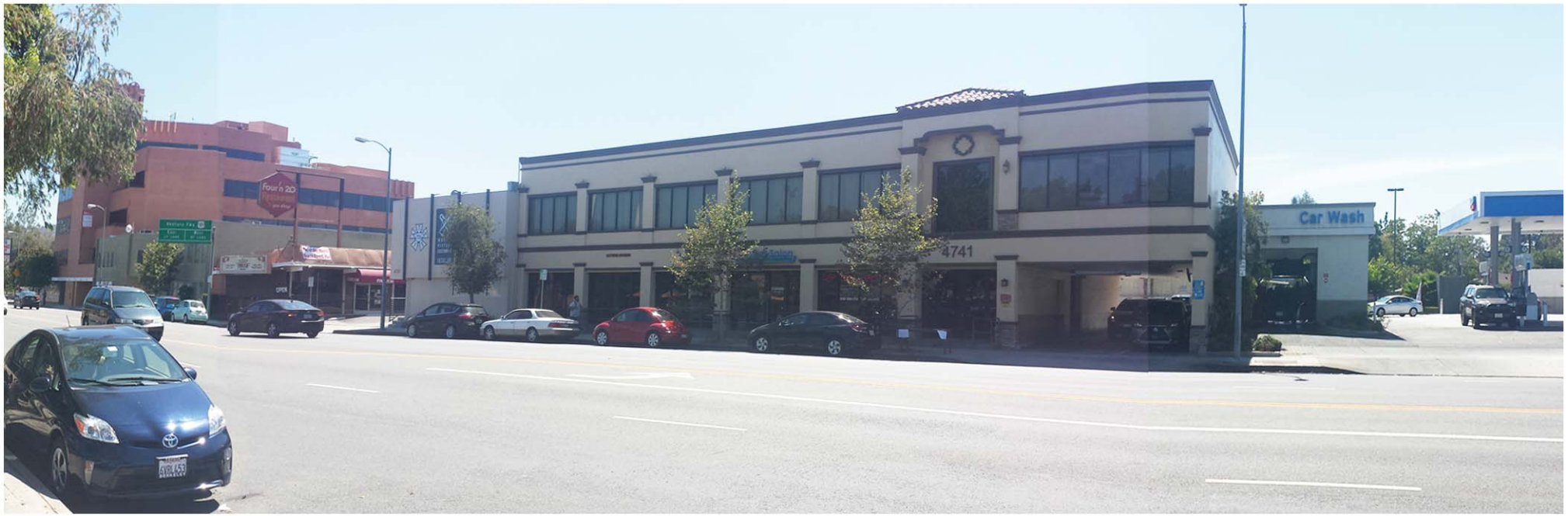
26 Facing Southwest (view down Laurel Canyon Blvd.), partial view of the existing Mobil Station and commercial buildings that are along Laurel canyon Blvd. with multi-residential and single residential are behind the commercial properties.
