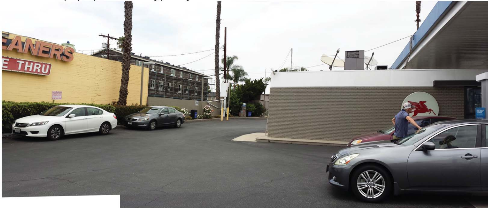
8 Facing North at the South of the project property. South of property, partial South facade of existing convenience store with curb. In addition, depicting existing landscape planter with conc. curb. along the West of property with 2 existing parking, and adjacent commercial (existing Cleaners) Building along the west of property, behind the building is commercial parking for the cleaners (the rest of the length along the west of the property).
