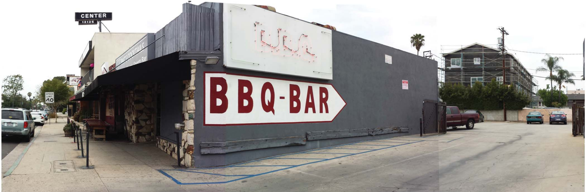
19 Facing West - North (view down Laurel Canyon Blvd. at West of the project property), commercial buildings are along Riverside Dr. and multi-residential and single residential are behind the commercial properties.
