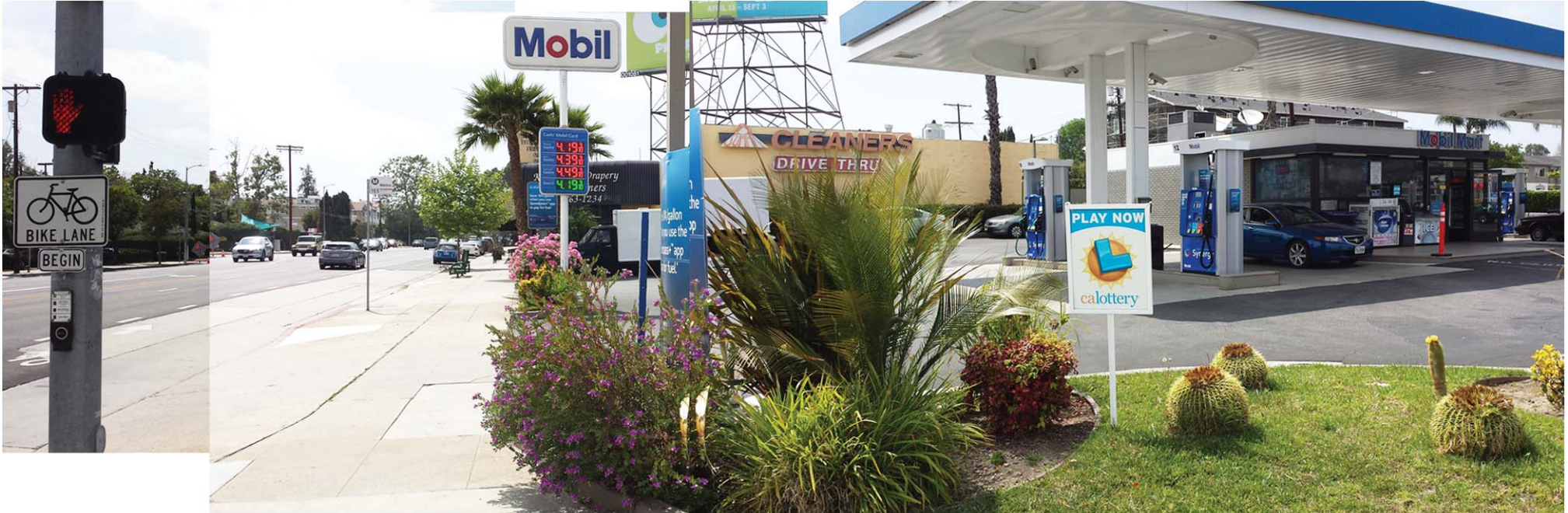
12 Facing West at the Southeast corner of the project property. Southeast corner of the property, partial East/South facade of existing fuel canopy and existing convenience store with conc. curb (tile and conc. finish on top). In addition, depicting existing landscape planter with conc. curb. at the Southeast corner at the intersection of Riverside Dr. and Laurel Canyon Rd. of the property. And the secondary price pole signage at South of Prop.
