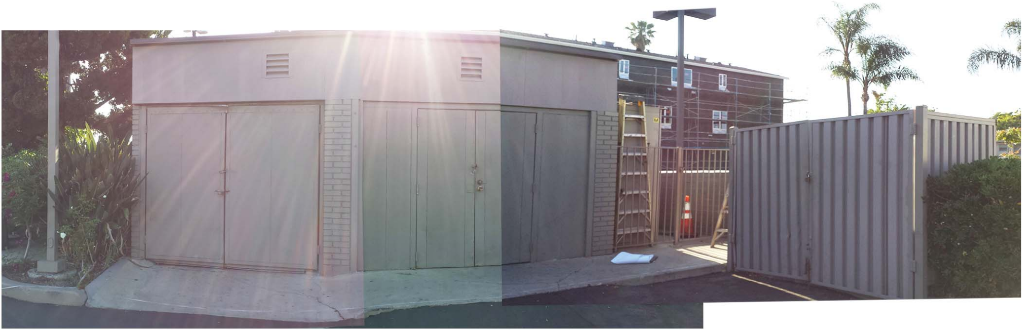
5 Facing West - North at the Northwest corner of the project property. Northwest of property, east facade of existing storage building (to be removed) and existing metal trash enclosure (to be removed and relocated).
