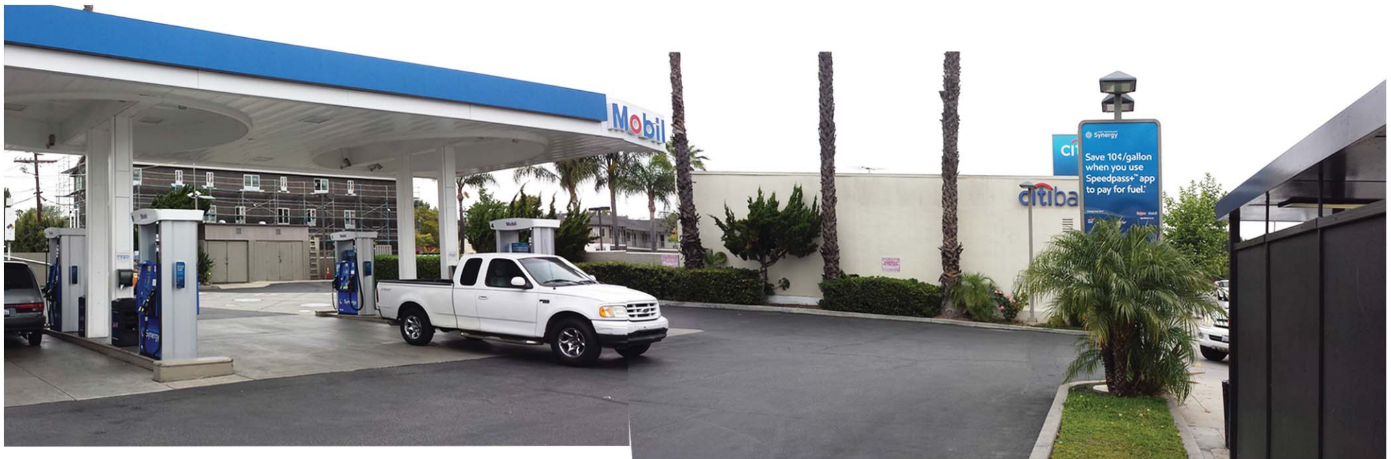
② Facing West - North at the east side of project property. East of property, East facade of existing fuel canopy with dispensers/ conc. curb. And depicting existing landscape planter along the east and north of property.
