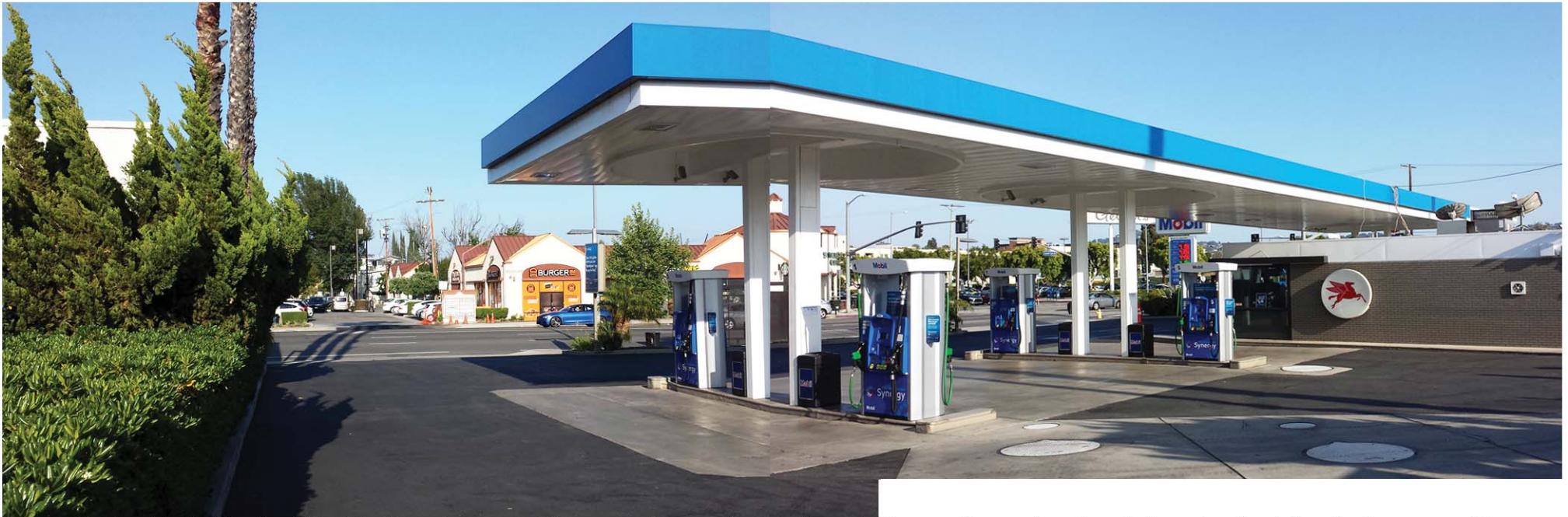
3 Facing East - South at the Northwest corner of the project property. Northwest of property, west and north facade of existing fuel canopy with dispensers/ conc. curb and North facade of existing convenience store with curb (tile and conc. finish on top). And depicting existing landscape planter with conc. curb. along the North of property.
