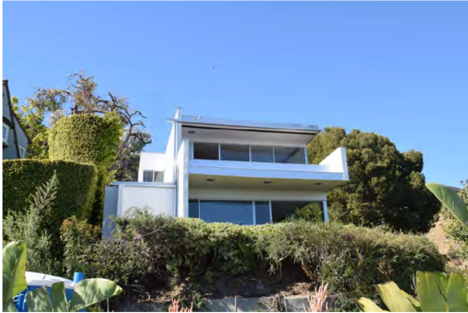
Figure 18. South elevation of Kun House II, facing Fareholm Drive. Camera facing north (Source: ESA, 2021)
