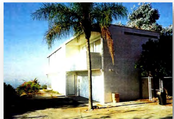
Figure 8. 1997 photograph of Kun House II, showing the double door feature (Source: Chris Hacker and Will Thomas)
