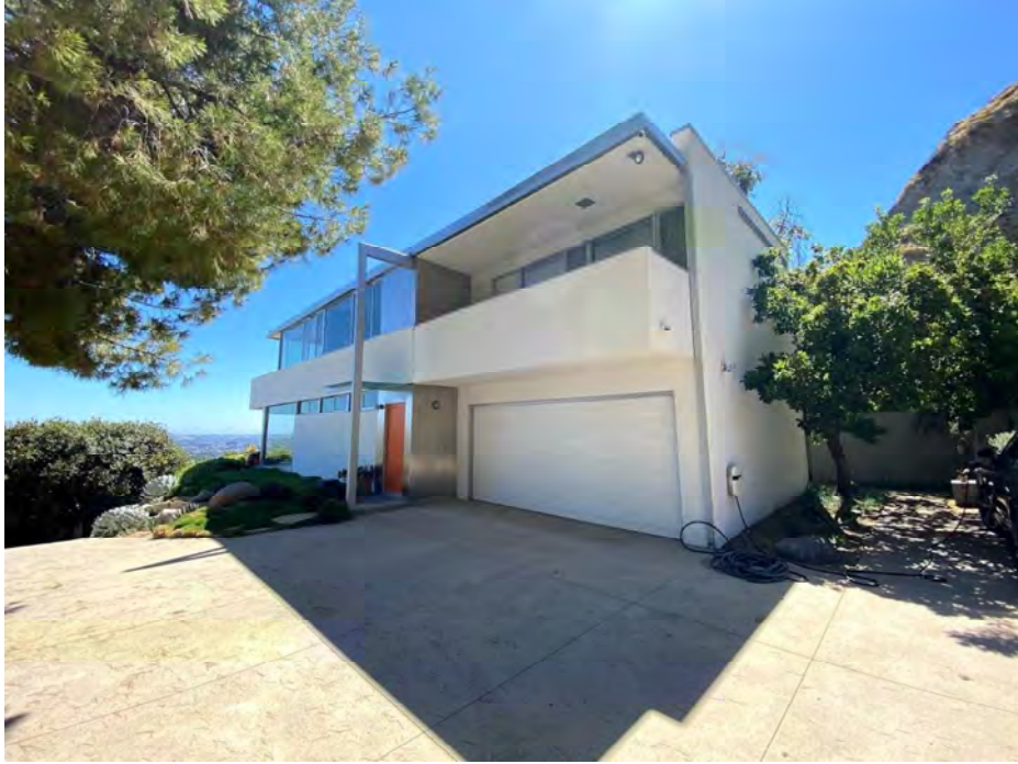
Figure 20. East elevation and north (rear) elevation of Kun House II. Camera facing southwest (Source: ESA, 2021)
