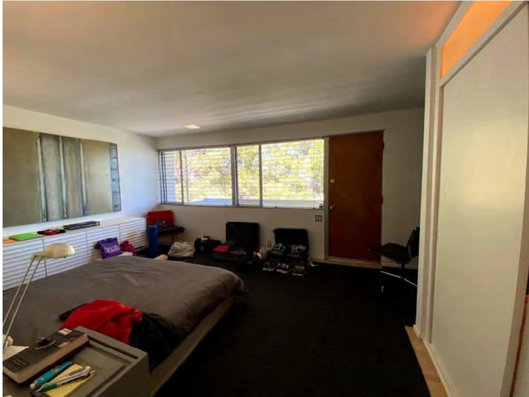
Figure 36. Second-story guest bedroom with original single-leaf door leading to a balcony and original closet built-in with glass transom light above. Camera facing east (Source: ESA 2021)
