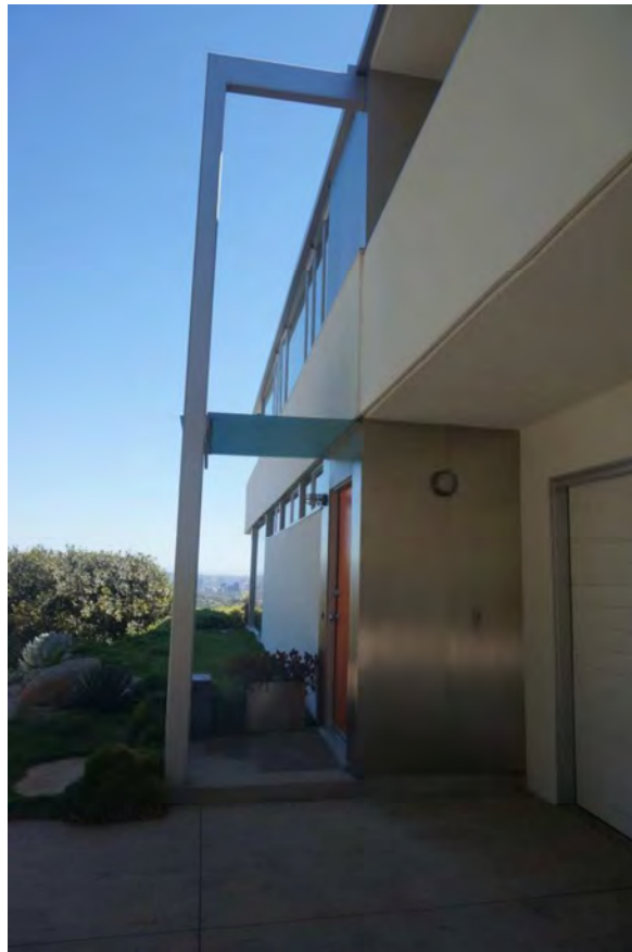
Figure 21. Detail view of the east elevation's spider leg. Camera facing south (Source: ESA 2021)
