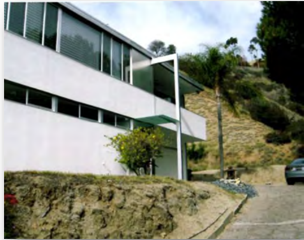
Figure 3. 2008 photograph of the landscaping around Kun House II after the landslide and prior to the landscape re-design (Source: Chris Hacker and Will Thomas)
