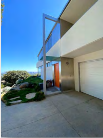
Figure 9. 2021 photograph of Kun House II's spider leg on its east elevation. Camera facing northwest (Source: ESA 2021)
