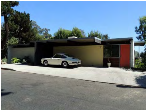
Address: 3319 Tareco Drive Name: Jason Hailey House Architect: John Blanton for Richard Neutra Date: 1959
