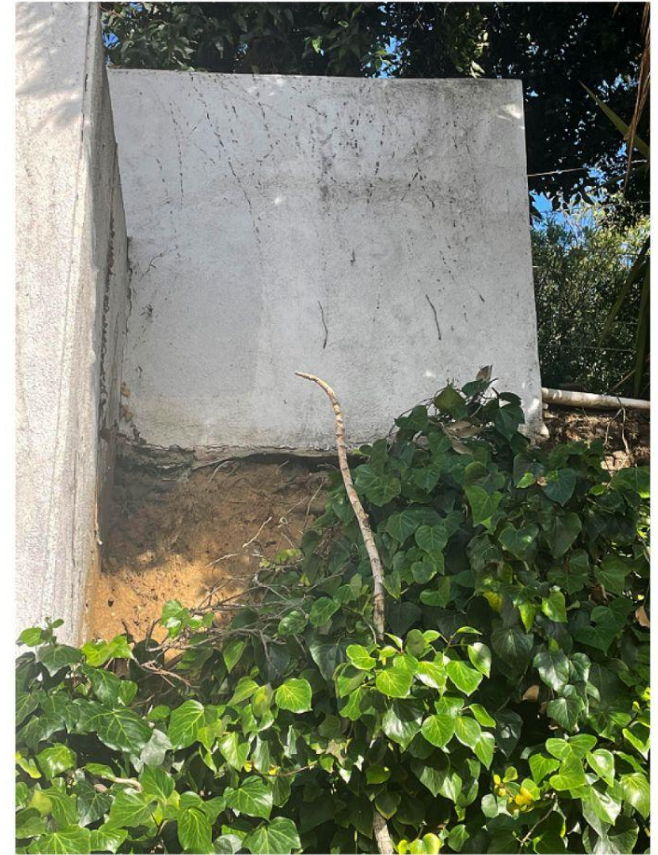
DUNDEE RETAINING WALL / CURRENT PHOTOS OF UNSUPPORTED WALL + SLOPE
