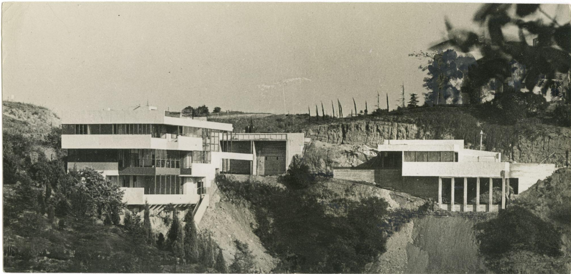
DUNDEE RETAINING WALL / ARCHIVAL PHOTO (1929)
