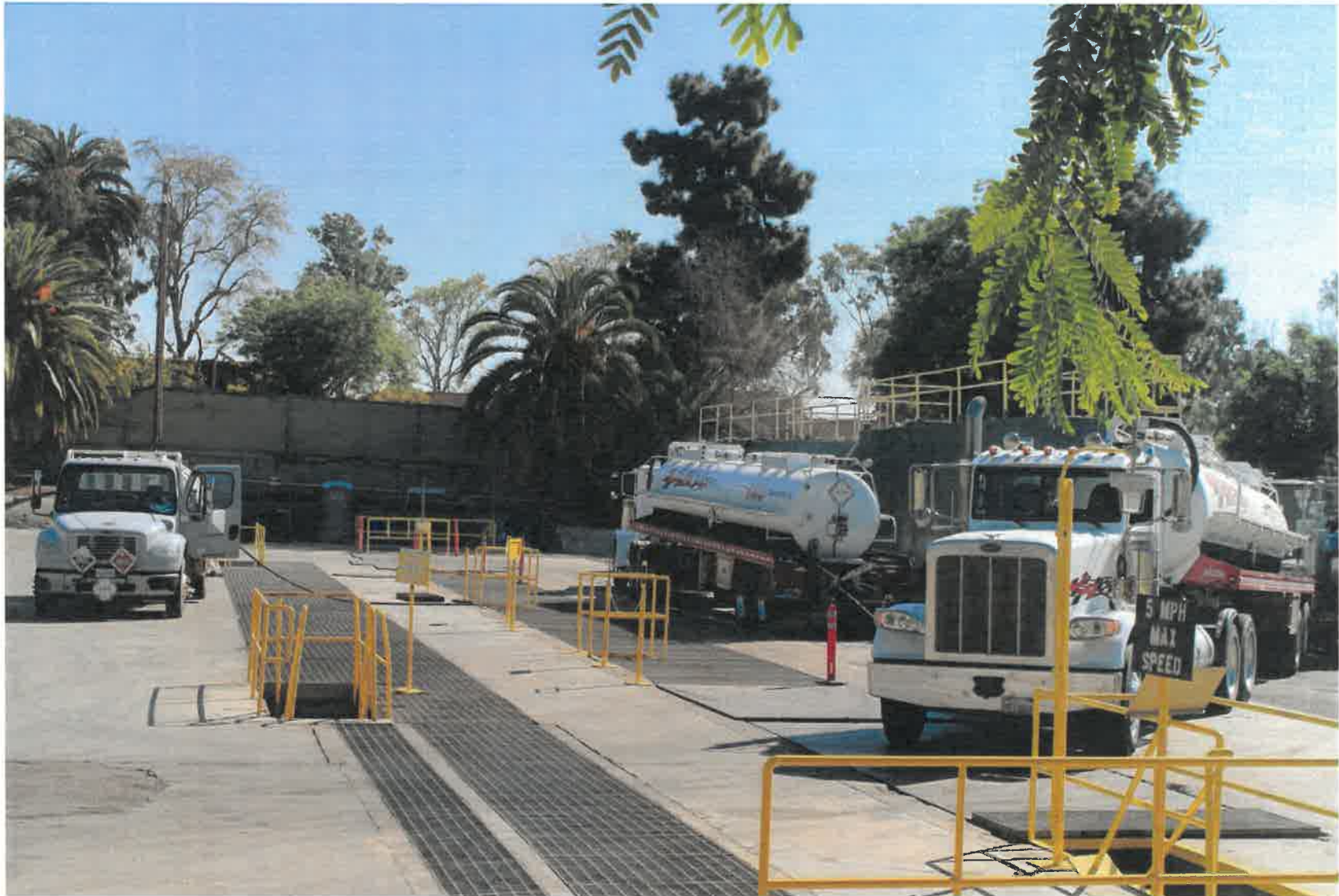
Figure 21 - An acid tanker (on left) pumps acid down well while two vacuum trucks remove fluids from a degassing of the FWKO tank (2/24/2021)
