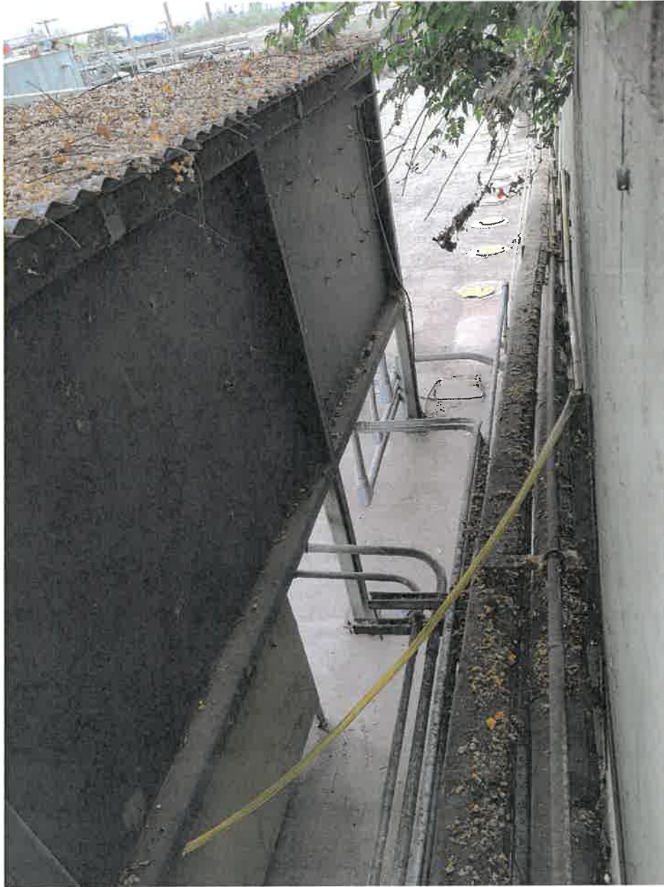
Photo 6: Clear tubing strung along the shared wall with the AIDS Healthcare Foundation, pulses with acid-yellow liquid from what appears to be an odor counteractant diffuser.
