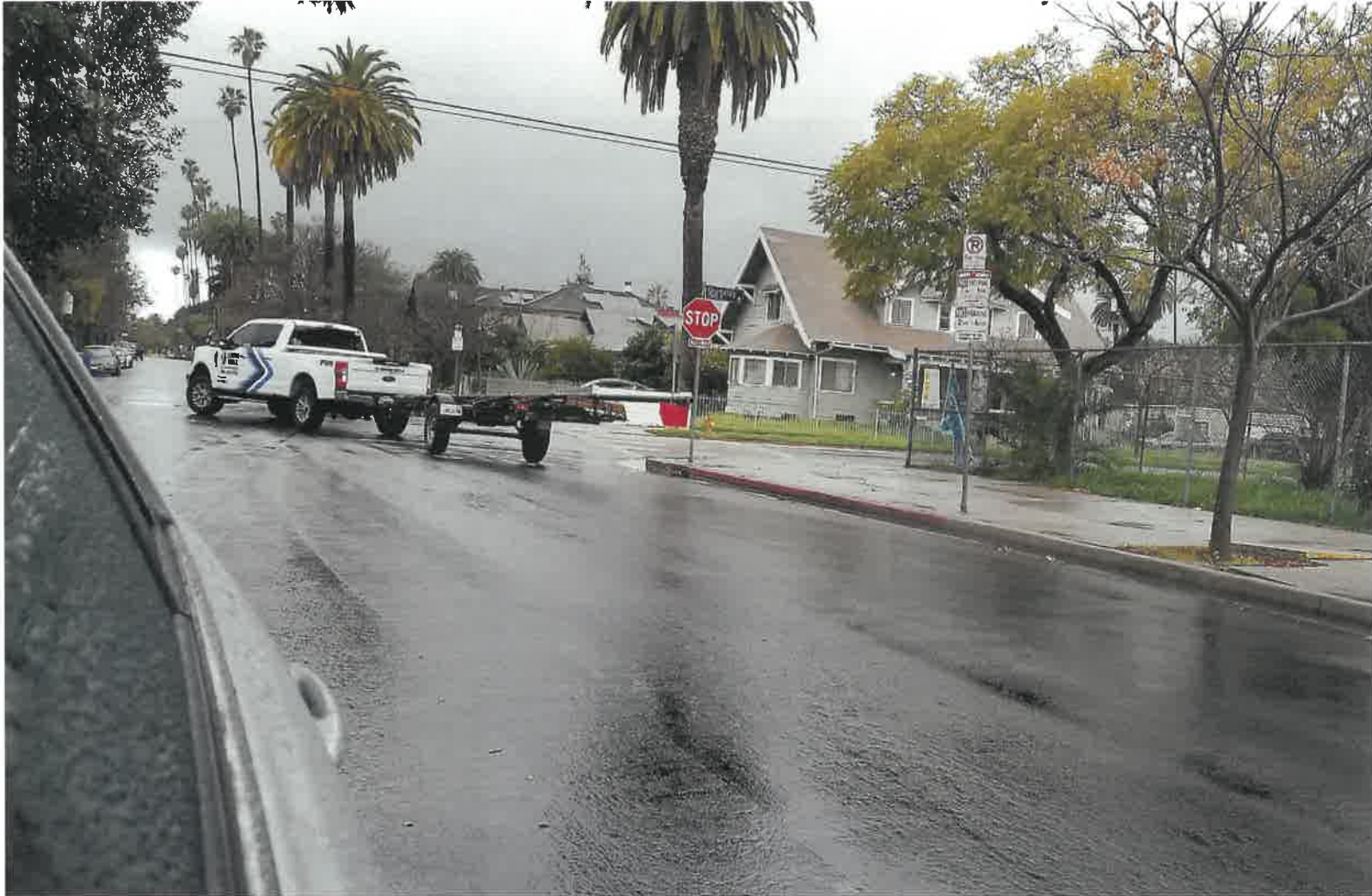
Figure 19 - Snow Well workers drive a large pipe past 24th St Elementary School and the Widney High School on 24th Street.
