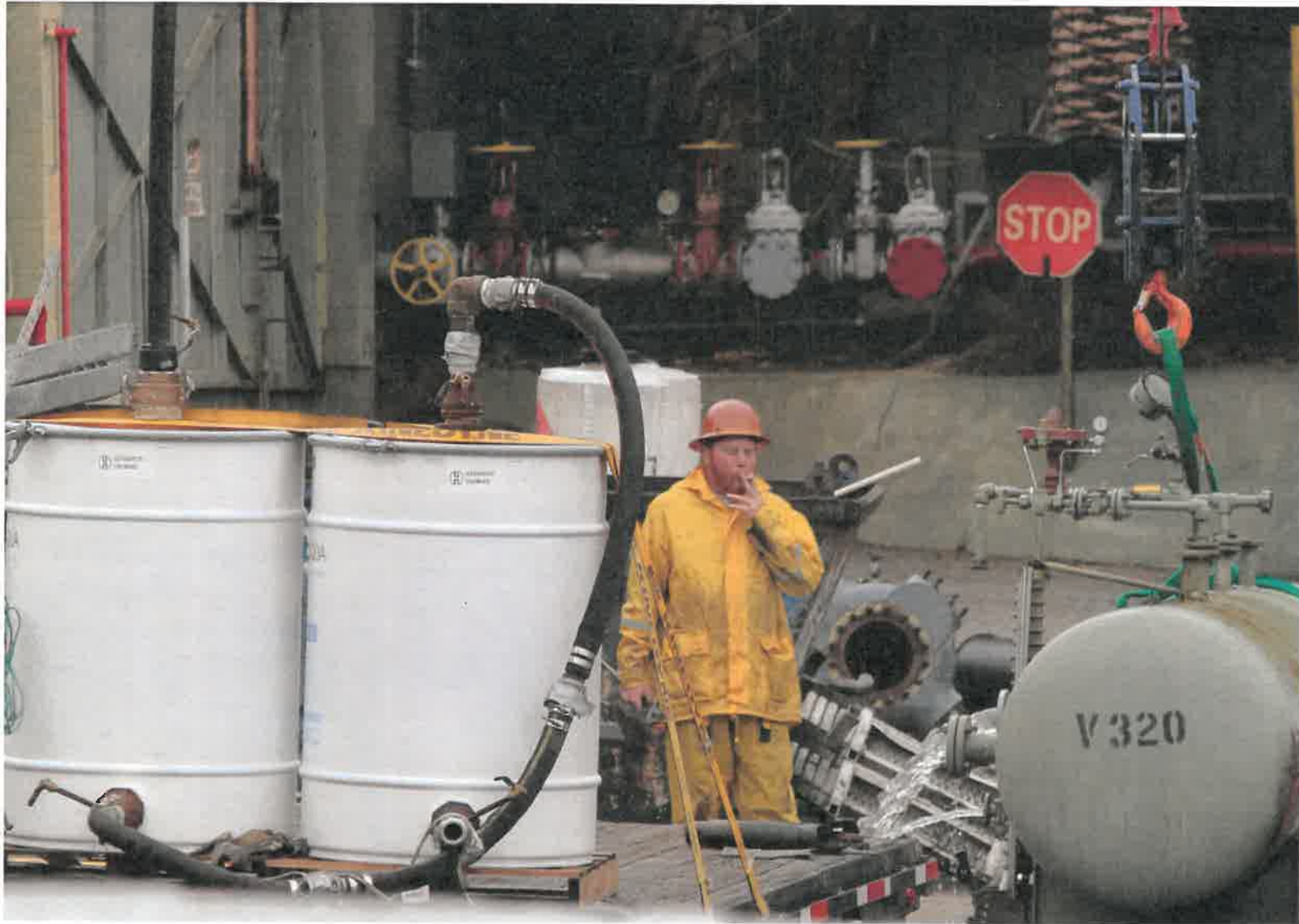
Figure 28 - Worker smokes on the drill site (3/15/2021)
