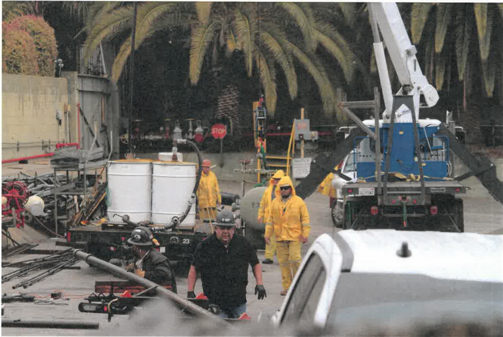
Figure 18 - Snow Well workers secure a large pipe to a trailer (3/15/2021)
