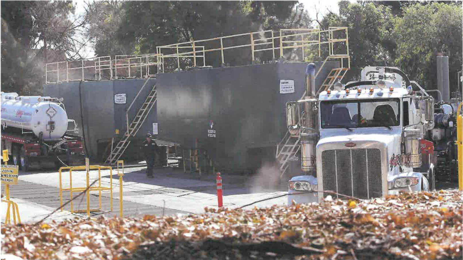
Figure 22 - Visible fumes float away from both vacuum trucks (2/24/2021)
