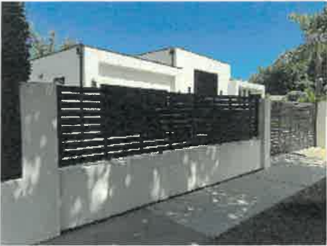
BLOCK CONCRETE WALL
