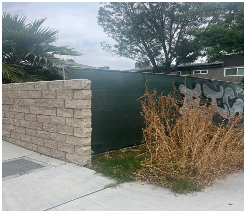
8. Taken from Northwest corner of project site, facing Southeast into project site.
