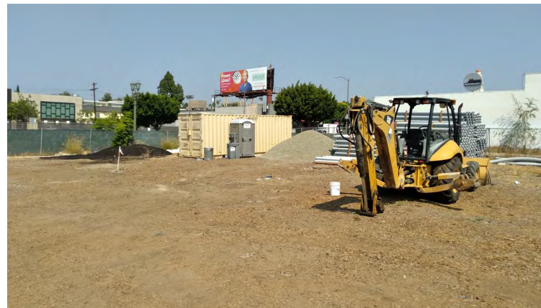
5 VIEW OF WEST SIDE OF SITE LOOKING NORTH
