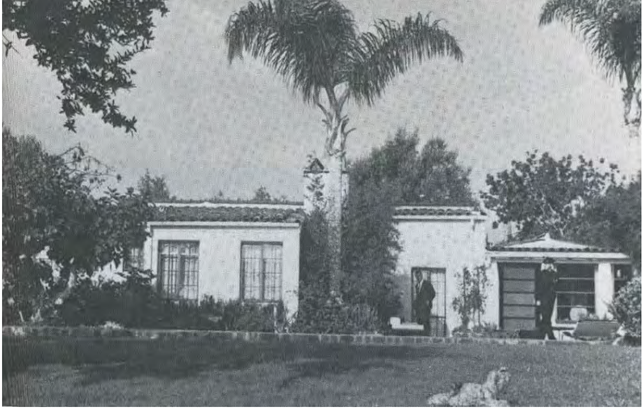
Rear (west) façade, view looking east. Courtesy of CursumPerficio.net.
