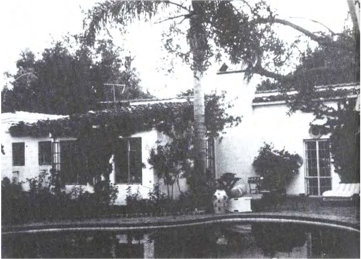
Rear (west) façade detail, view looking east. Courtesy of CursumPerficio.net.
