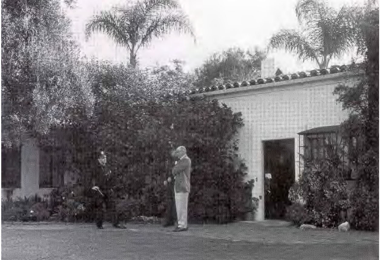
View looking northeast toward the primary entrance. Courtesy of CursumPerficio.net.
