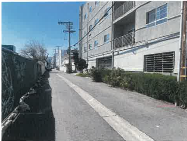
12. Taken from the NE corner of the project site, W into the adjacent alley.
