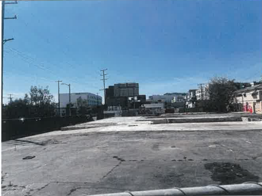
9. Taken from the E side of the project site, W into the site.
