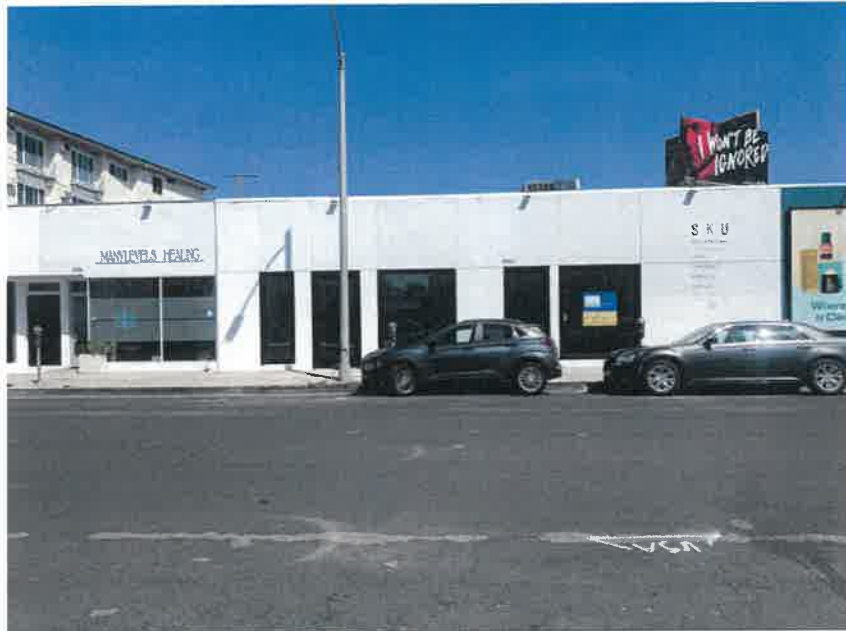
10. Taken from the SE corner of the intersection of Magnolia Blvd and Van Nuys Blvd, NW into the project site.
