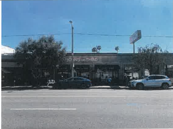
3. Taken from the SW corner of the project site, S across 3 rd Street.
