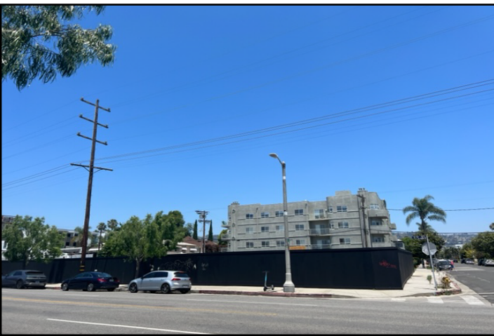
View 3: From the south side of 3rd Street, looking north at the Project Site.
