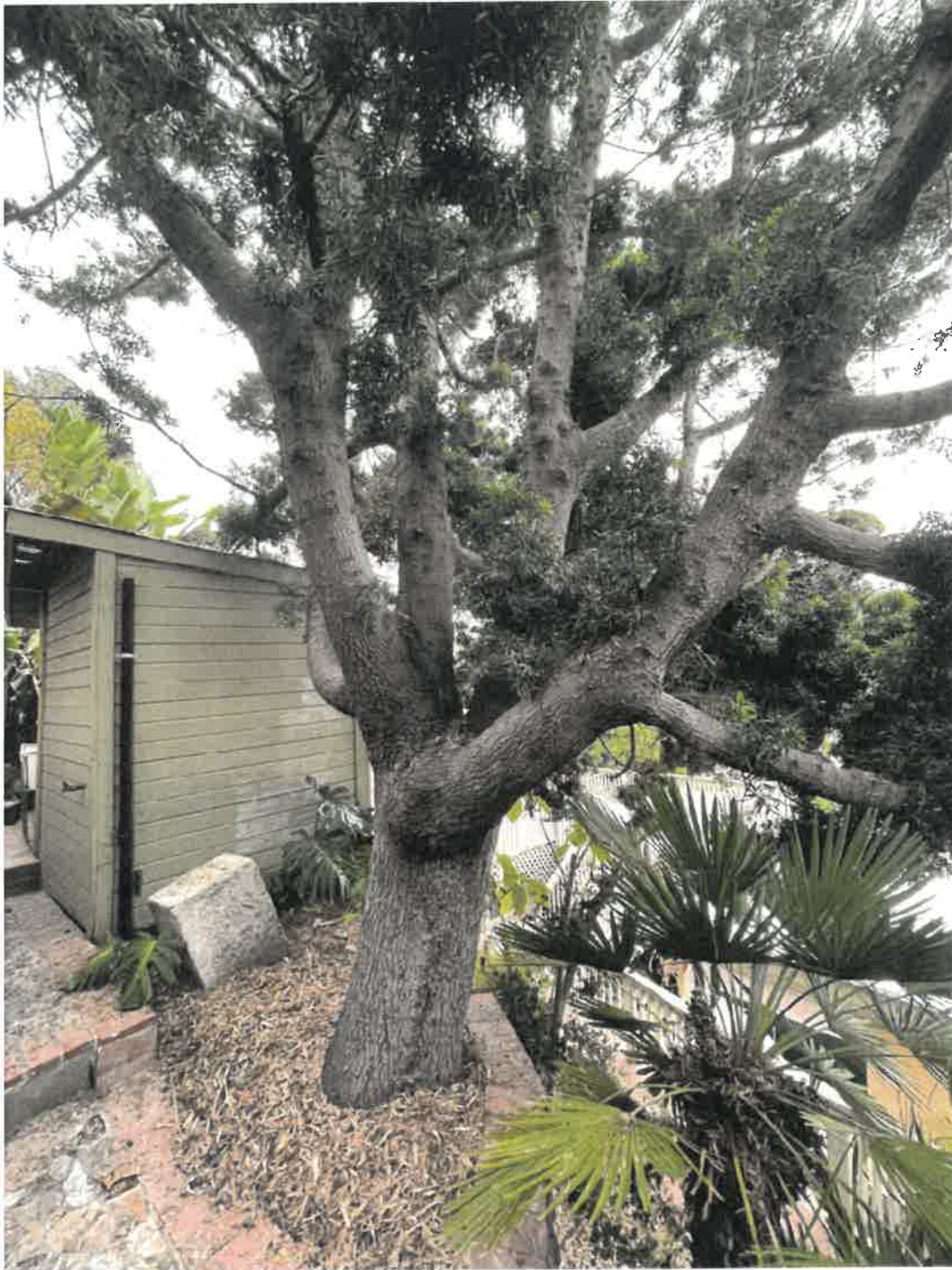
PHOTO 8 - Fern Pine - Afrocarpus falcatus tree located in slender planter. This tree is heaving the hardscape and low retaining walls. This tree will require removal due to the grading and remediation of the site.
