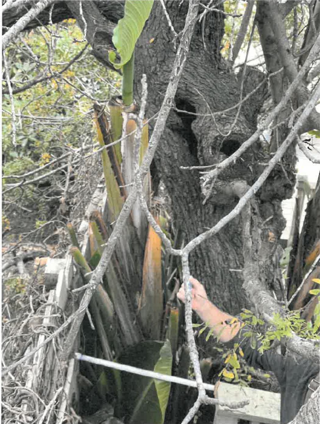
PHOTO 1 - Black Walnut Tree #1 - This tree is growing in an elevated vintage retaining wall, and shifting and cracking the wall frontage. This old black walnut tree is in senescence, has a decayed trunk that appears to be coalescing with lower trunk decay. This tree is a removal candidate due to the steep terrain, grading and soils remediation, removal of the concrete wall for site remediation, and the lack of ability to retain this tree. This tree will be removed and replaced at a 4:1 ratio with a minimum 15 gallon size container or largest available nursery size.
