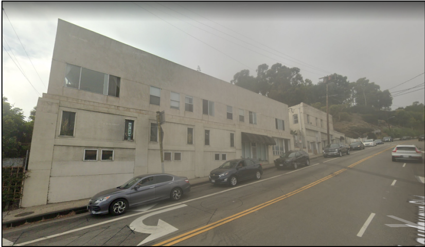
2- and 3-story buildings located at 101-121 N. Chautauqua Blvd.
