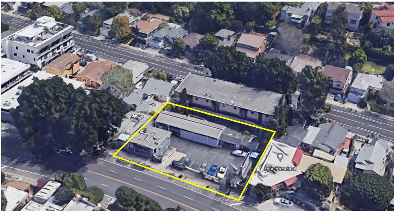
Figure 2. Aerial view of subject Property from Hyperion Avenue, facing east
