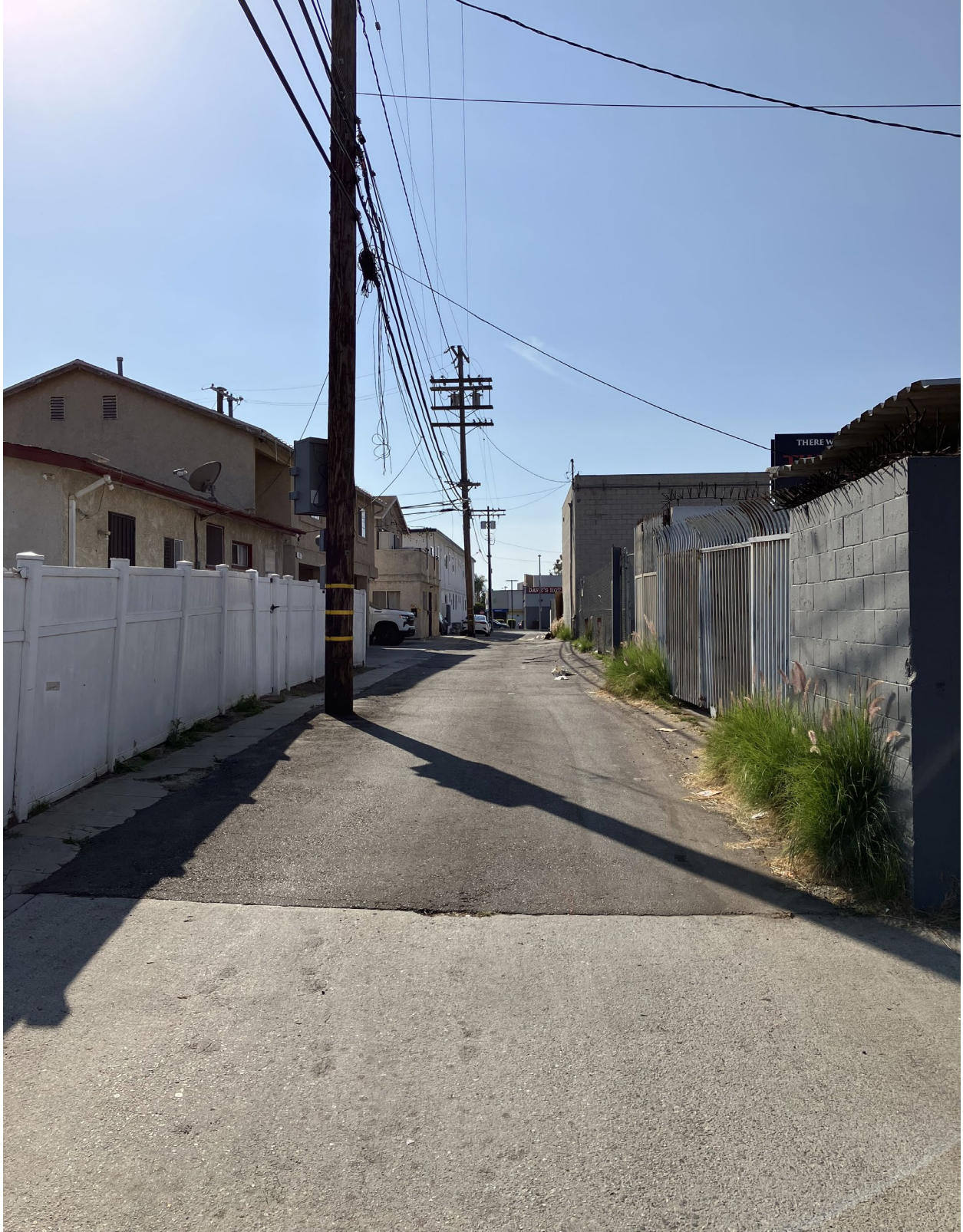
(Note: proximity between Project site and Perez Family Child Daycare. The two properties are separated by an alleyway.)
