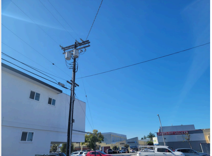
32. Pole-mounted transformers
