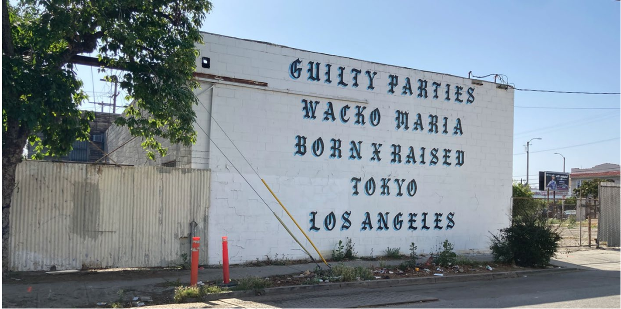
13. Taken across Catalina St. towards the SE corner of the project site
