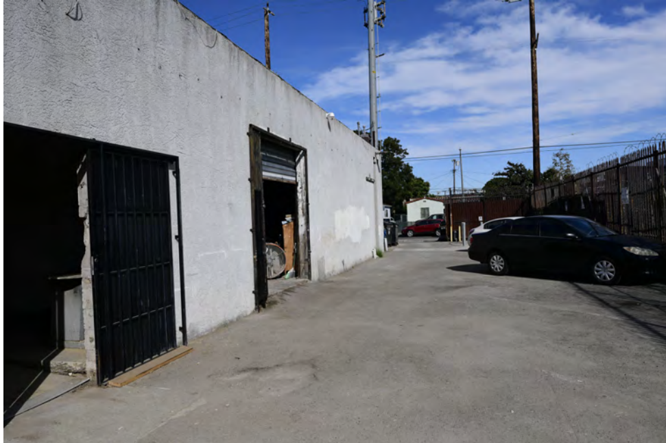
Former loading dock, back of Cadet Records. 2023 (J. Kress)
