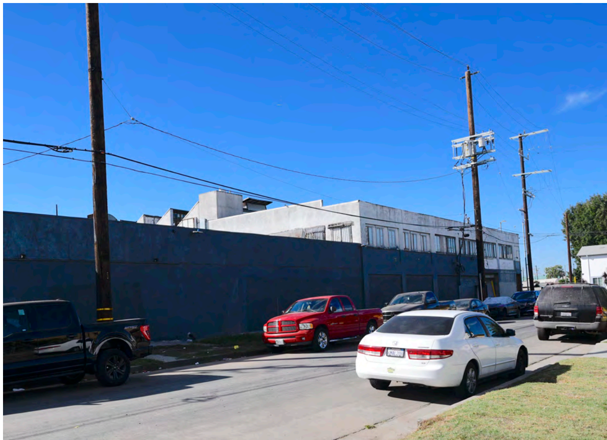
58th Street side of Cadet Records showing sawtooth roof/skylights. 2023 (J. Kress)
