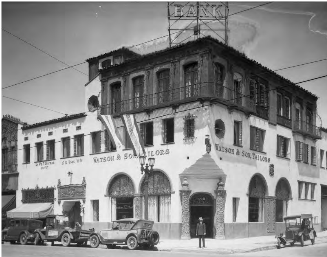
Baine Building / 6601 Hollywood Boulevard Gogerty & Weyl (1926) Photo: University of Southern California Digital Library
