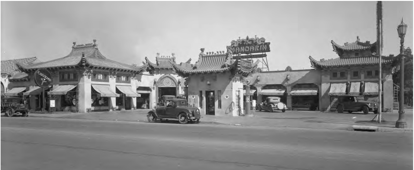
Mandarin Market / 1234-48 Vine Street (demolished) Gogerty (1929) Photo: California State Library
