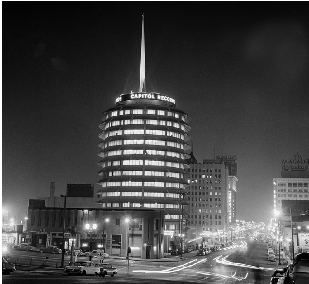
Gogerty Building / 6274-84 Yucca St Gogerty (1930) Photo: LADWP (1958)
