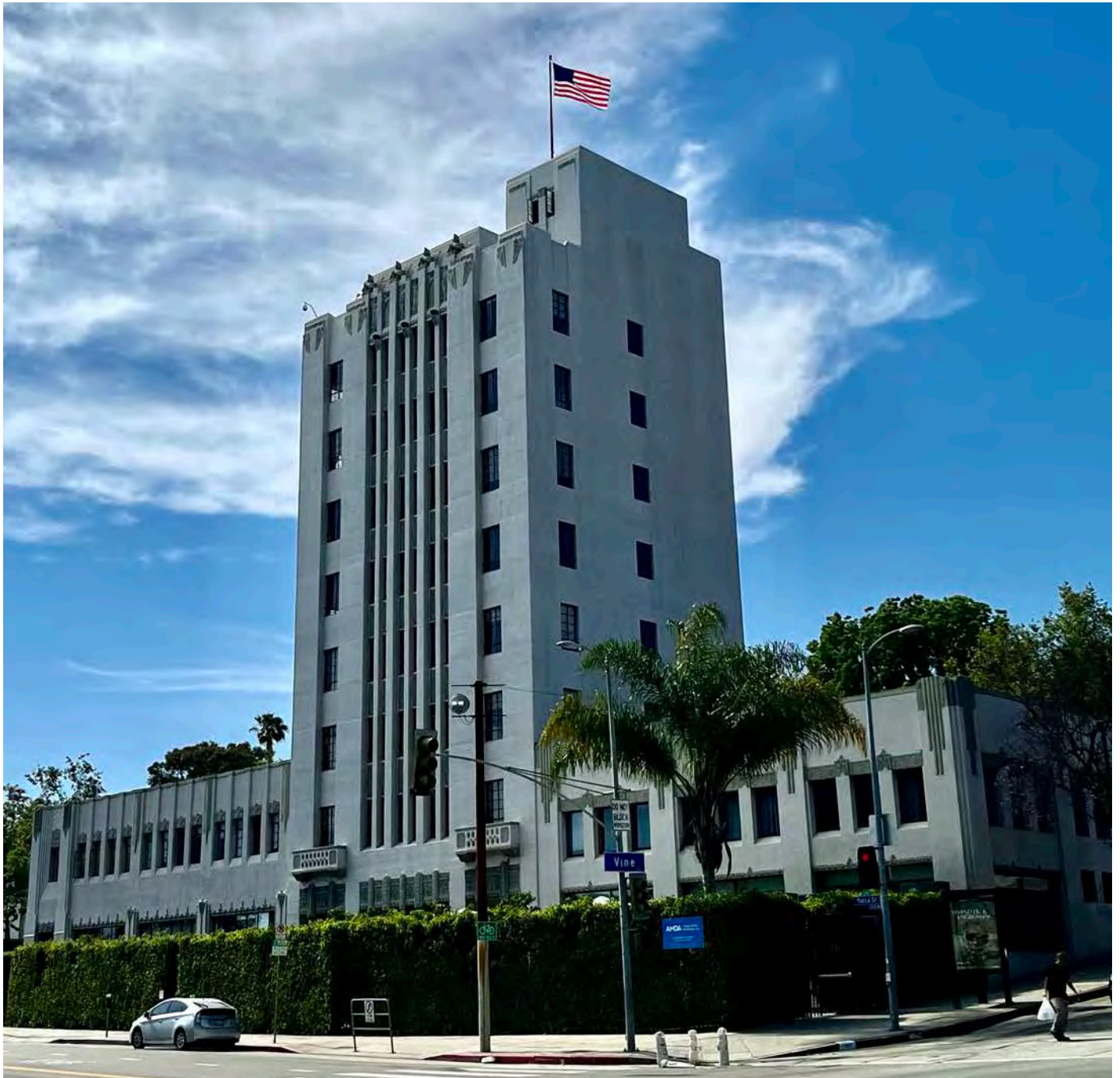
2023: Looking northwest at the Yucca-Vine Tower
