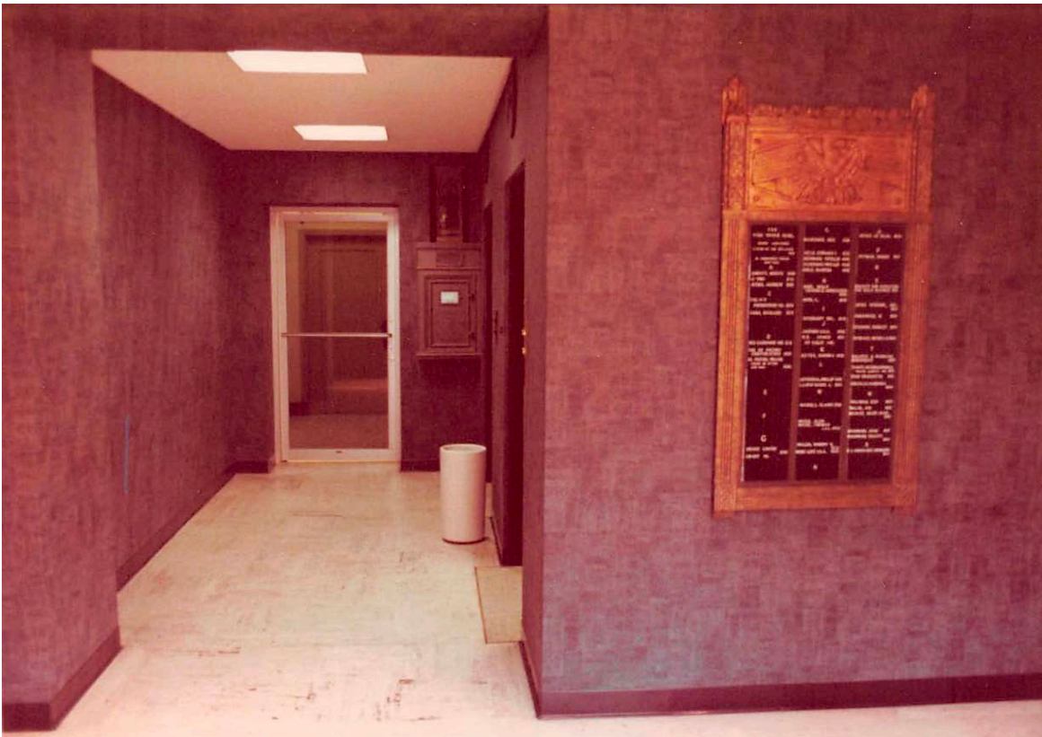
1977: Entrance lobby and elevator lobby, with original directory (photo courtesy of the De Pietro Family, Yucca-Vine Tower owners 1971-2003)
