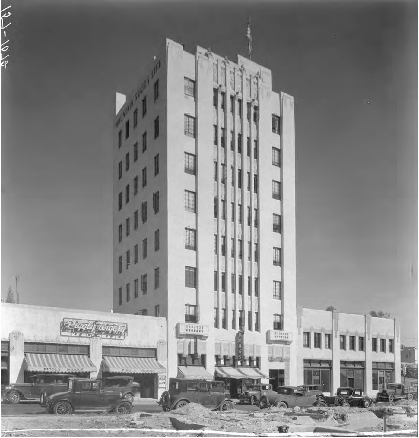
1930: Mountain States Life Building and its new east wing (California State Library)
