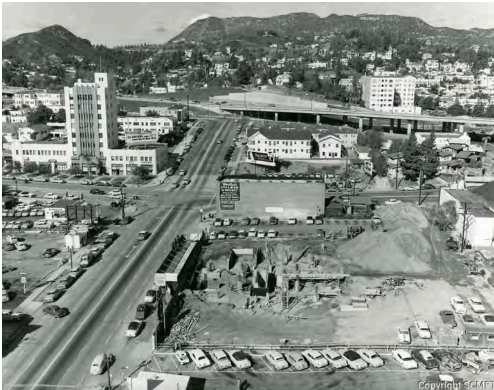
1955: Amid Capitol Records construction (HollywoodPhotographs.com)
