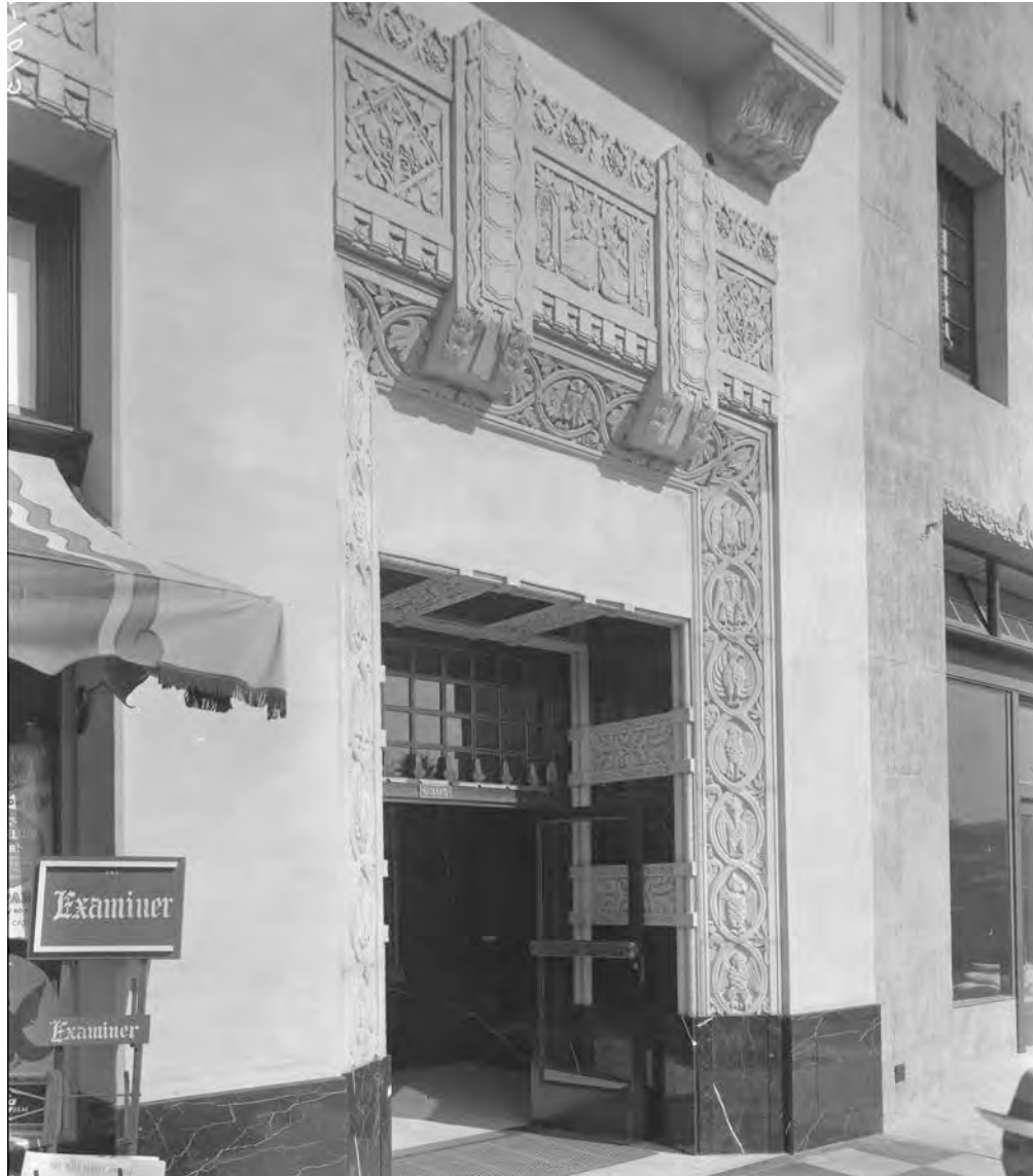
main entrance at 6305 Yucca in 1930 (California State Library)
