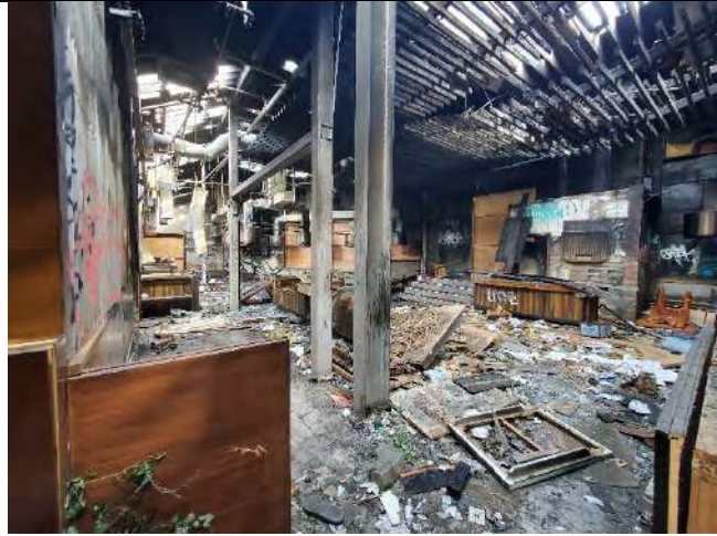
Photo (5) View of subject site building interior.
