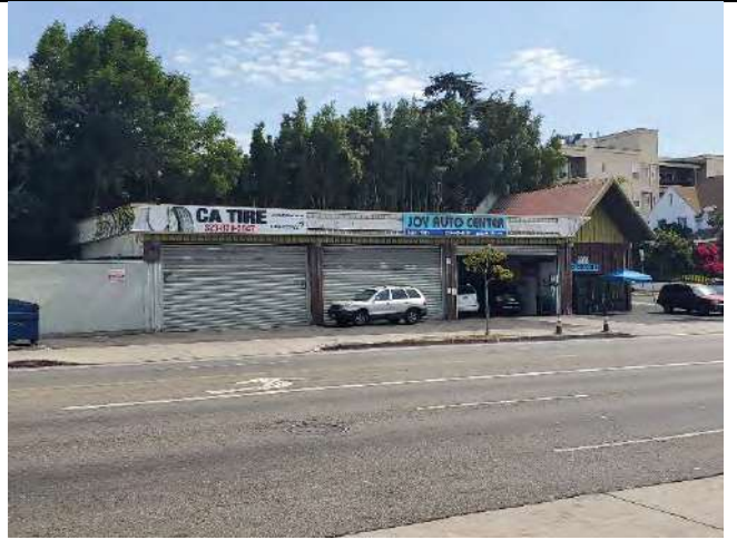
Photo (9) View of east neighboring property, CA Tire and Joy Auto Center, addressed as 3355 West Olympic Boulevard.
