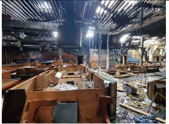
Photo (6) View of subject site building interior.
