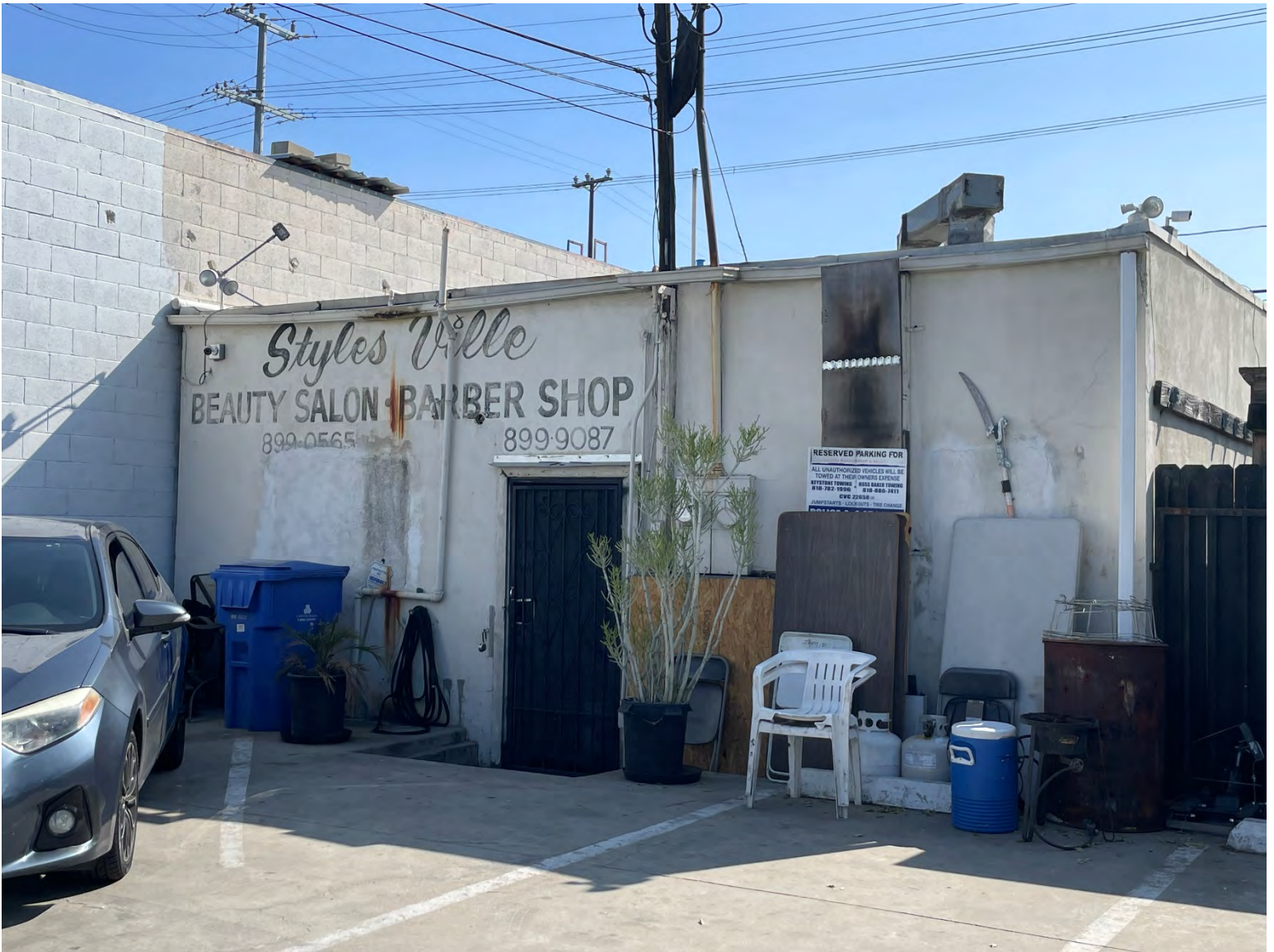
Rear (northwest) façade, view southeast (ARG, 2023).
