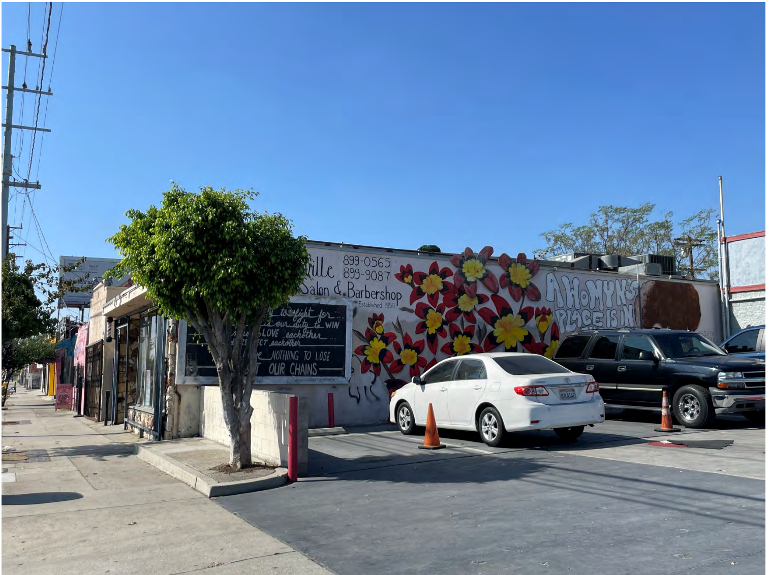
Northeast façade, view southwest (ARG, 2023).
