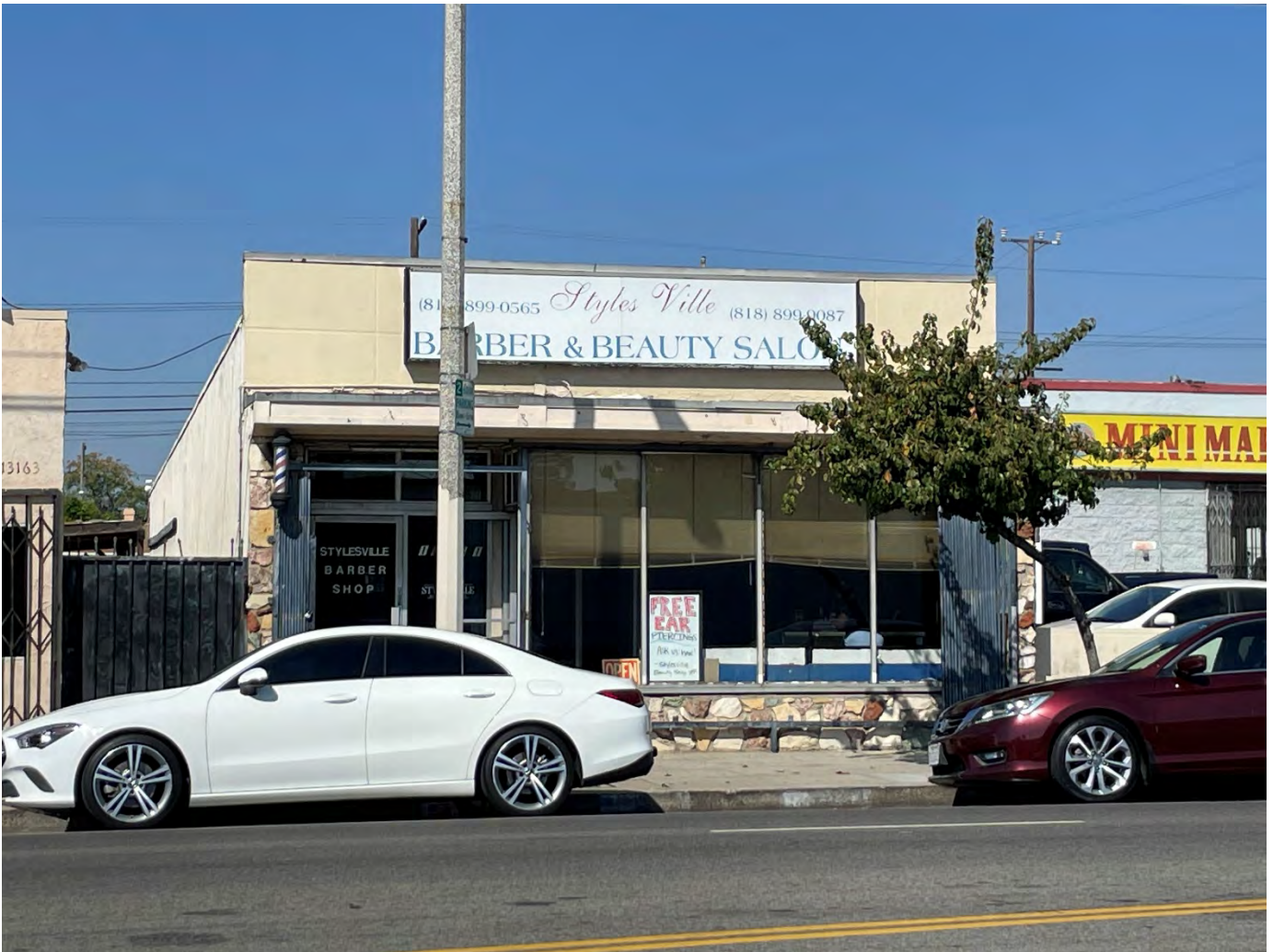
Southeast (primary) façade, view northwest (ARG, 2023).
