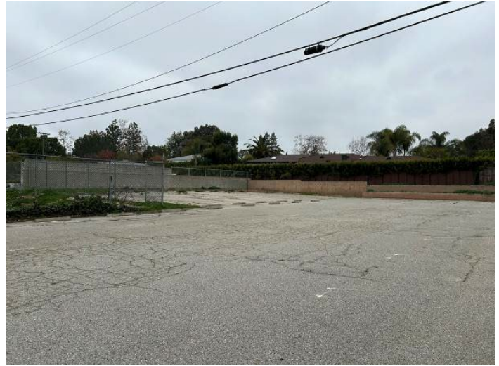
Barry Building rear surface parking.
