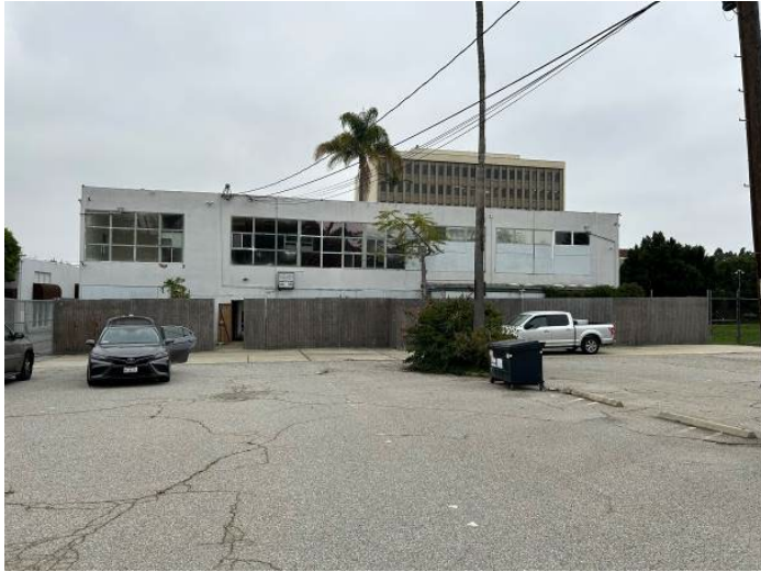
Barry Building, rear side.
