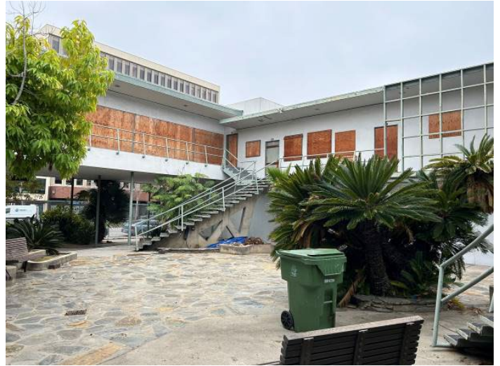
Barry Building courtyard. Note plywood over windows.
