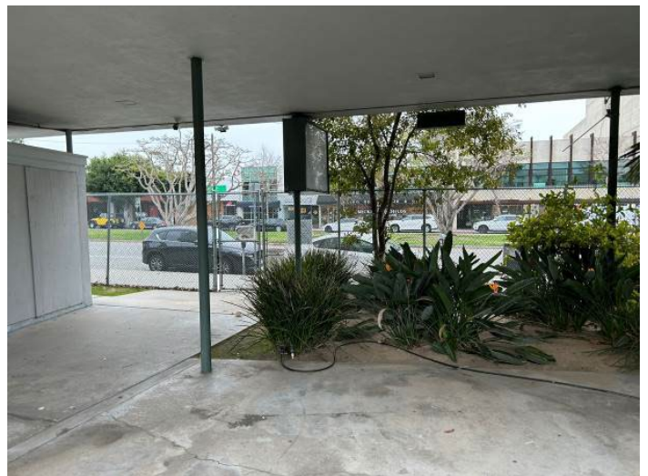
Barry Building "soft" ground floor.
