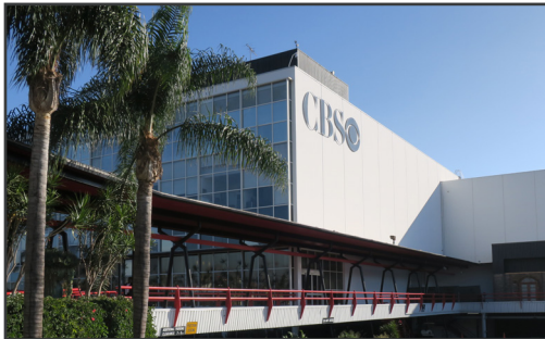
Fig. 26. View of the northwest corner of the Service Building. 2017.
