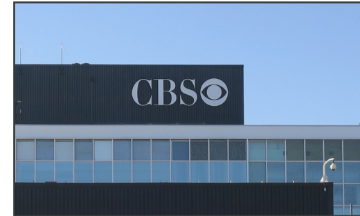
Fig. 22. Detail of the east elevation of the Service Building. 2017.
