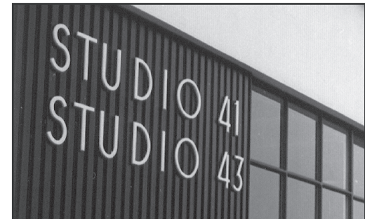
Fig. 16. Detail of the west elevation of the Studio Building. 1952.
