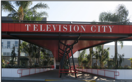
Fig. 18. Detail of the Bridge. 2017.
