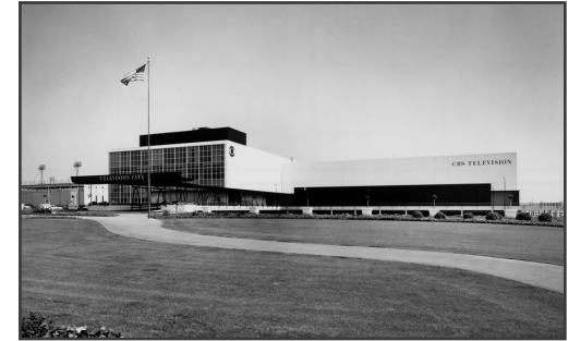
Fig. 11. View of the northwest corner of the Studio Complex. c. 1958.
