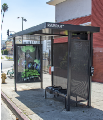
1.2.1 BUS STOP SHADE STRUCTURE
