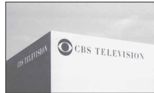
Fig. 12. View of southwest corner of the Studio Building. 1952.
