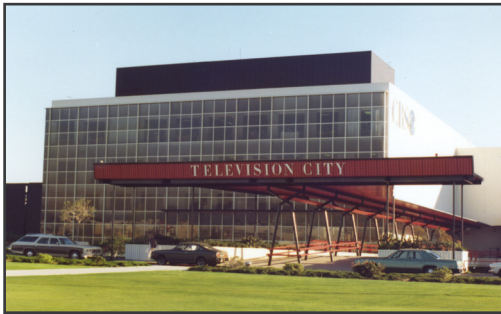
Fig. 14. View of north elevation of Service Building and Bridge. c. 1978.
