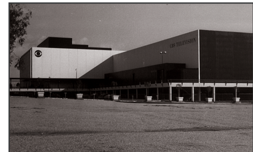
Fig. 28. View of the northwest corner of the Studio Complex. 1952.
