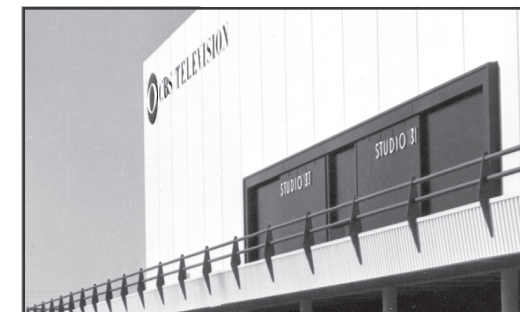
Fig. 24. Detail of the south elevation of the Studio Building. c. 1958.
