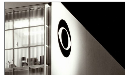
Fig. 17. Detail of the northwest corner of the Service Building. 1955.
