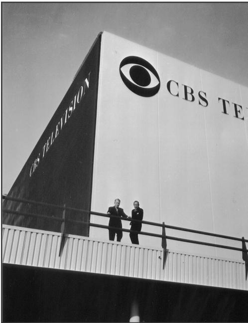
Fig. 7. View of the southwest corner of Studio Building, c. 1958.
