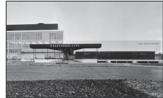
Fig. 15. View of the north elevation of the Studio Complex and Bridge. 1956.
