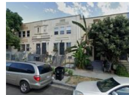
Columbia Place, West Lake Source: Google Earth
