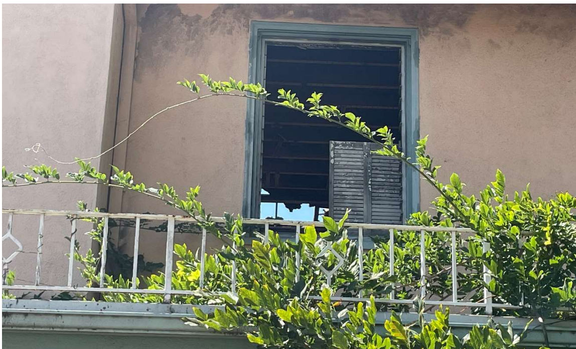
Image 8: Missing window and gutted interior, view east from driveway
