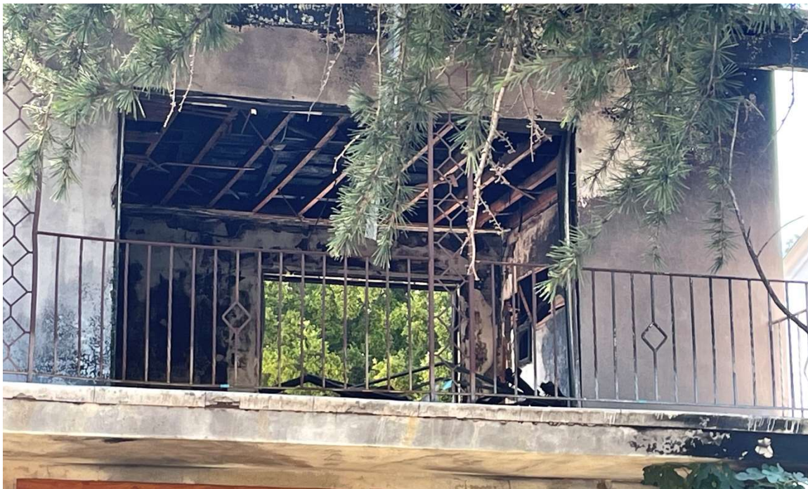
Image 6: Missing doors at primary (south) façade and gutted interior, view southeast from driveway
