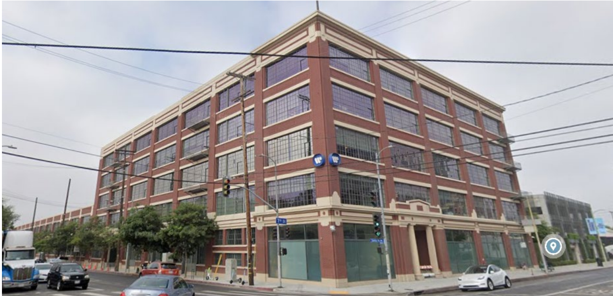
View of the Existing Warner Music Group Building from 7th Street and Santa Fe Avenue
