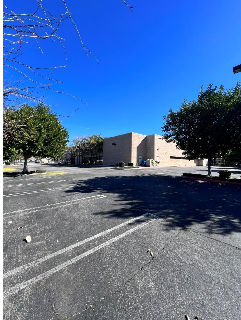
8) Northwest corner view of the structure and lot
