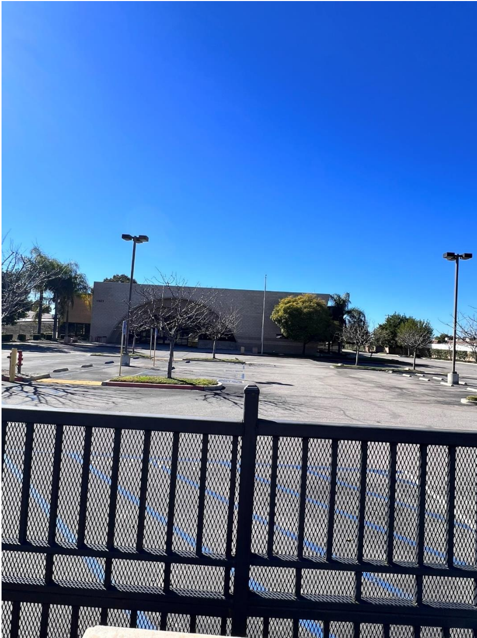
3) View from Glenoaks entrance towards existing structure
