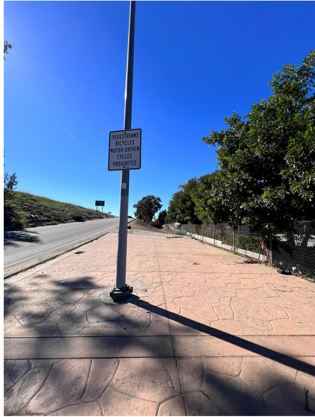
20) Side of freeway ramp adjacent to the structure
