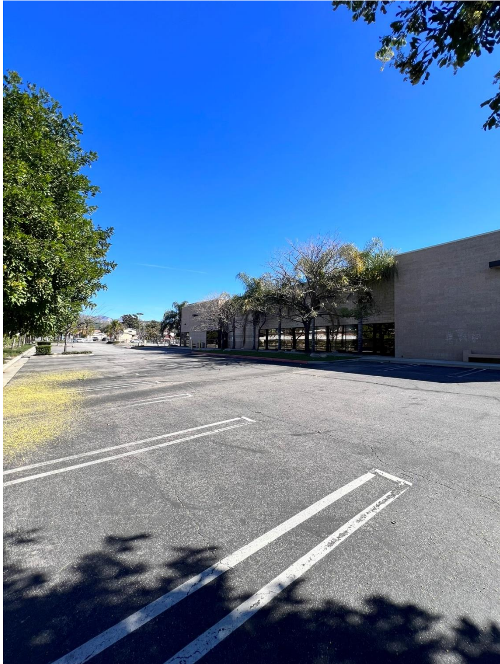
7) Side view of the structure towards Glenoaks entrance
