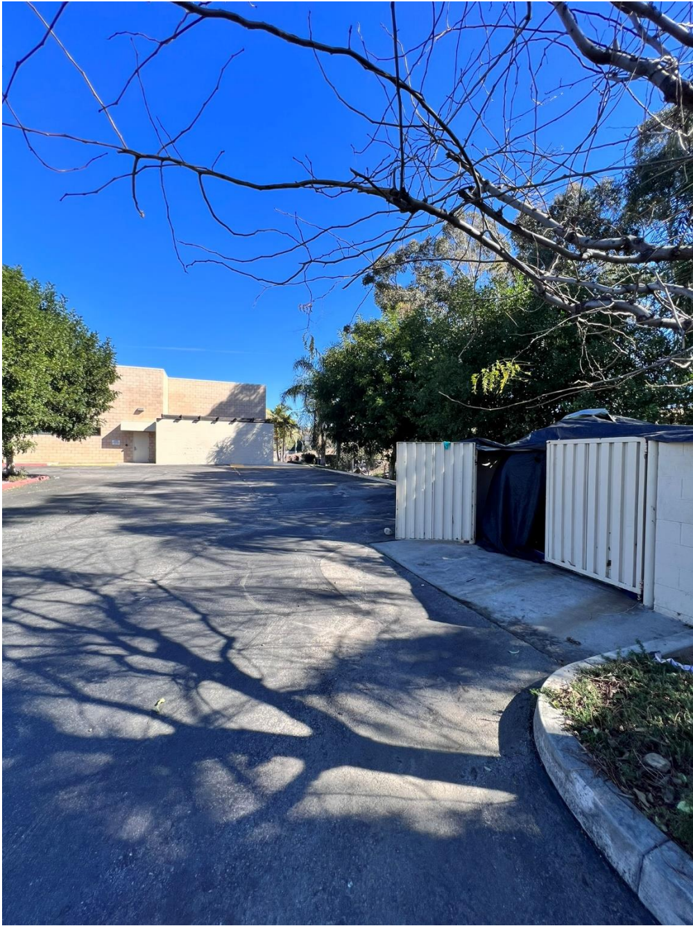
11) Southwest corner view of the back of the structure
