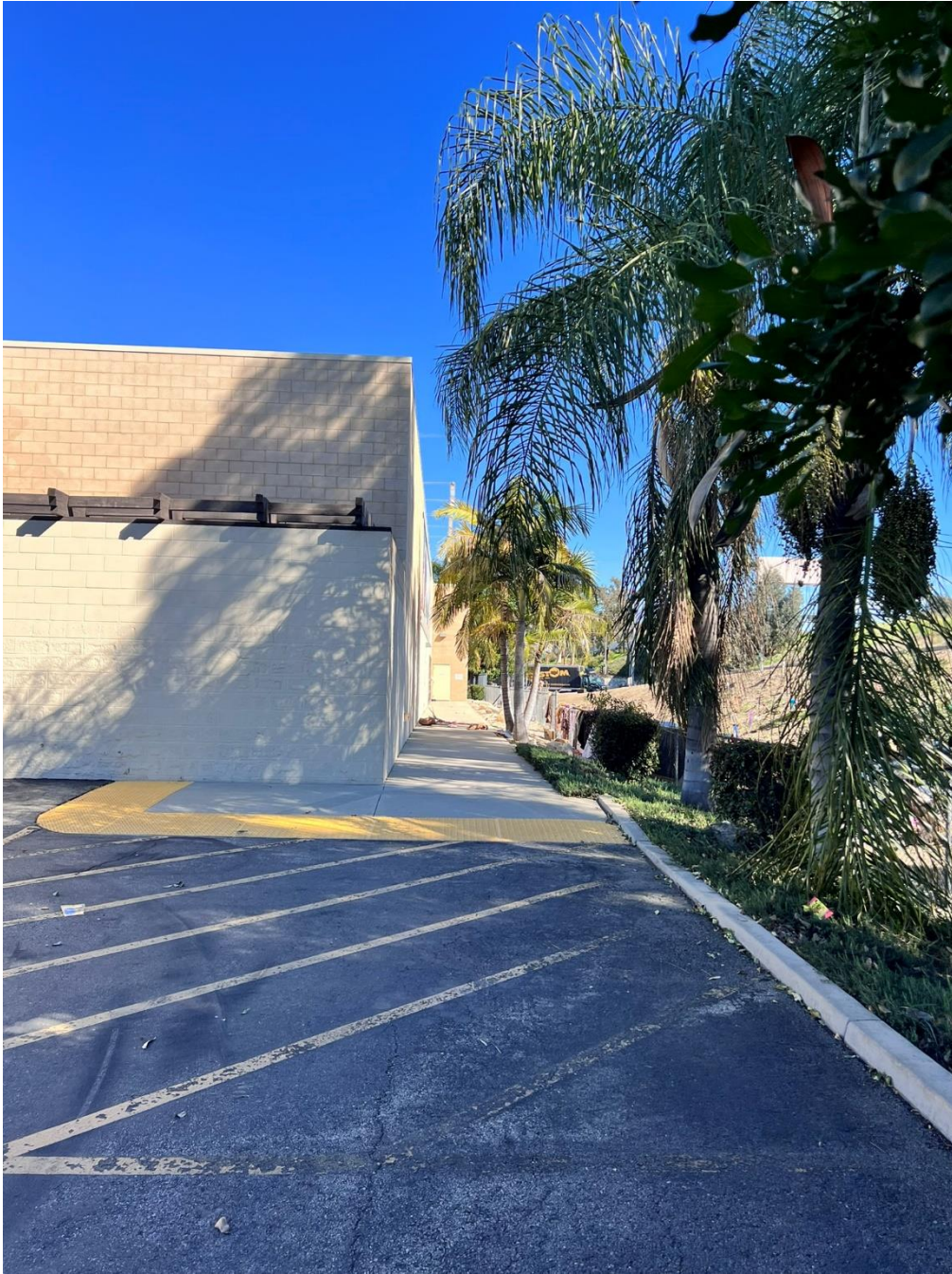
13) Back of the structure towards the front, next to freeway ramp
