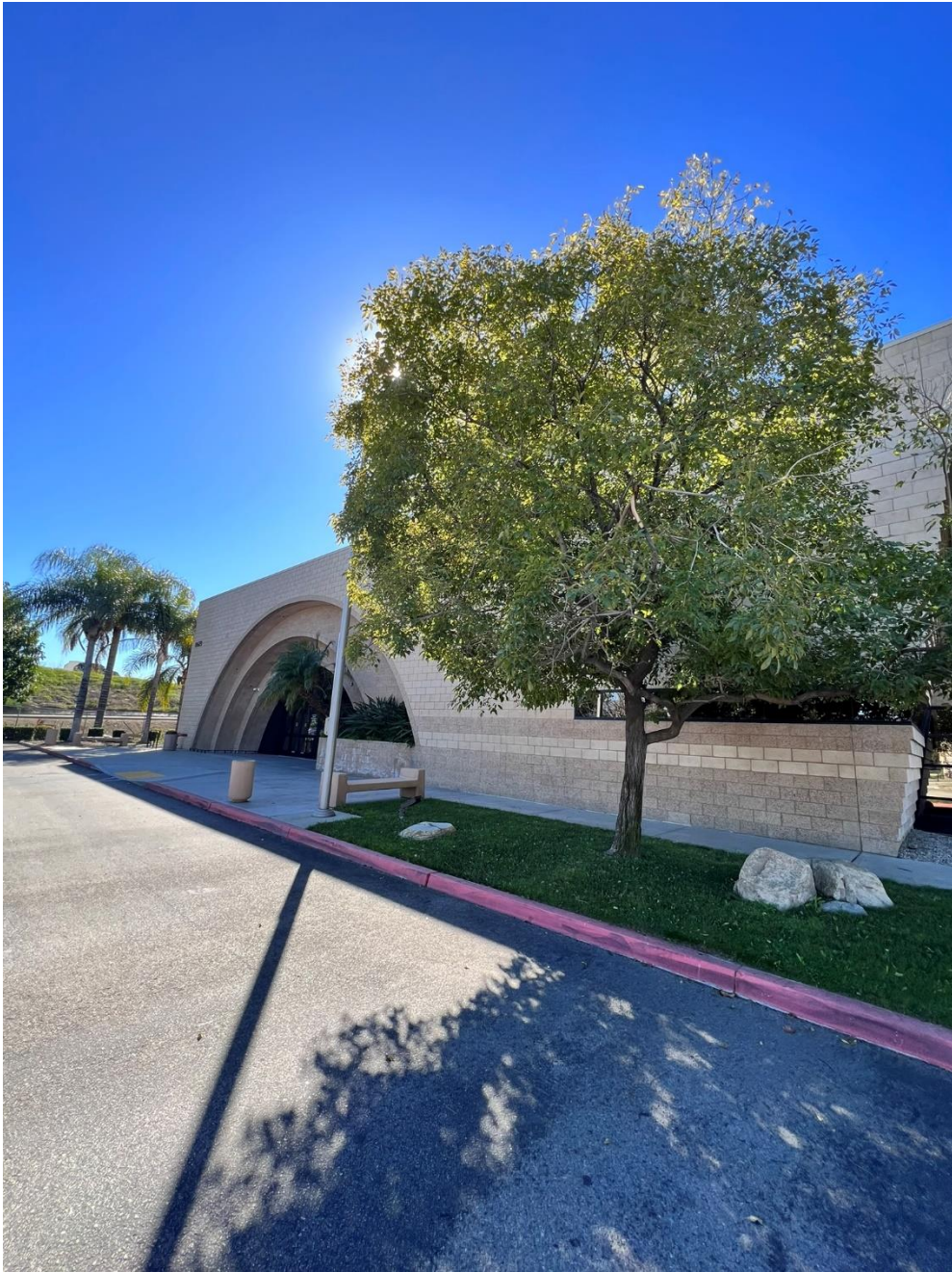
15) Up close front of the structure towards freeway ramp
