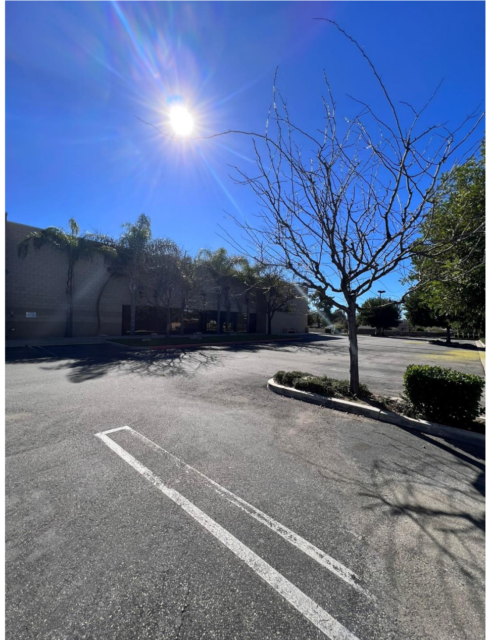
6) Northwest side view of structure towards the back of the lot
