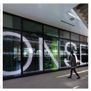
ON-SITE DIGITAL DISPLAYS ARE LARGE FORMAT LED DISPLAYS THAT CAN BE INSTALLED EITHER ON TOP OF OR BEHIND THE EXTERIOR WALL, BUT THEY MUST ALIGN WITH THE GLAZING MODULES. THE FINISH OF THE DISPLAY EDGES (IF VISIBLE) SHALL BE COORDINATED WITH THE EXTERIOR GLAZING SYSTEMS. ALL WIRING MUST BE DESIGNED TO BE HIDDEN FROM VIEW. LATEST HIGH QUALITY LED TECHNOLOGIES SHALL BE USED, AND BRIGHTNESS WILL BE CONTROLLED PER DARKSKY GUIDELINES.
