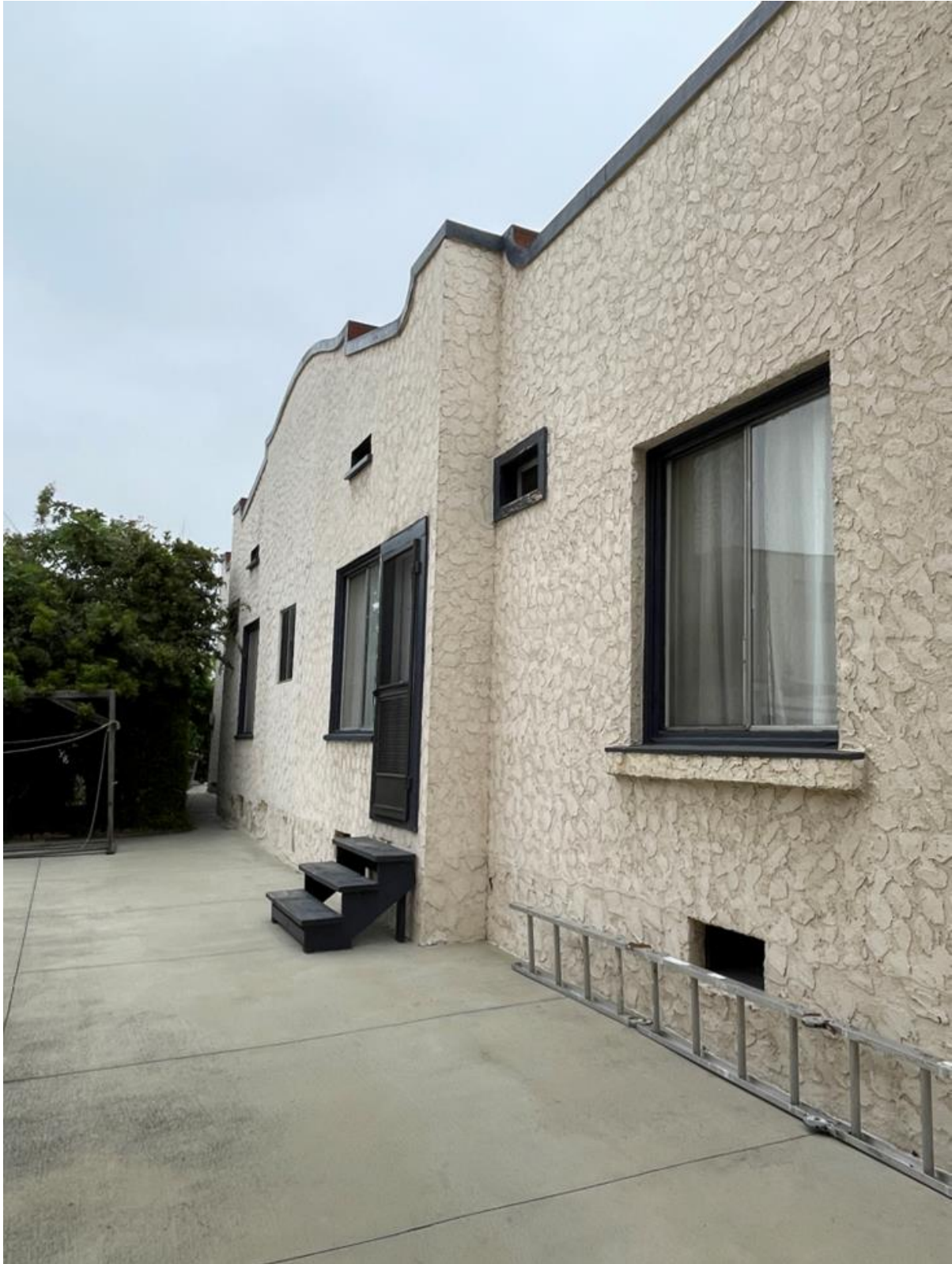
Figure 23. West elevation, southwest perspective
