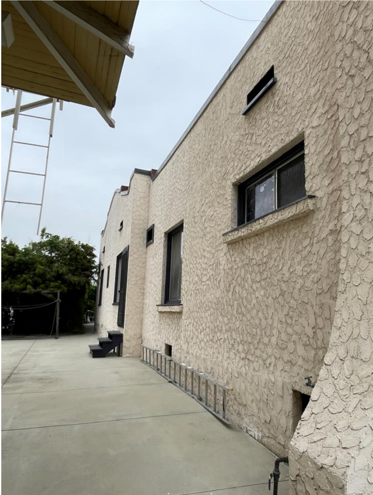
Figure 22. West elevation, southwest perspective
