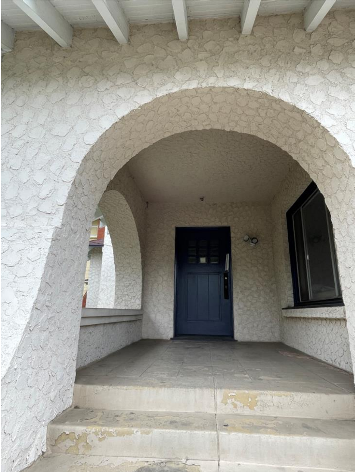
Figure 18. Detail of entry porch and front door, east perspective
