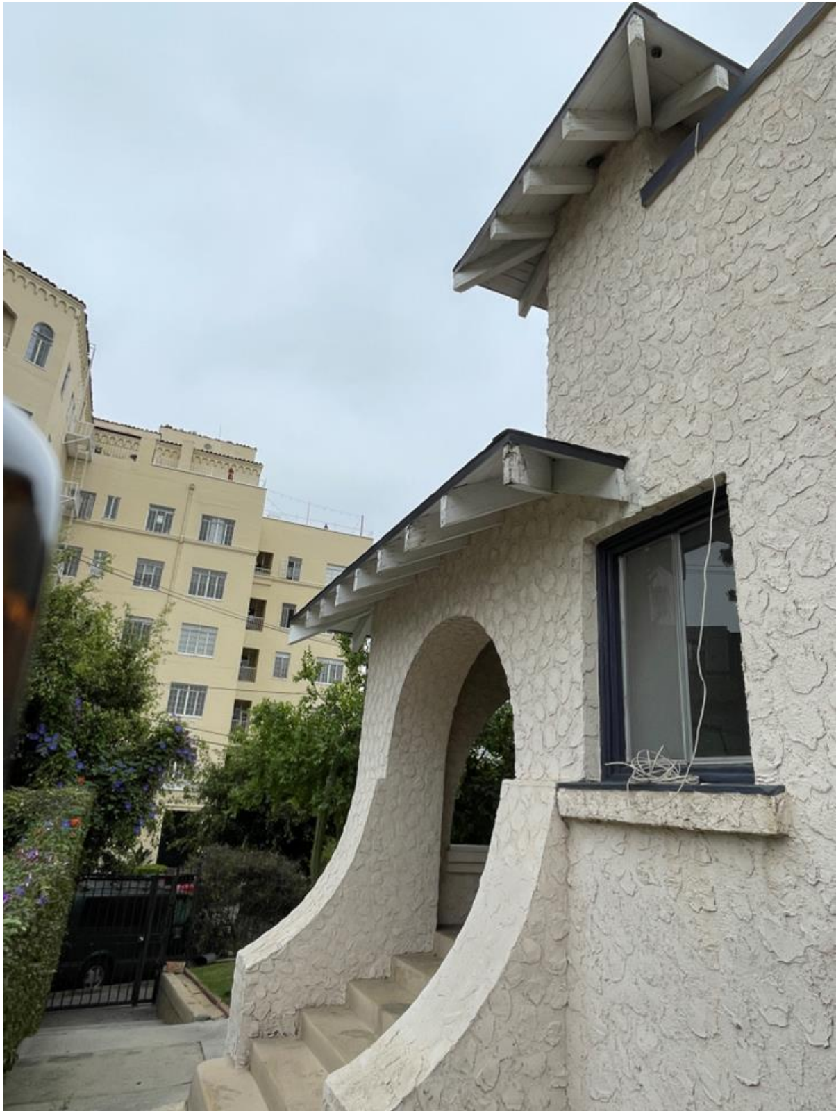
Figure 17. Façade entry porch and tower with hipped roof, northeast perspective
