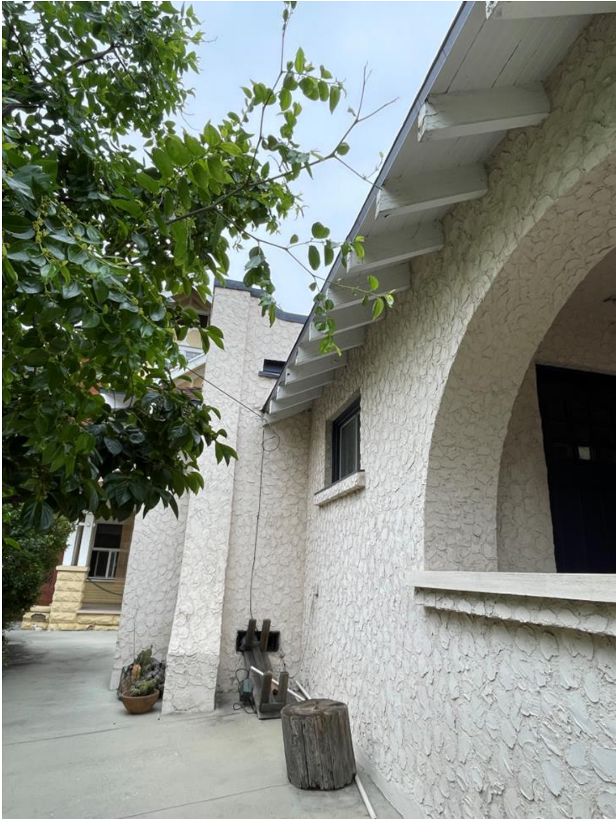
Figure 19. Main entrance and portion of façade, east perspective
