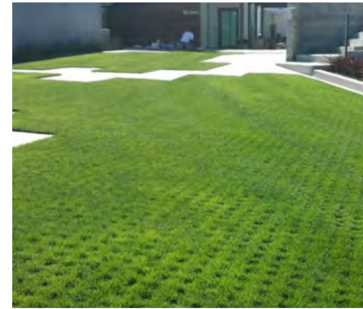
DRIVABLE GRASS BY SOIL RETENTION
