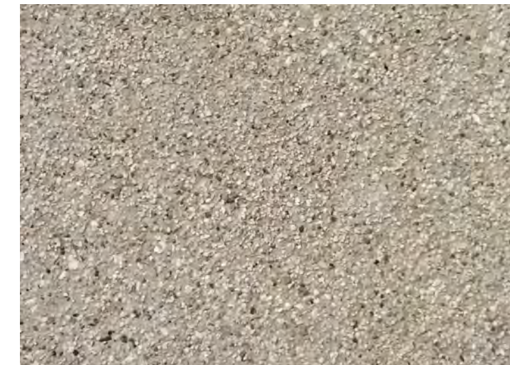
CIP CONCRETE PAVING TYPE 2 GREY CONCRETE W TOPCAST #3 FINISH LOOSE FURNITURE (BY OTHERS)
