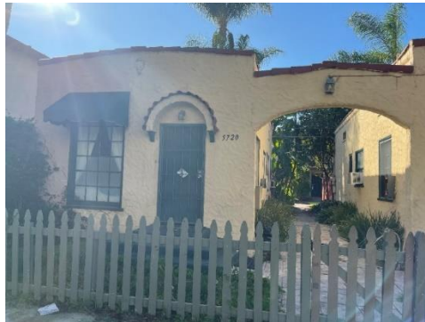
Primary/Northern Façade (5720 Waring Avenue, view south)
