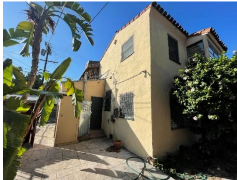
Eastern Façade, 5722 Waring Avenue (view southwest)
