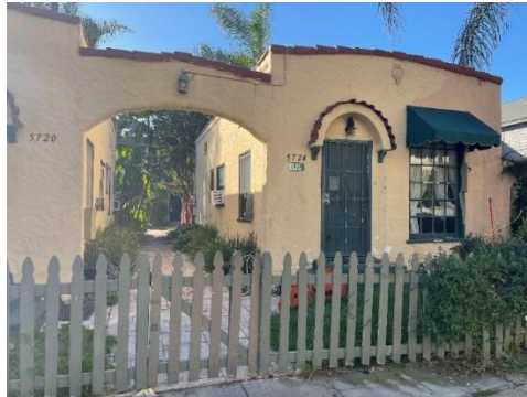
Primary/Northern Façade (5724 Waring Avenue, view southwest)
