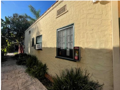
Eastern Façade, 5724 Waring Avenue (view southwest)
