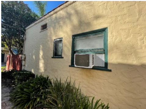
Eastern Façade, 5724 Waring Avenue (view southwest)
