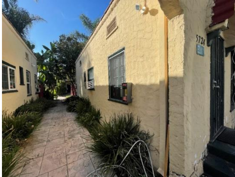
Eastern Façade, 5724 Waring Avenue (view southwest)
