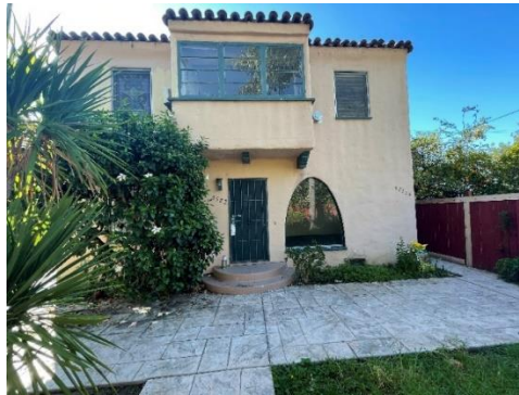
Primary/Northern Façade, 5722 Waring Avenue (view south)
