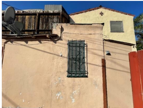
Eastern Façade, 5722 Waring Avenue (view west)
