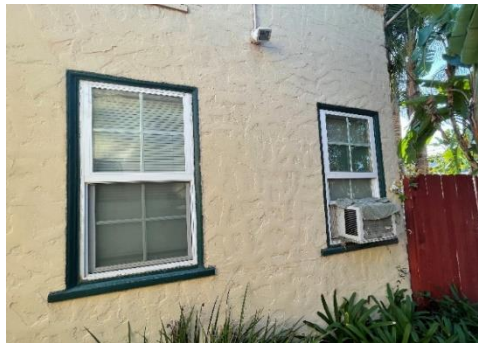
Western Façade, 5720 Waring Avenue (view southeast)
