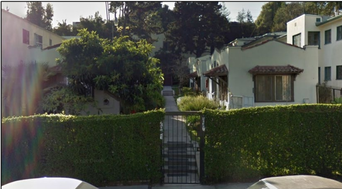
Figure 11. Street view of 2001-2007 Argyle Avenue (Google Earth).
