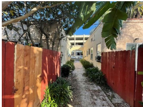
Southern Façade (5720 and 5724 Waring Avenue, view north)
