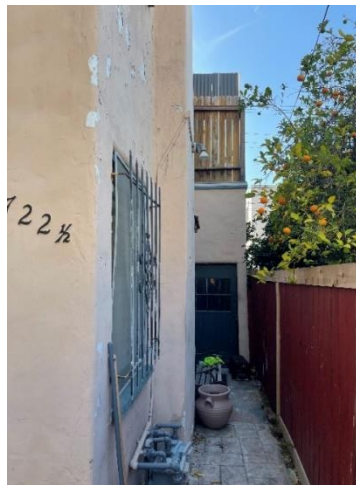
Western Façade, 5722 Waring Avenue (view south)
