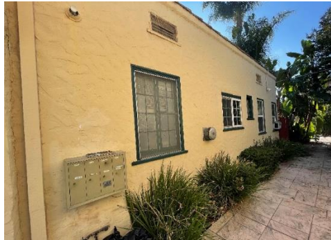
Western Façade, 5720 Waring Avenue (view southeast)
