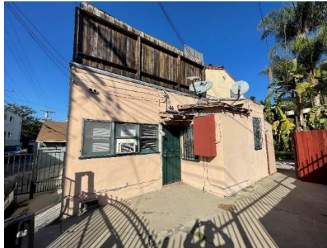
Eastern Façade, 5722 Waring Avenue (view northwest)
