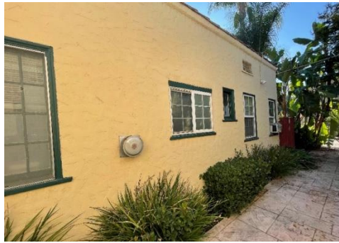
Western Façade, 5720 Waring Avenue (view southeast)
