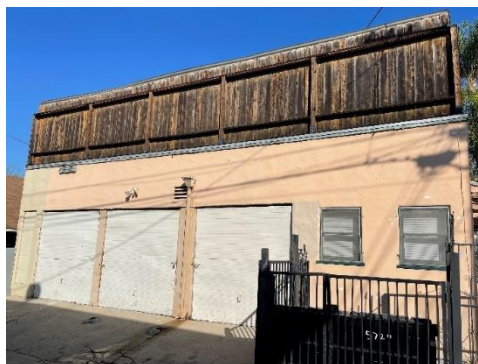
Southern Façade, 5722 Waring Avenue (view north)
