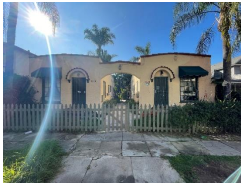
Primary/Northern Façade (view south)
