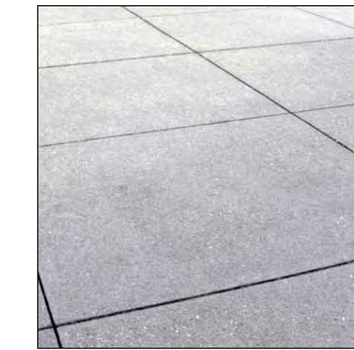
POURED IN PLACE CONCRETE PAVING
