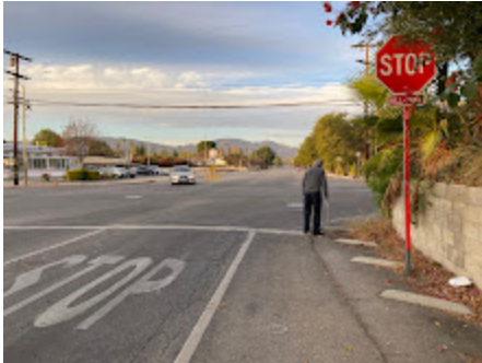
traffic bumps to keep cars from running into property wall at on Woodlake.jpg 1148K
