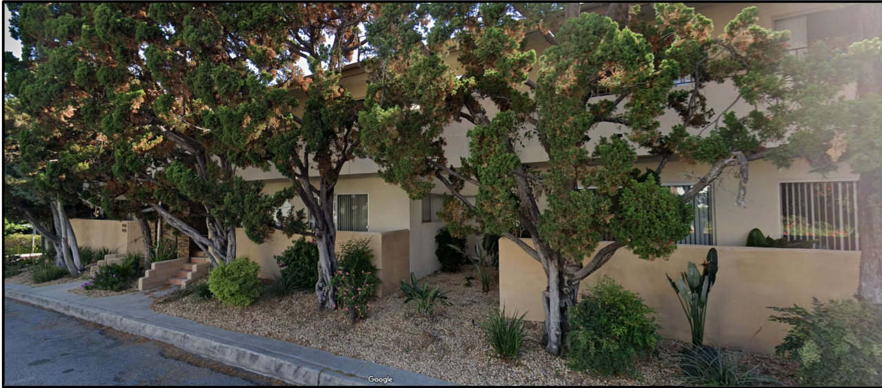
Photo 3 – View of property across Cartwright Avenue looking easterly.
