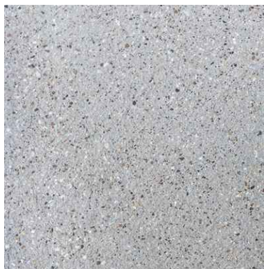
CONCRETE PAVING SANDBLAST FINISH
