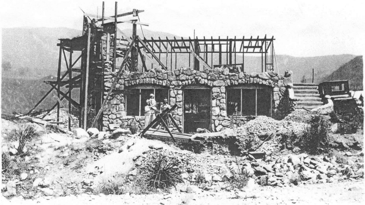
Elmer Reavis House under construction, 1923-24
