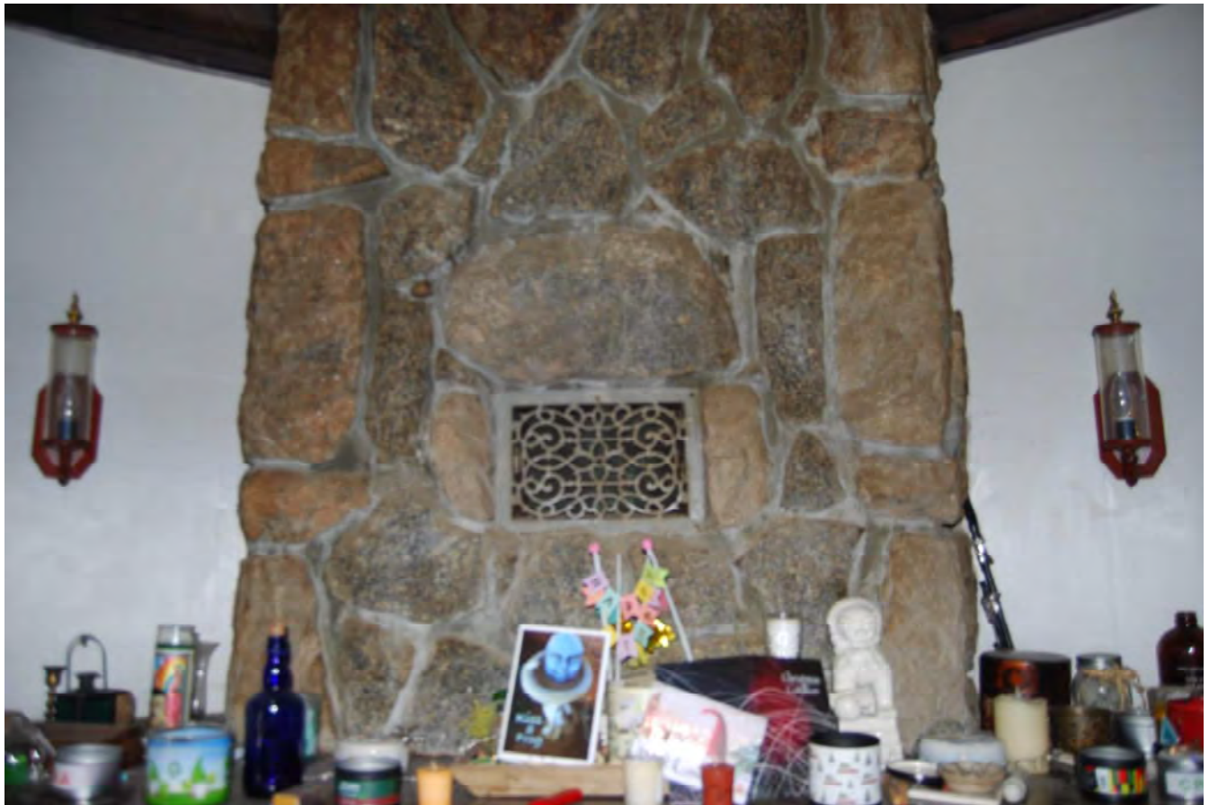
Elmer Reavis House, upstairs chimney, 10620 N Samoa Avenue, January 24, 2023, (Photograph by Charles J. Fisher)
