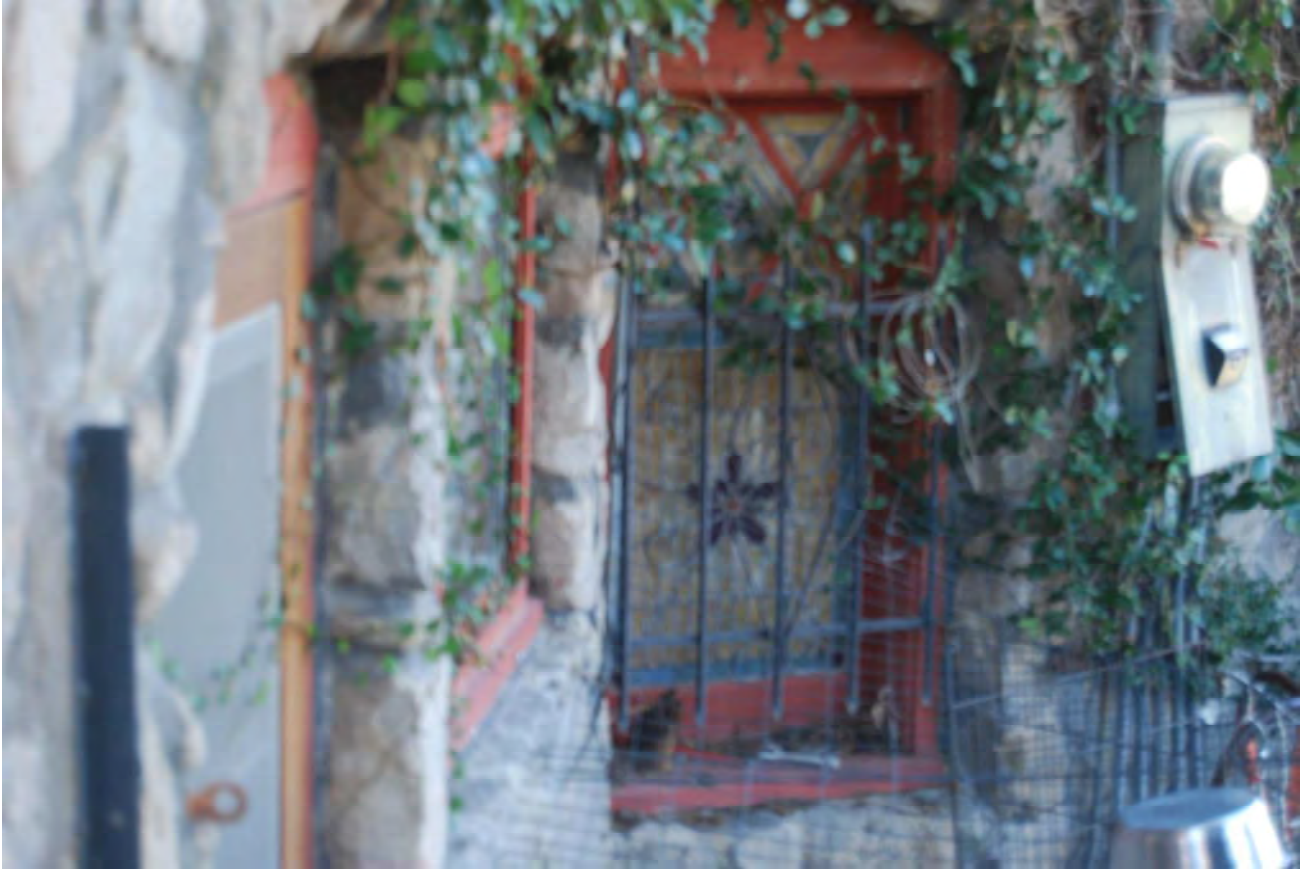
Elmer Reavis House, windows, 10620 N Samoa Avenue, January 24, 2023, (Photograph by Charles J. Fisher)
