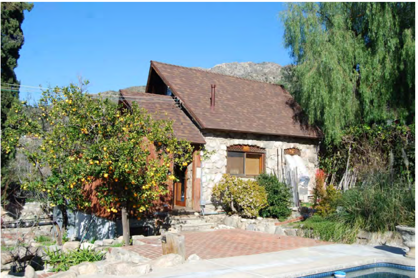
Elmer Reavis House, studio guest house, 10622 N Samoa Avenue, January 24, 2023, (Photograph by Charles J. Fisher)
