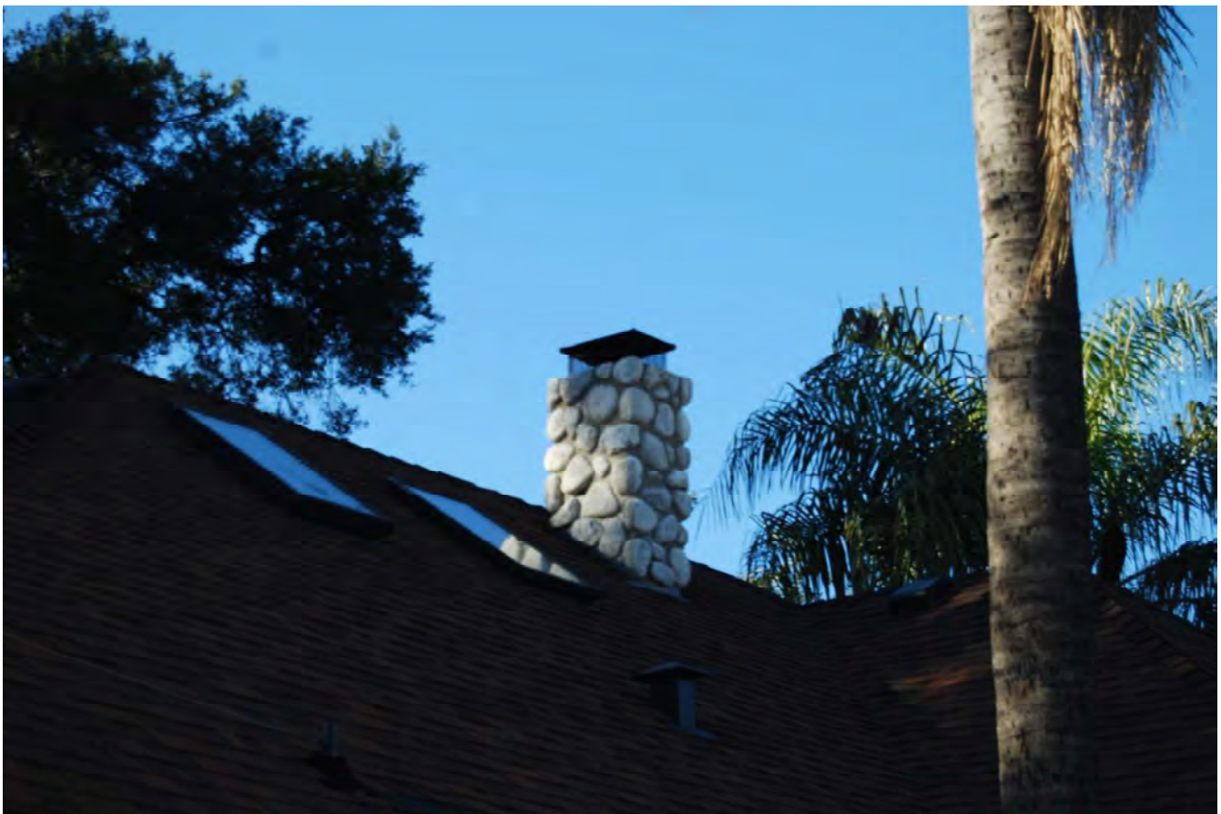
Rowley Residence, chimney, 8436 W Hillrose Street, January 24, 2023, (Photograph by Charles J. Fisher)
