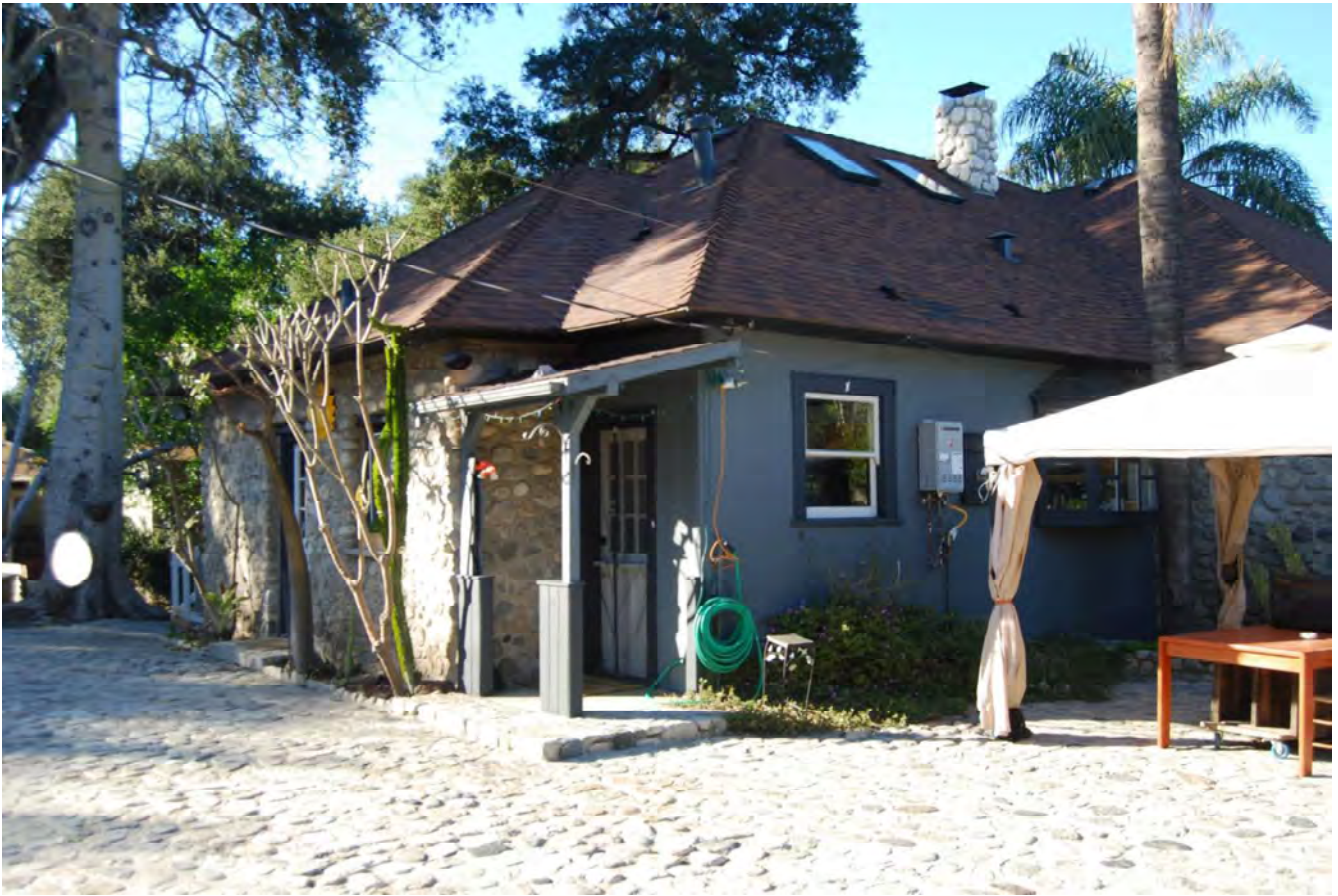
Rowley Residence, rear addition, 8436 W Hillrose Street, January 24, 2023, (Photograph by Charles J. Fisher)
